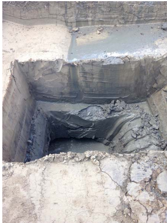
Plate 2: Trench 1, Section down to Gravel
