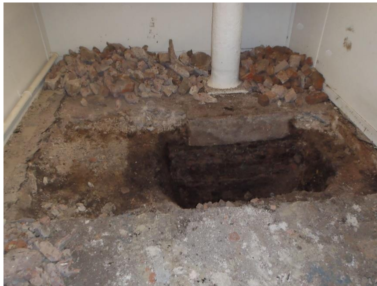
Figure 1: Test Pit 1, Looking North-West
