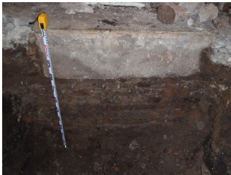
Figure 2: Footing [1] for Column
