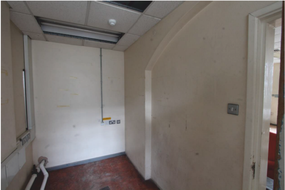
Plate 26 Room (G13) showing relieving arch
