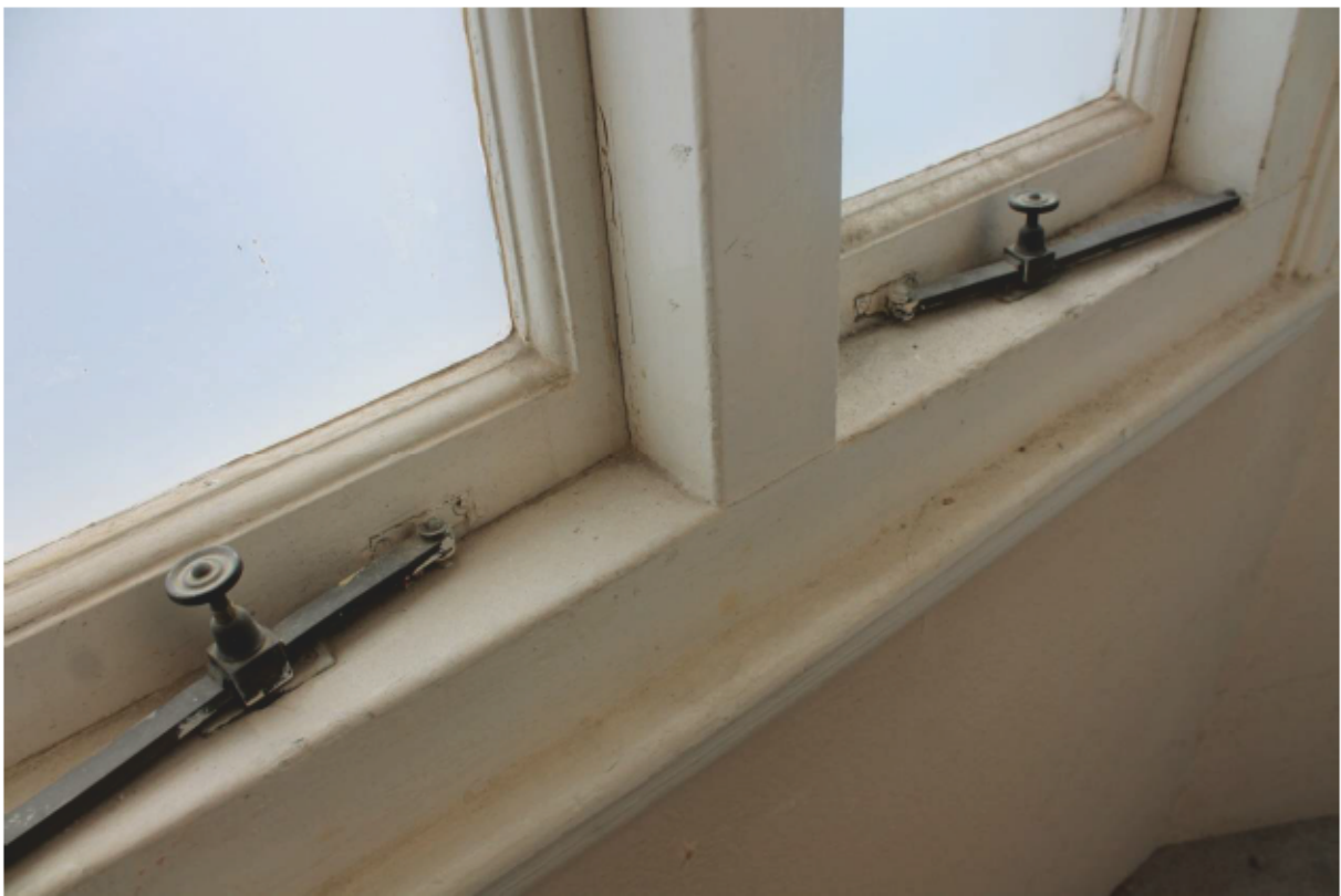
Plate 23 Window stays to bay window (G10)
