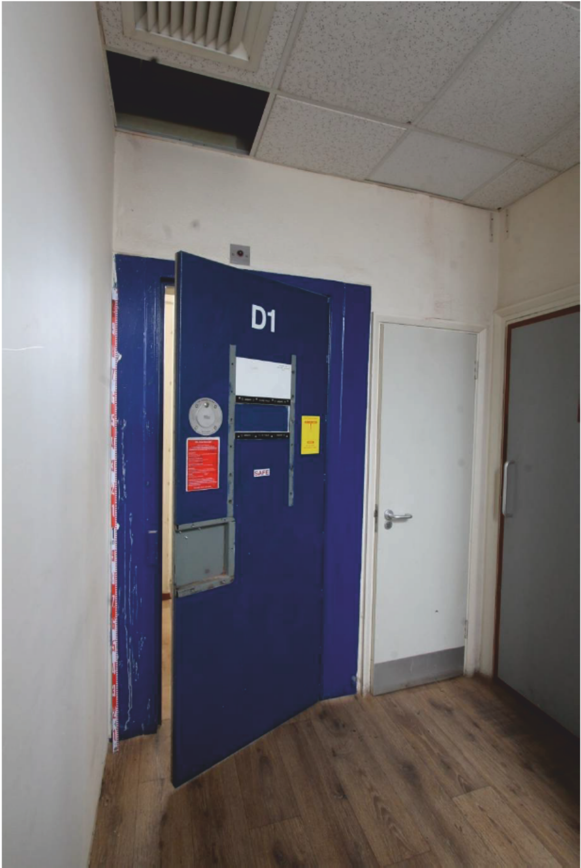
Plate 27 Cell Door (detention cell G16) and adjacent cistern cupboard
