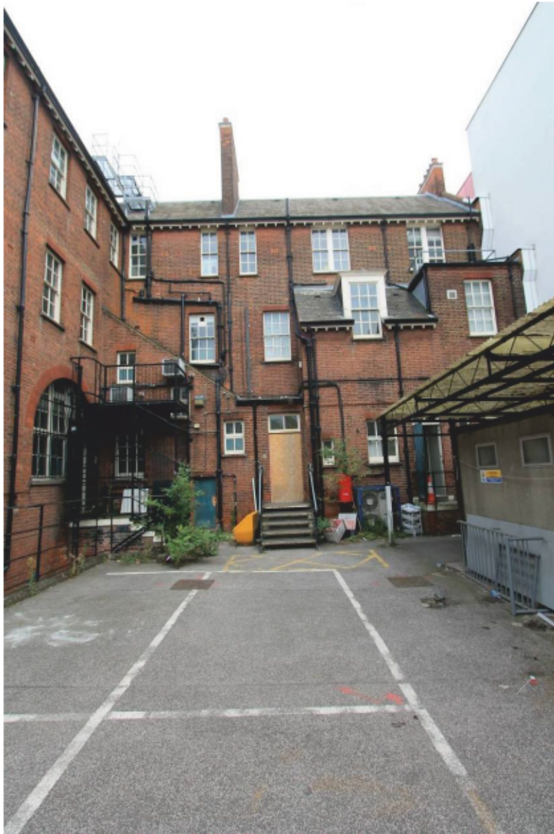
Plate 7 Rear elevations of Front Range looking north-east
