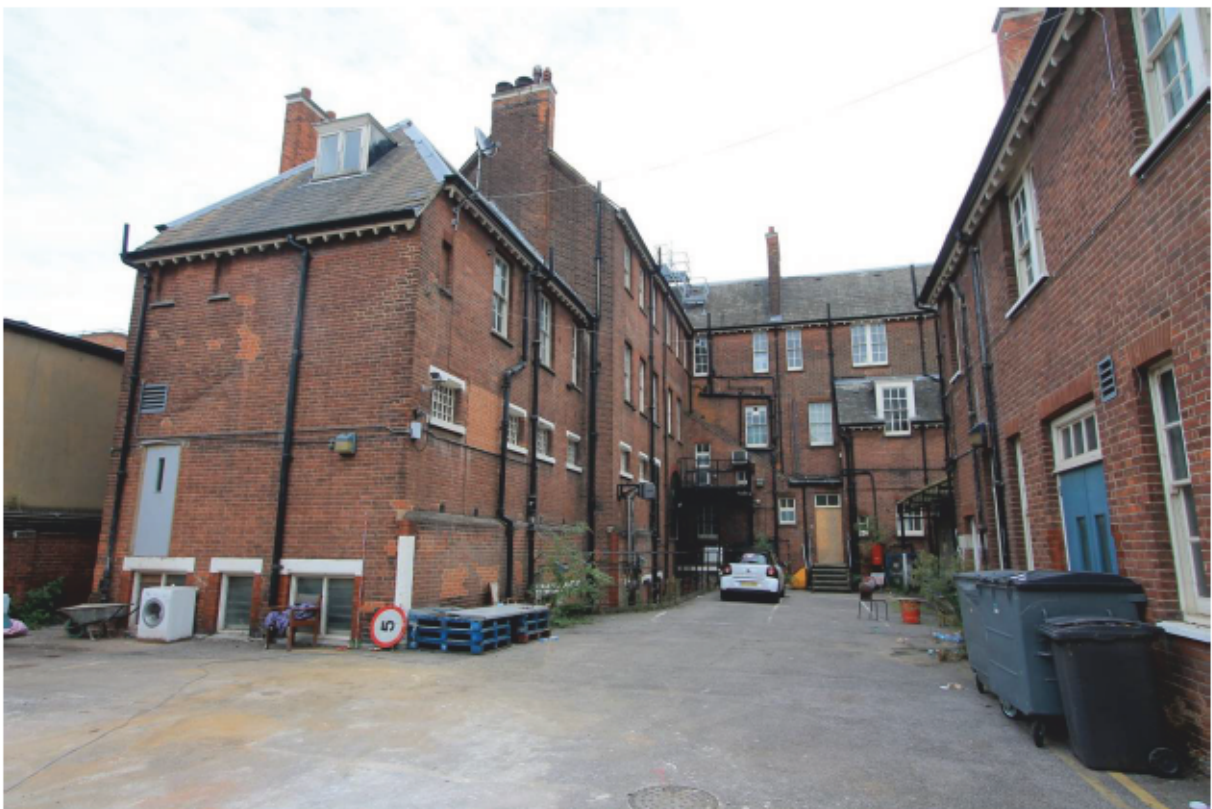
Plate 6 Rear Elevations of Police Station looking north-east
