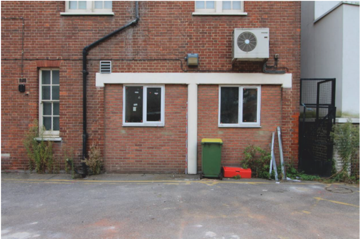
Plate 14 Blocked carriage opening
