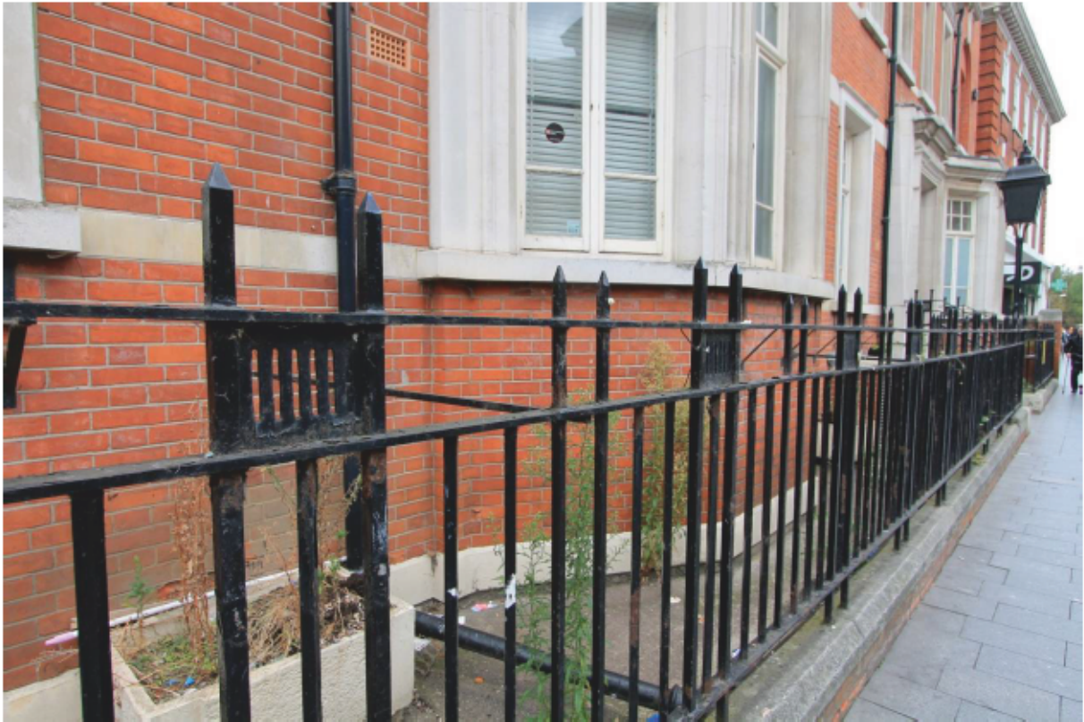
Plate 5 Railings to Ripple Road
