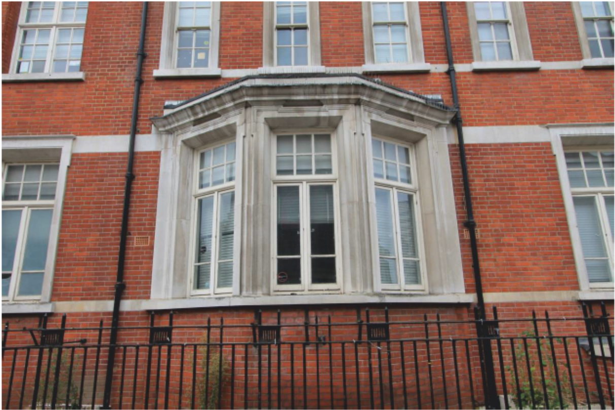
Plate 3 Detail of Portland Stone bay window and banding
