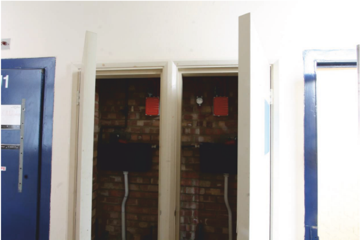
Plate 34 External cisterns to cell WCs
