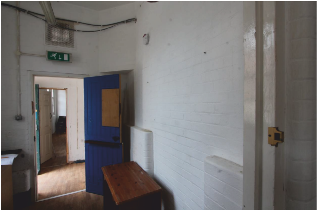
Plate 53 Present kitchen (SB2)
