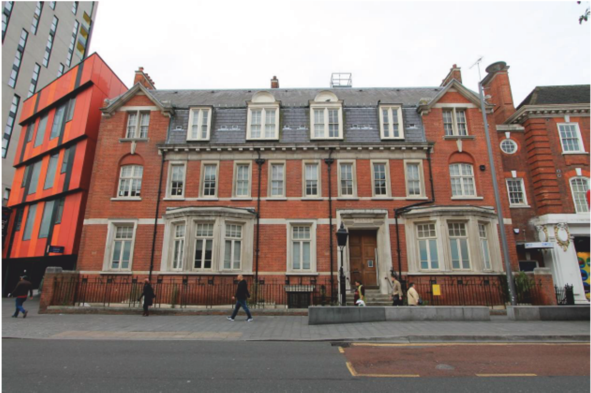
Plate 1 Principal Elevation to Ripple Road looking south-west
