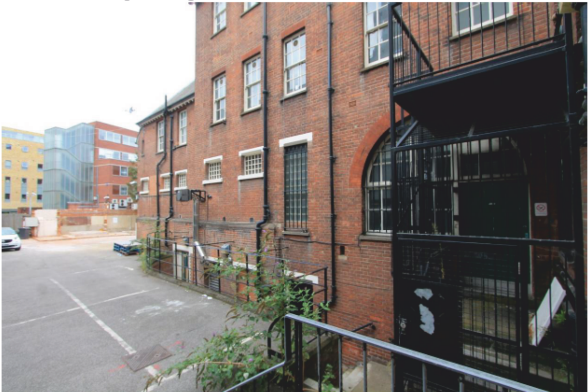
Plate 9 Return wing looking west
