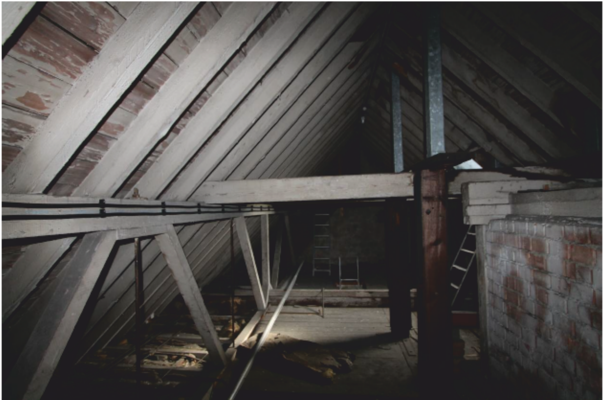
Plate 50 Roof structure over front range
