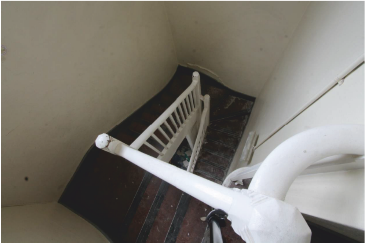
Plate 16 Elaborate open well stair (G23)
