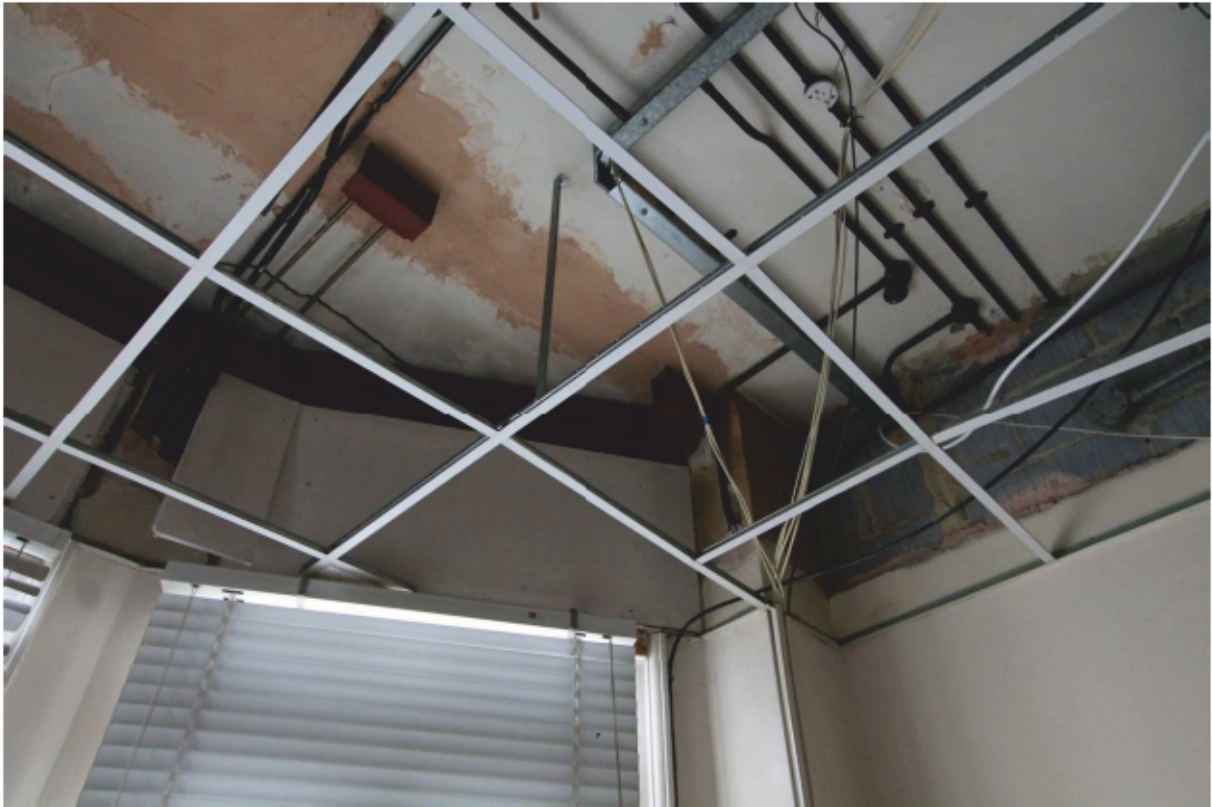
Plate 20 Structural steelwork to Bay Window (G6)
