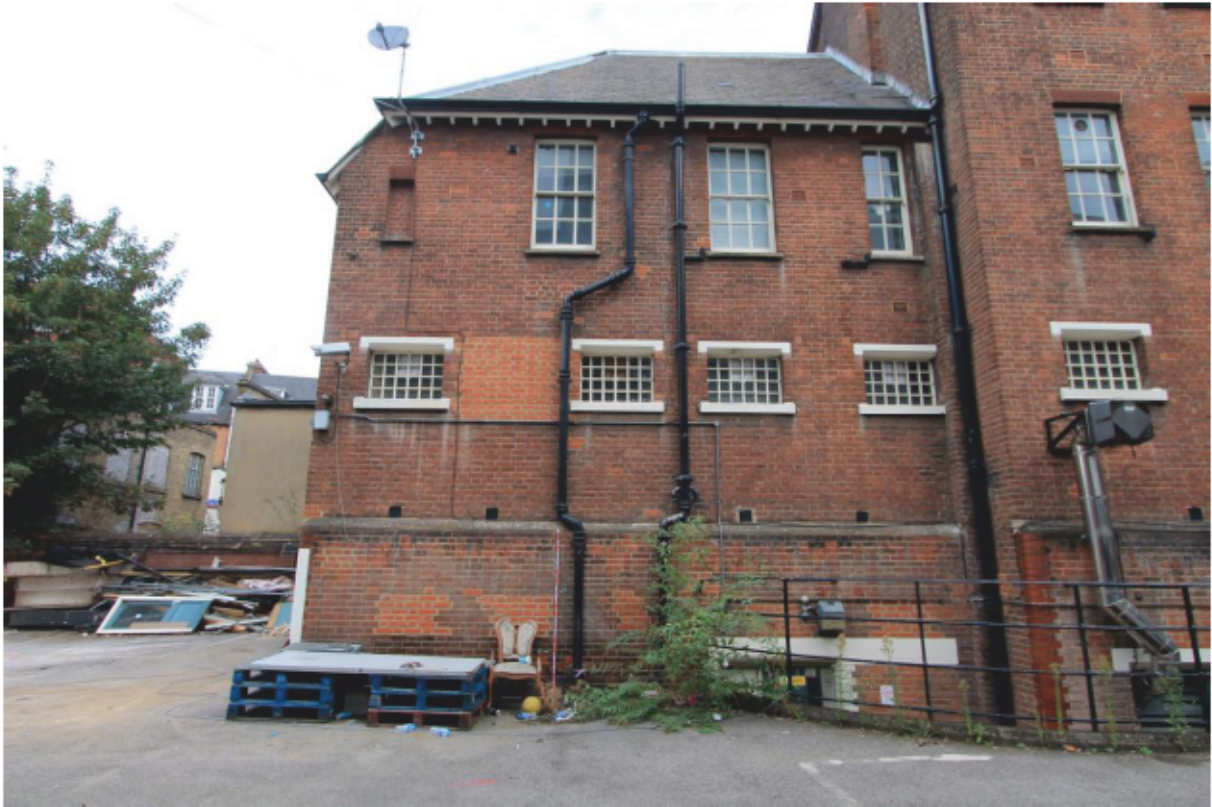
Plate 8 Return Range showing distinctive cell windows
