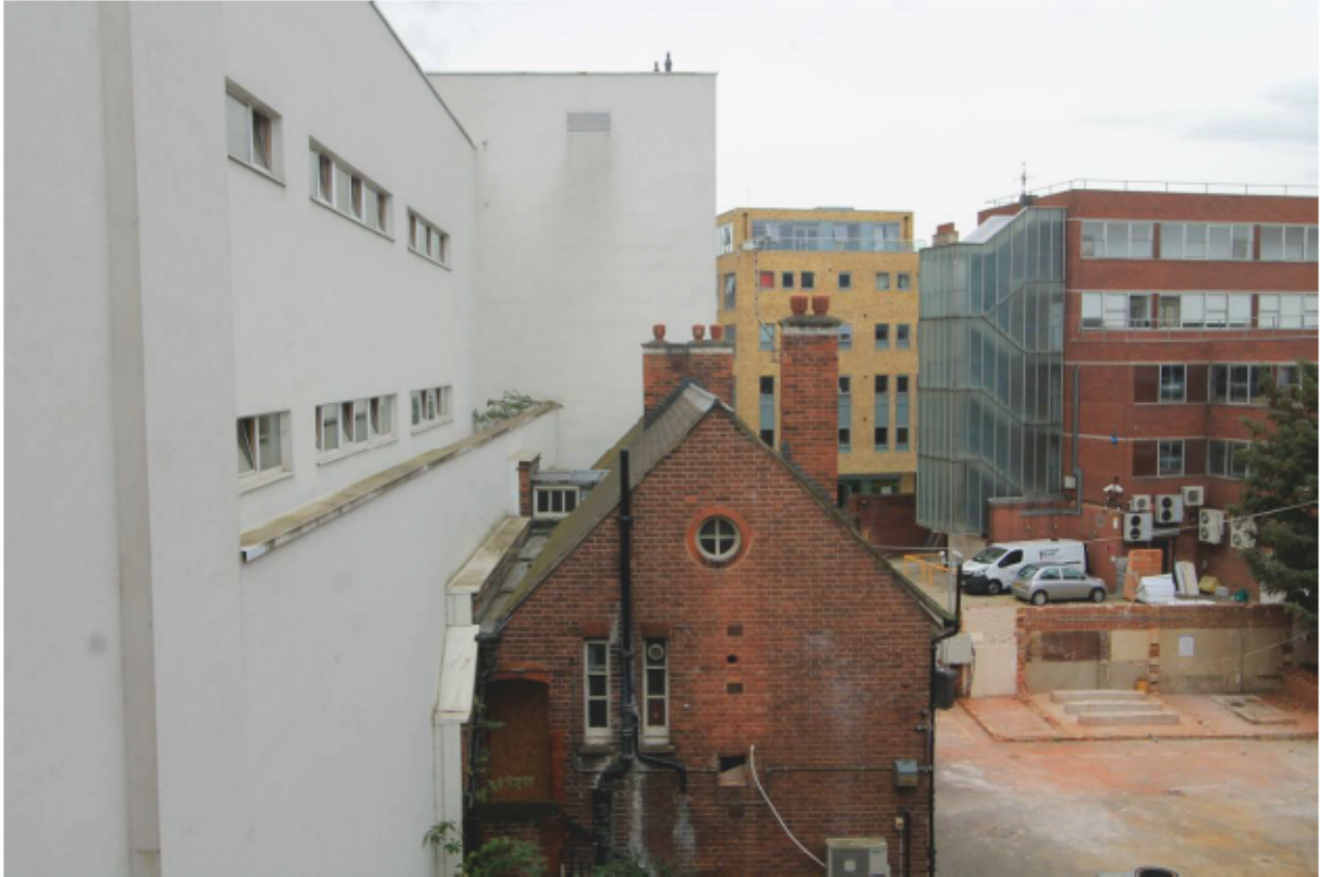
Plate 12 Stable Block gable elevation looking south-west
