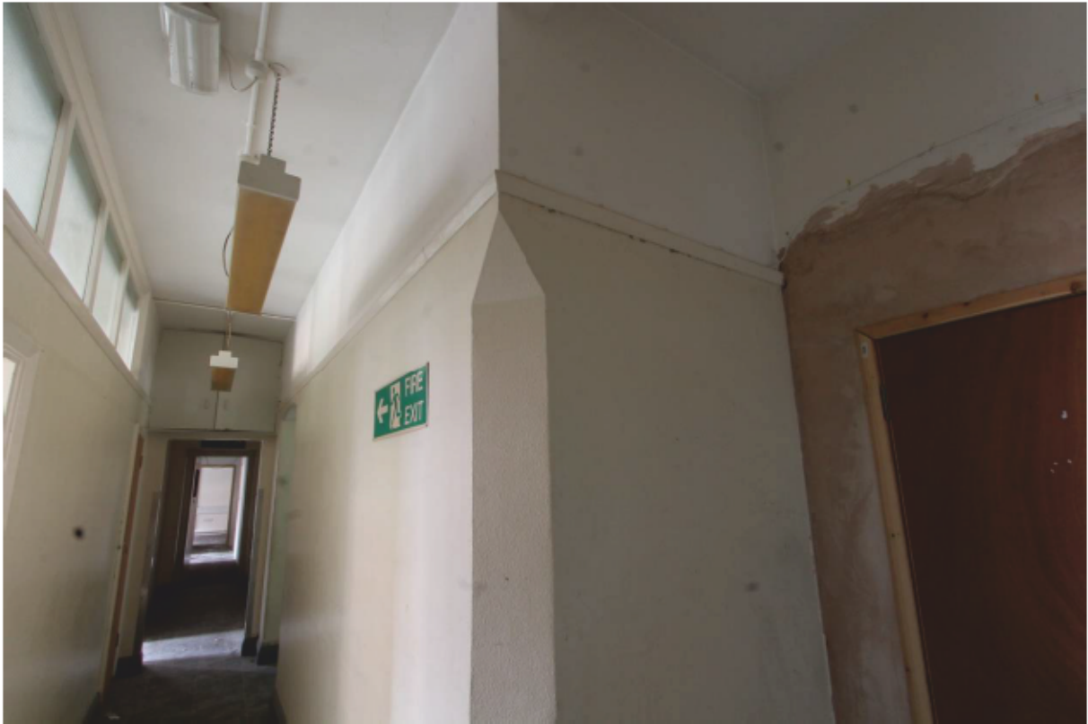
Plate 40 Chamfered and stopped corner (F22)
