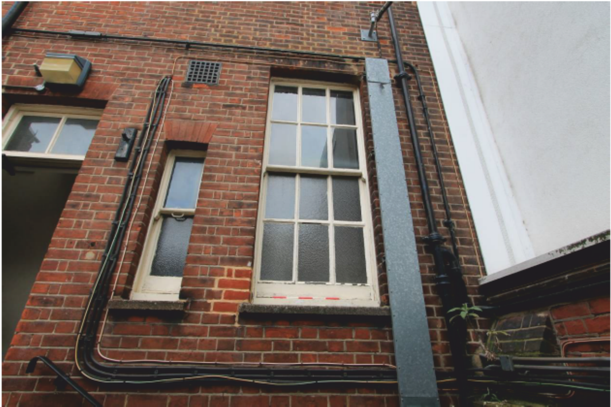
Plate 10 Typical sash window
