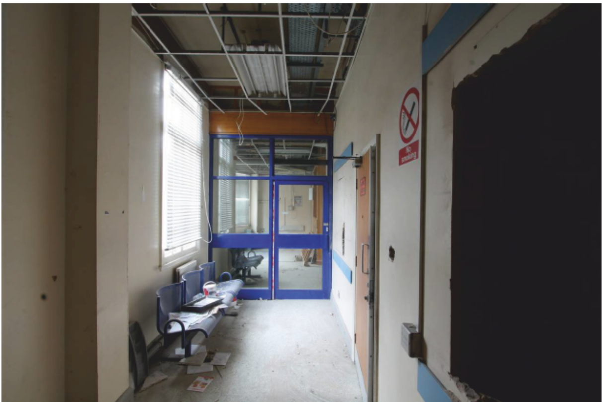
Plate 21 View to Reception from Entrance Foyer (G7)
