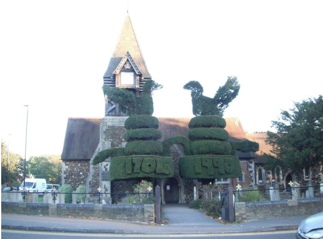
Plate 1: Looking north, St Mary's Church
