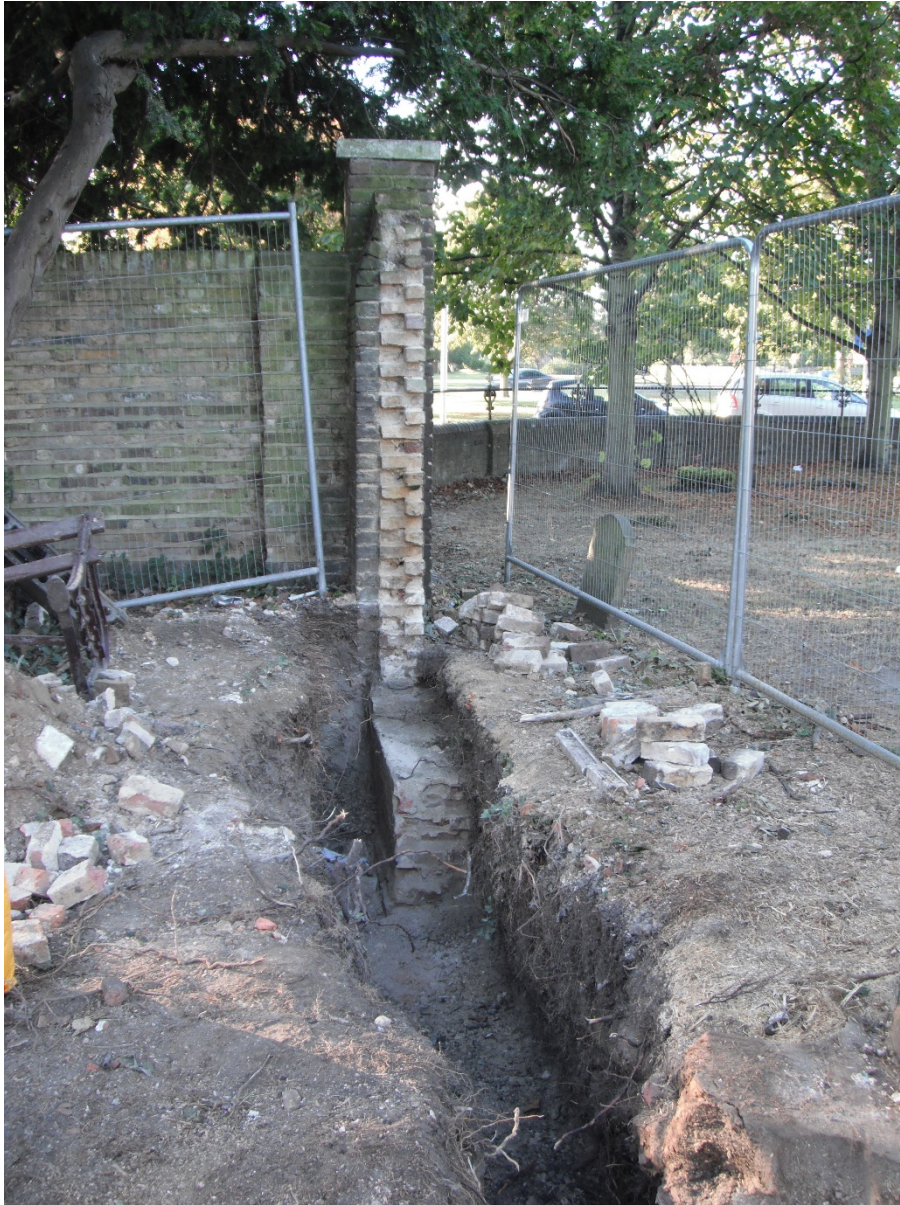
Plate 3: Looking south, north-south wall [7]
