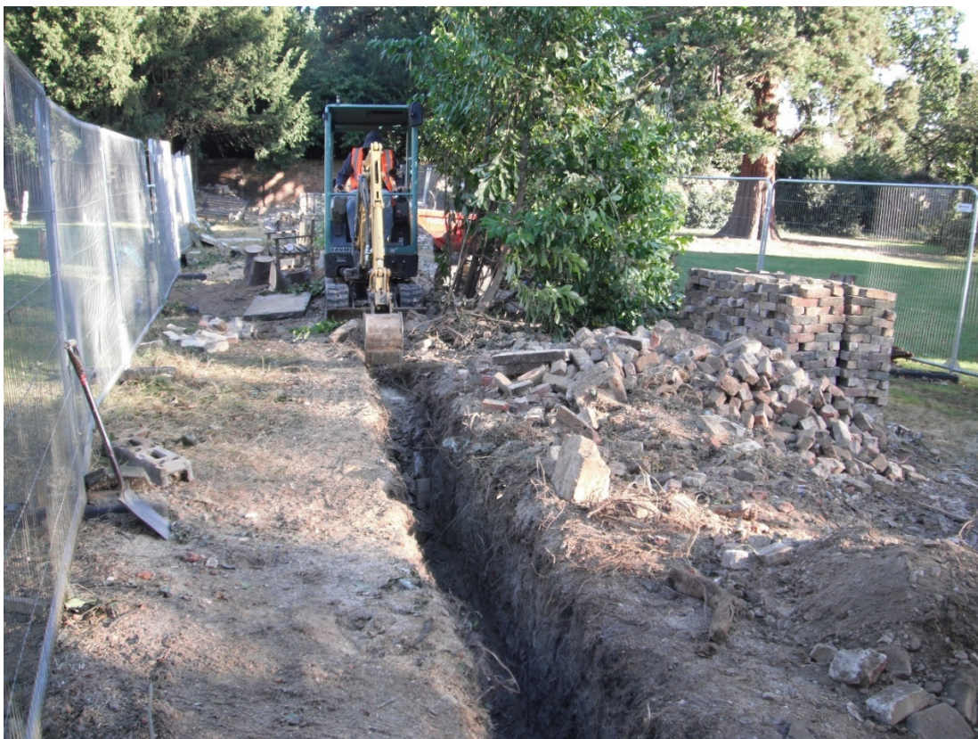
Plate 2: Looking north, mechanical excavator with flat bladed bucket
