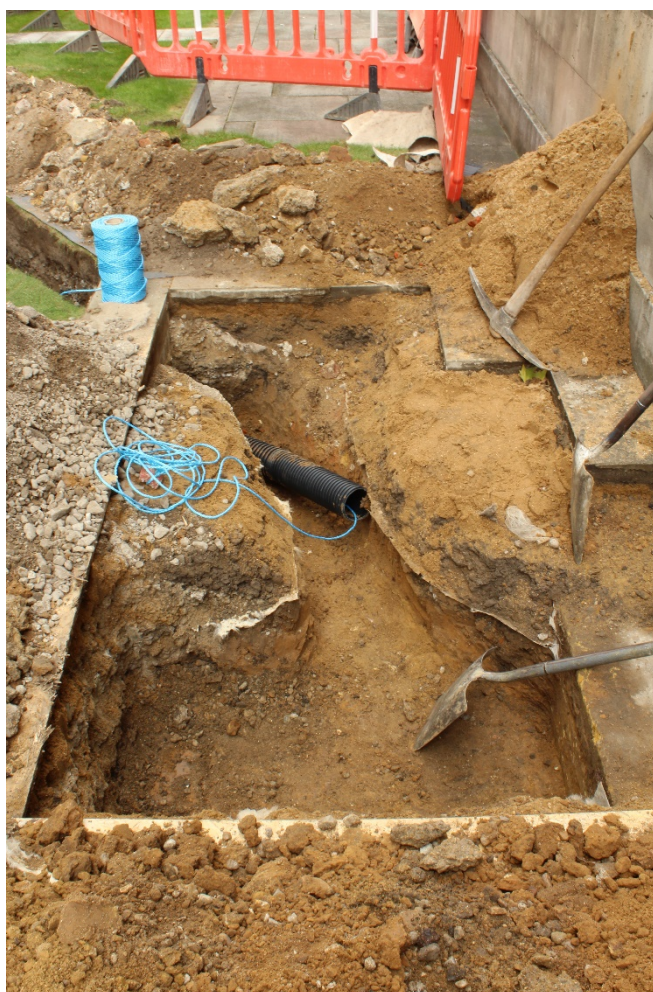
Plate 3: Access pit at south-eastern end, looking north
