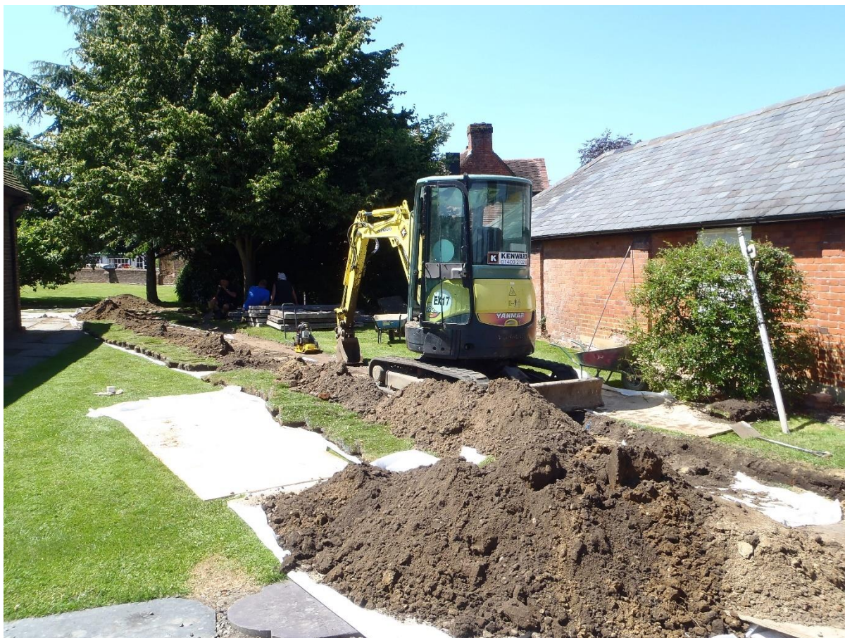
Plate 4 View to the east of the northern area of site (Figure 2)
