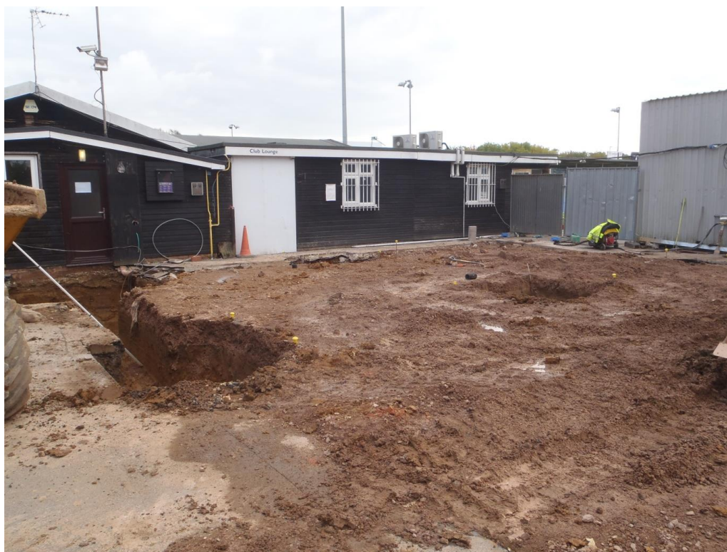
Plate 3 View to South East foundation pits
