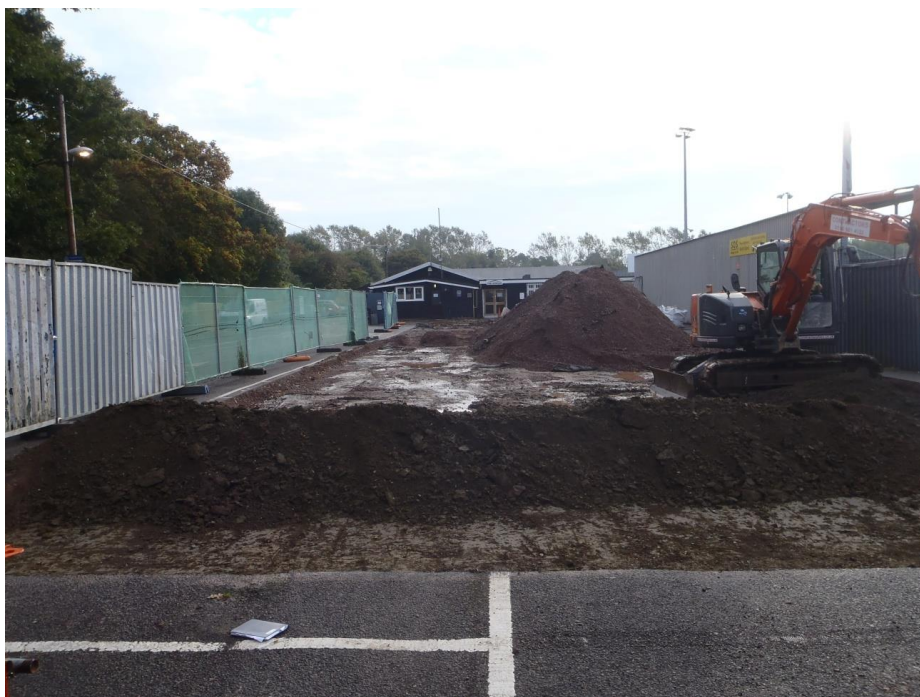
Plate 1 View to East of site
