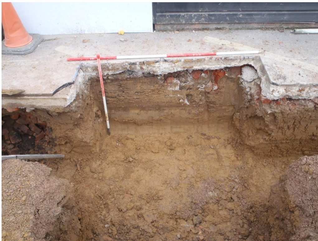
Plate 5 View to East foundation pit showing modern brickwork
