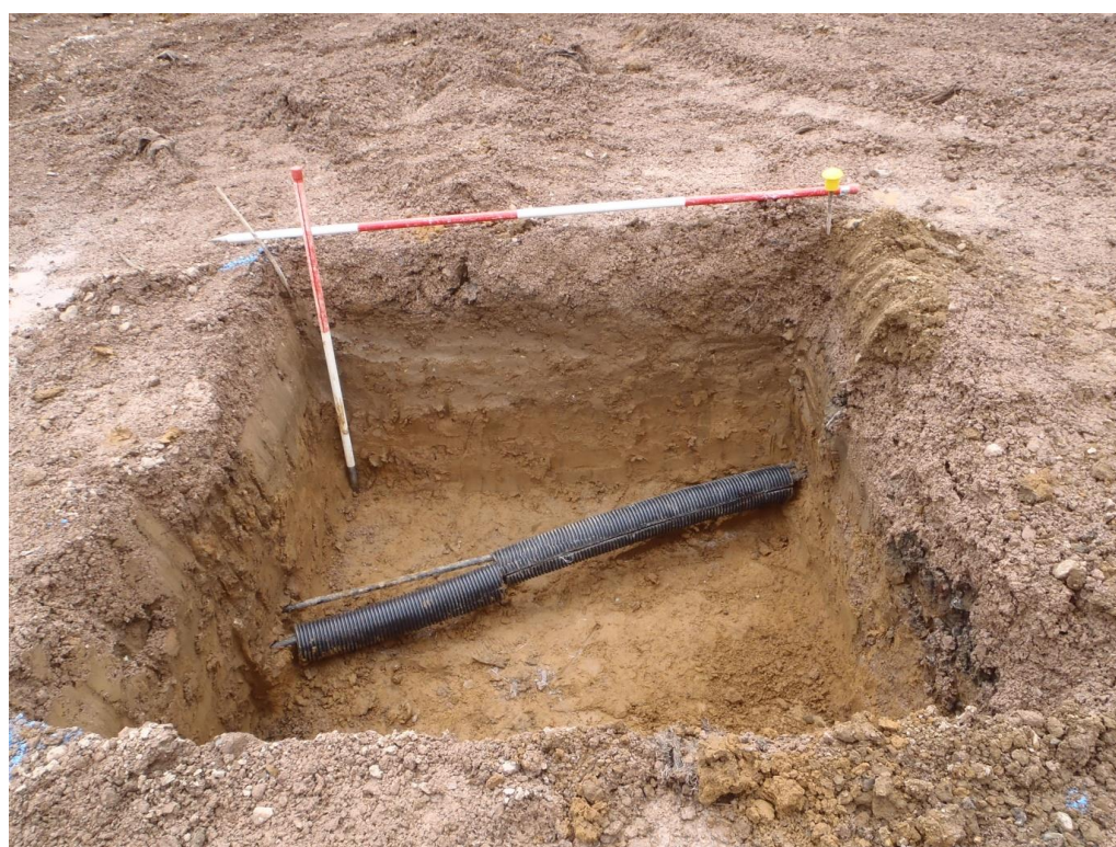
Plate 4 View to West foundation pit showing modern services
