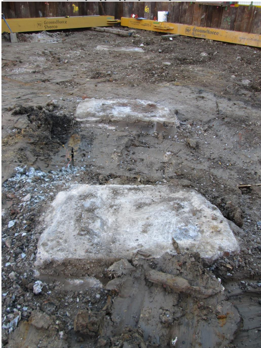
Plate 5 : Concrete piles [152],[153],[154]. Viewing North.
