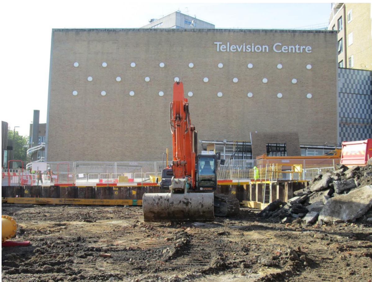
Plate 1 : Ground reduction, viewing NW.
