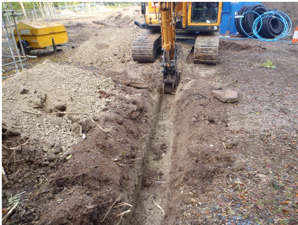
Plate 3 View to South East of excavation of service trench
