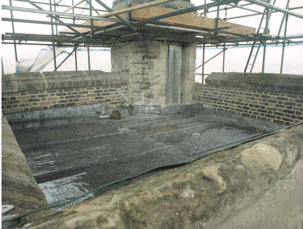
FIGURE 5: View of the roof post-conservation
