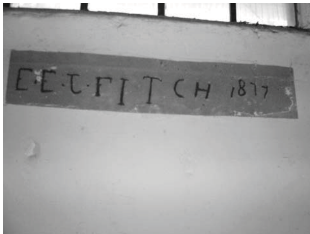
FIGURE 6: View of 'E.E.J. FITCH 1877' graffiti below the west Y tracery window
