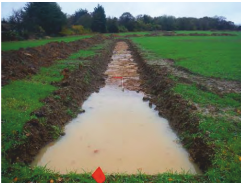
Plate 19: Trench 33 view west
