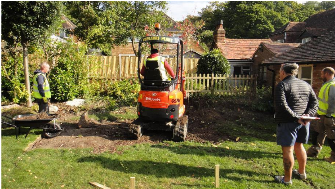
Plate 1. Initial machine stripping of topsoil, looking northeast.
