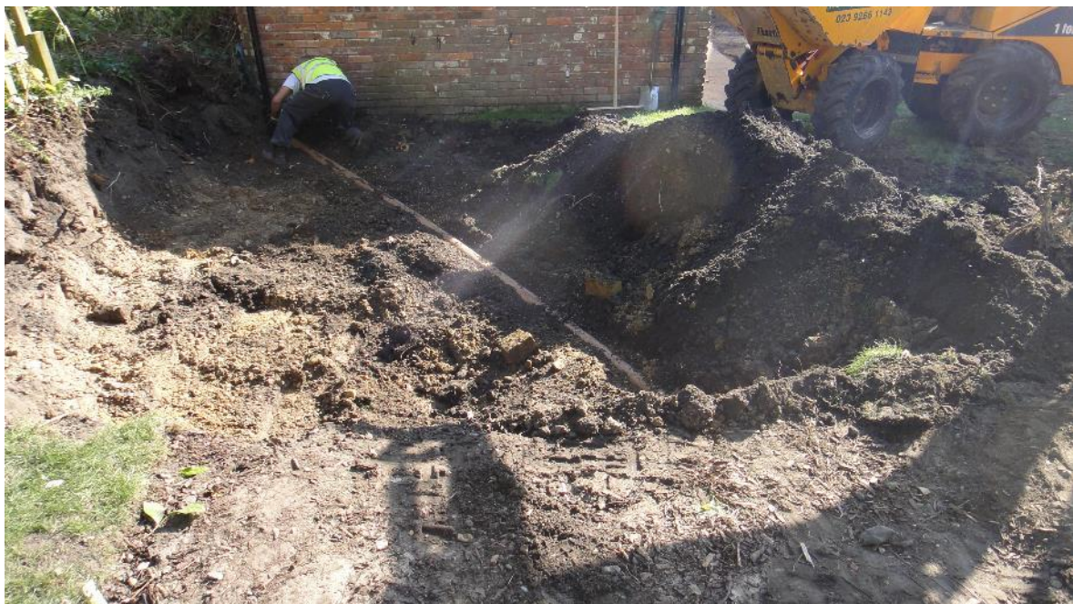
Plate 2. Working shot showing Modern soakaway pipe.
