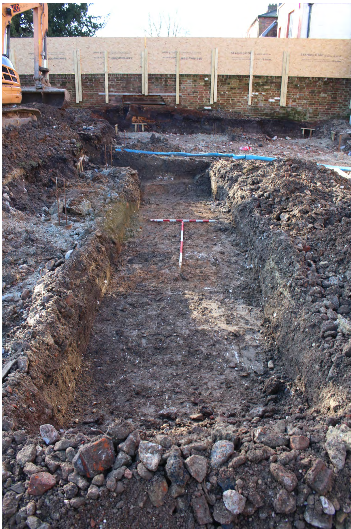
Plate 4 View to the south of evaluation trench, showing extensive modern disturbance in foreground
