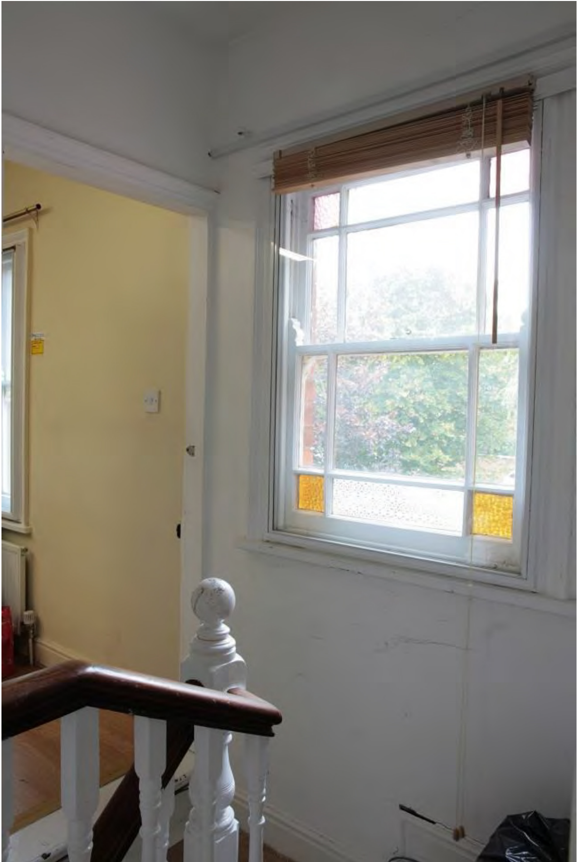
Plate 64: Sash window at First Floor Landing, looking east (LMSC16 D100 (73))
