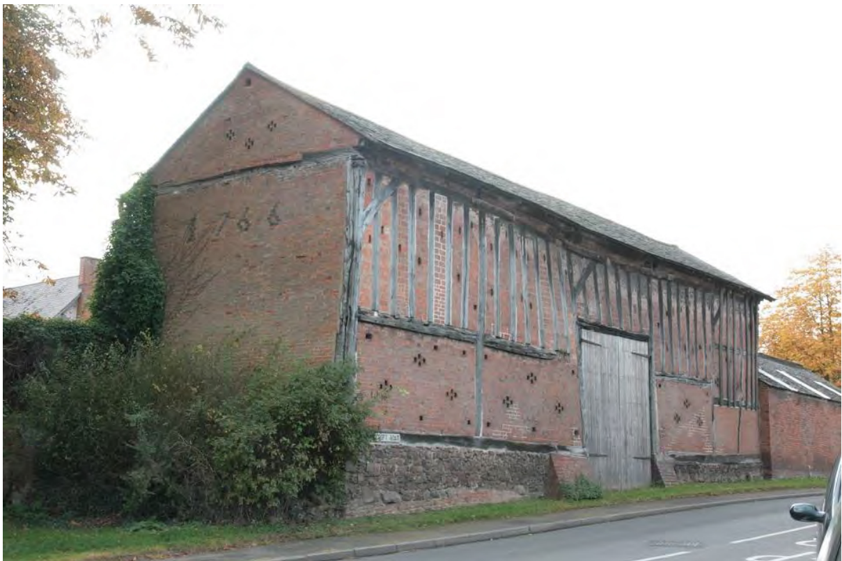
Plate 100: Late C16 Grade II Listed Barn, altered 1766, late C18, C19 and C20 on south side of Croft Road, Cosby with stone rubble plinth, looking west (LMSC16 D100 (132))
