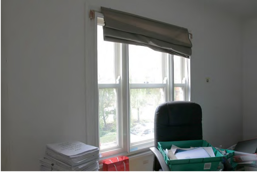
Plate 66: Sash window in the First Floor Store Room, looking south (LMSC16 D100 (78))
