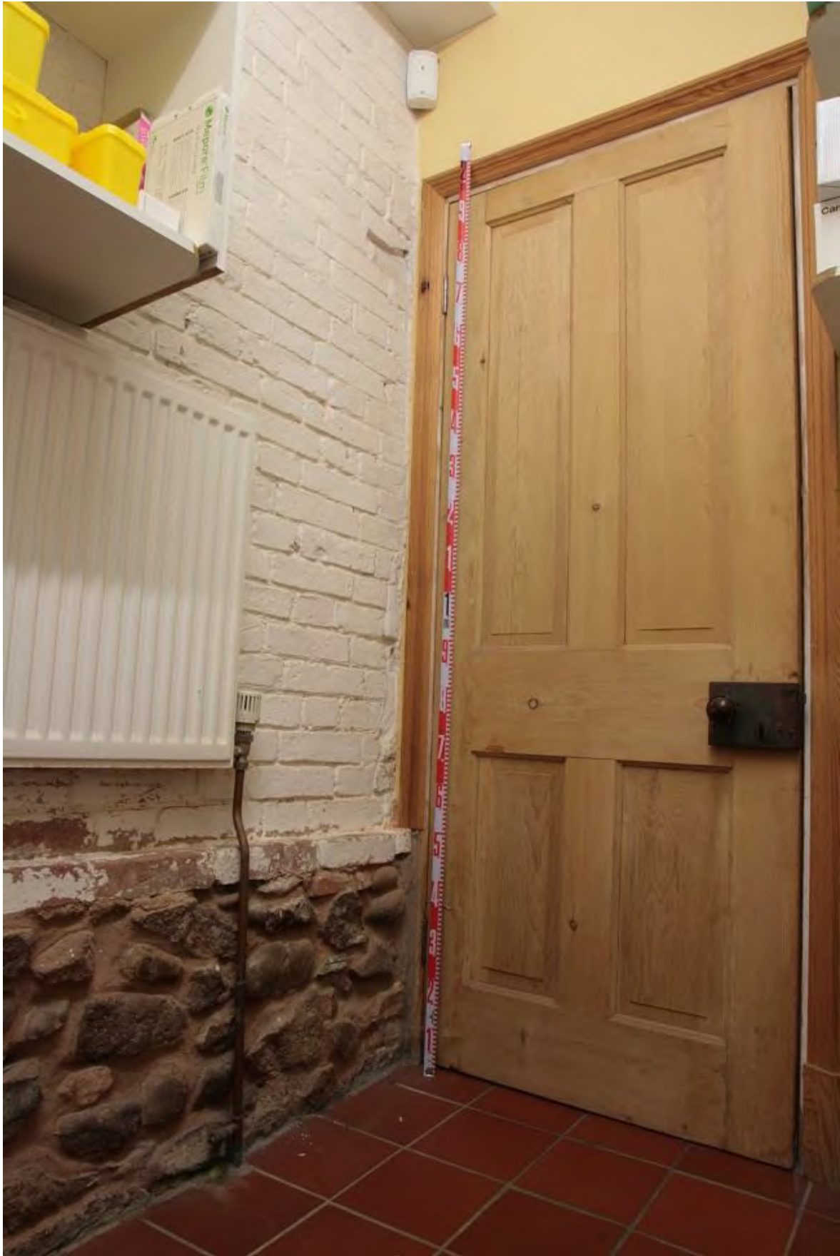
Plate 43: Detail showing original stone courses at base of Medstore's southeast wall, looking southwest (LMSC16 D100 (43))
