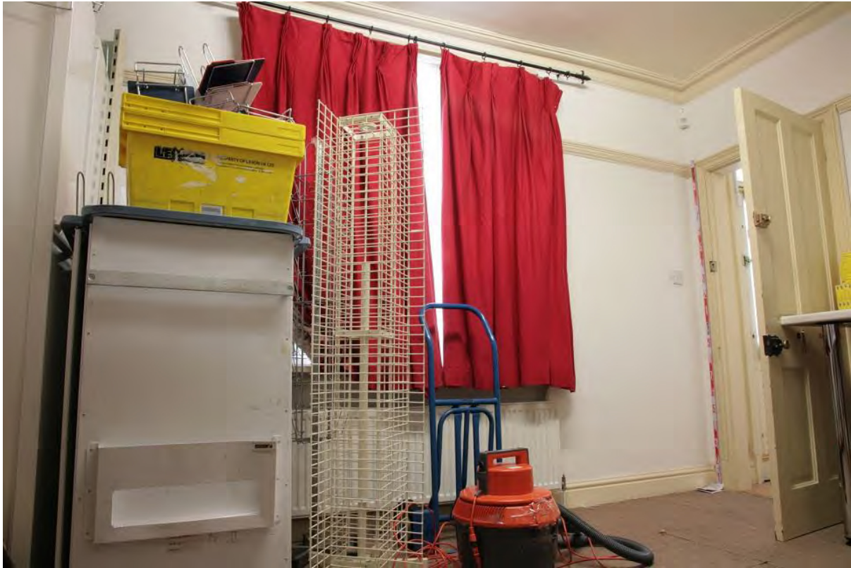
Plate 57: South-east wall of Staff/Store Area, looking south (LMSC16 D100 (67))
