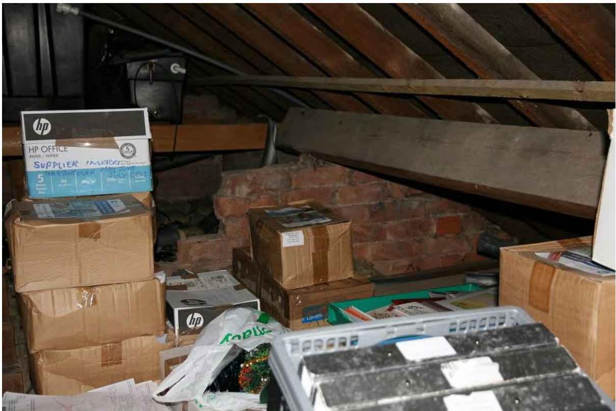
Plate 94: Attic space, looking east (LMSC16 D100 (99))
