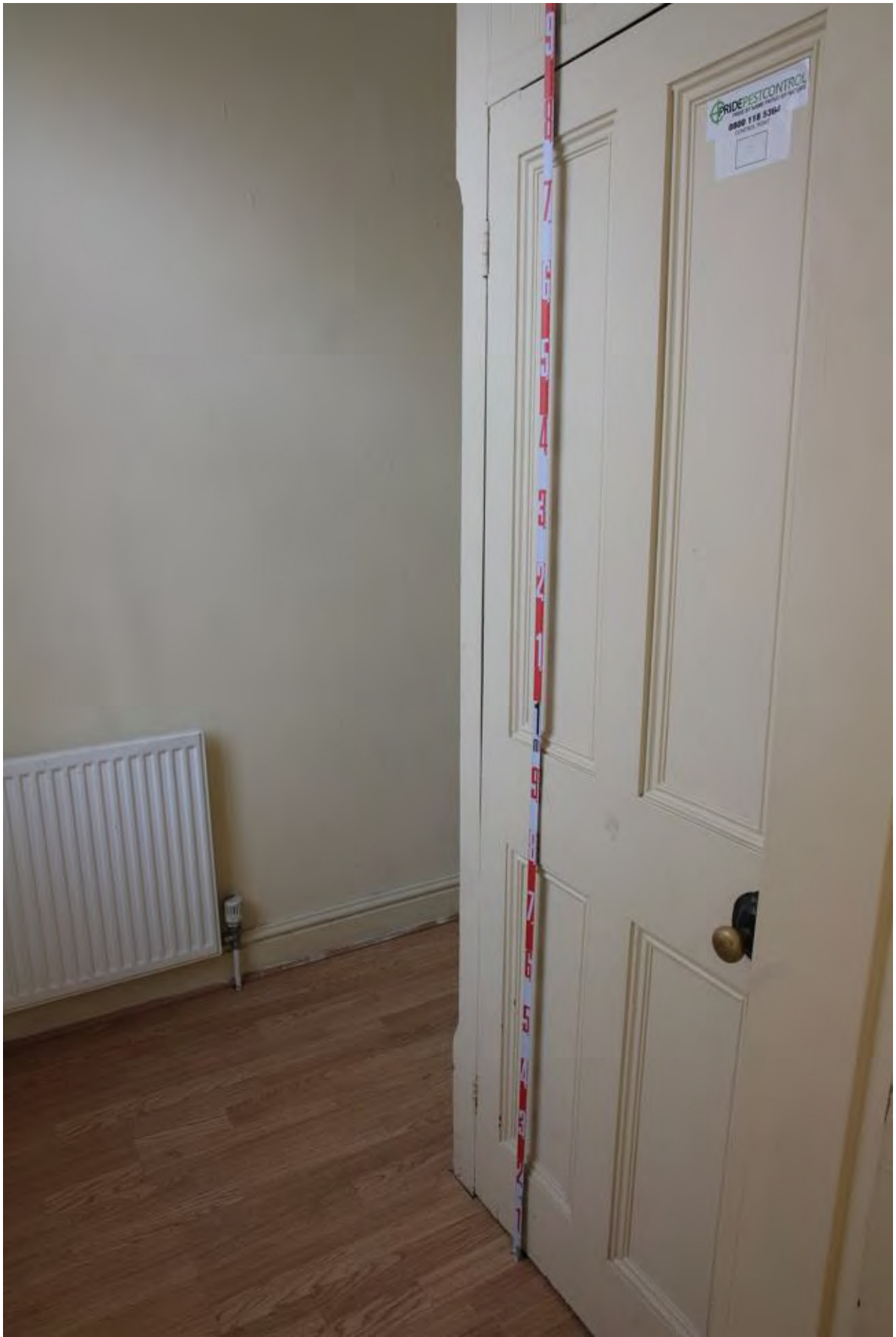
Plate 51: Under stairs cupboard in Entrance Lobby, looking west (LMSC16 D100 (58))
