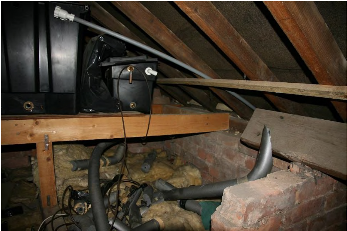
Plate 96: Attic space, looking east (LMSC16 D100 (103))
