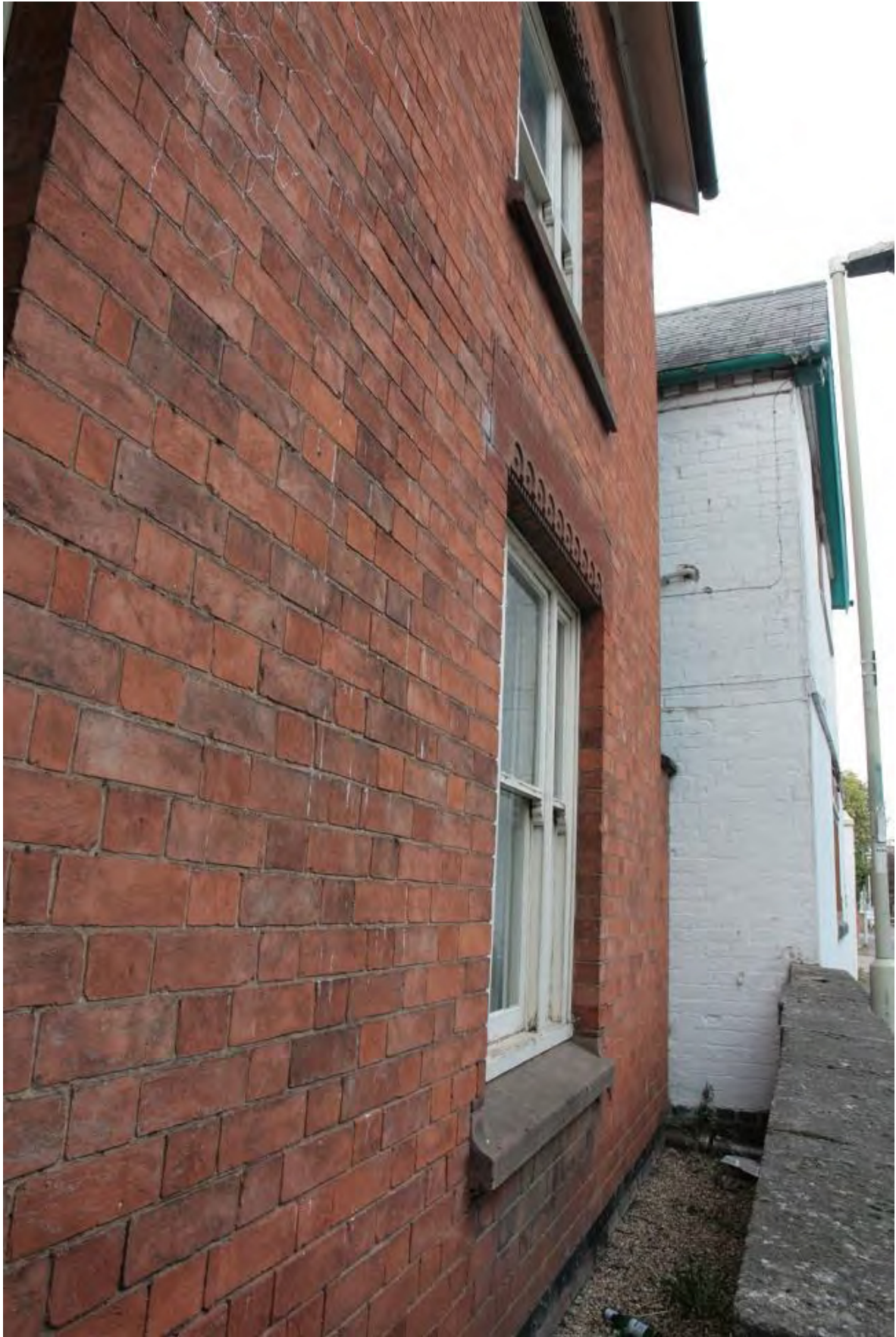
Plate 7: Oblique view showing front yard area, looking north-east (LMSC16 D100 (112))
