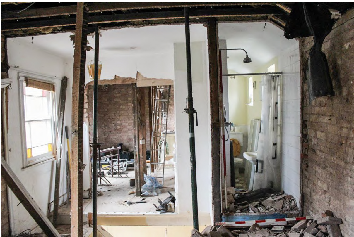
Plate 82: First floor following soft strip, looking south-west (LMSC16 D103 (24))
