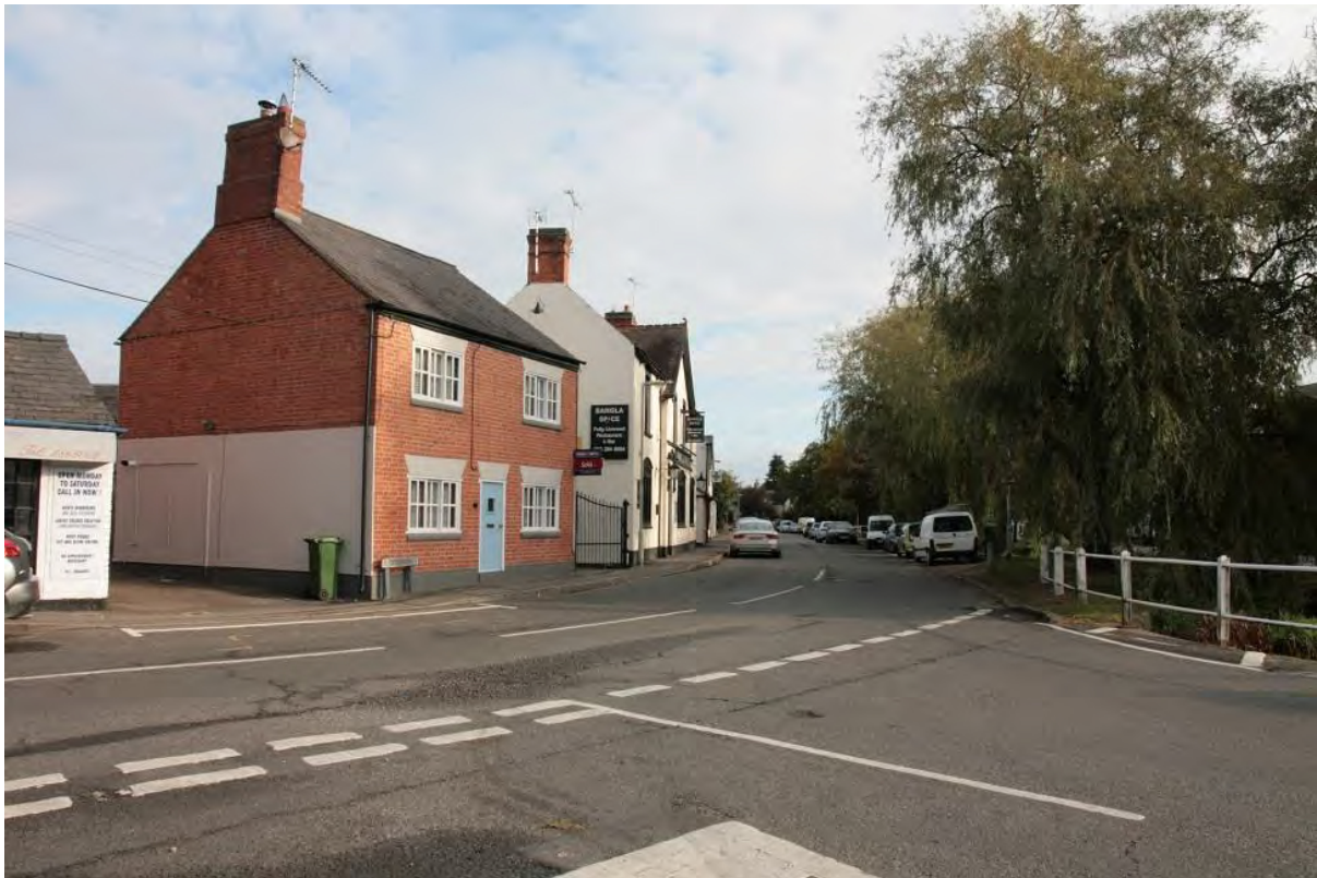
Plate 1: No. 79 Main Street, looking north-east (LMSC16 D100 (1))
