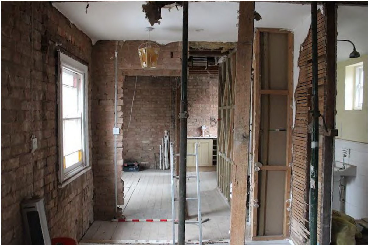
Plate 81: First floor following soft strip, looking south-west (LMSC16 D104 (26))
