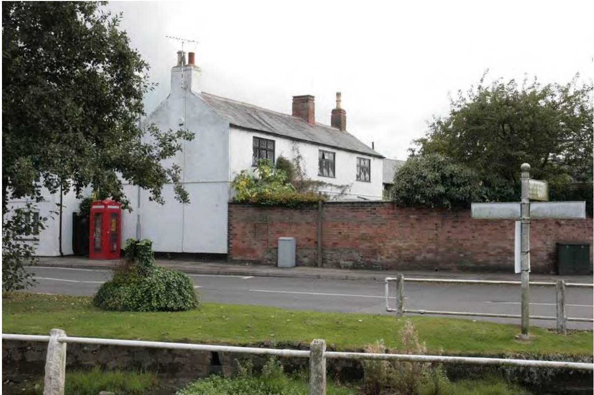
Plate 101: Brick garden wall with stone rubble plinth on the south side of The Nook, Cosby, looking south (LMSC16 D100 (133))
