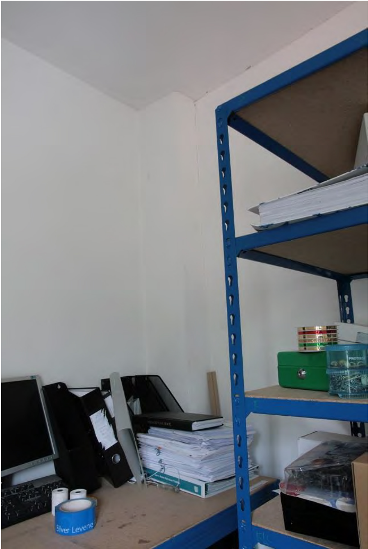
Plate 68: Chimney breast in the west corner of the First Floor Store Room, looking west (LMSC16 D100 (75))
