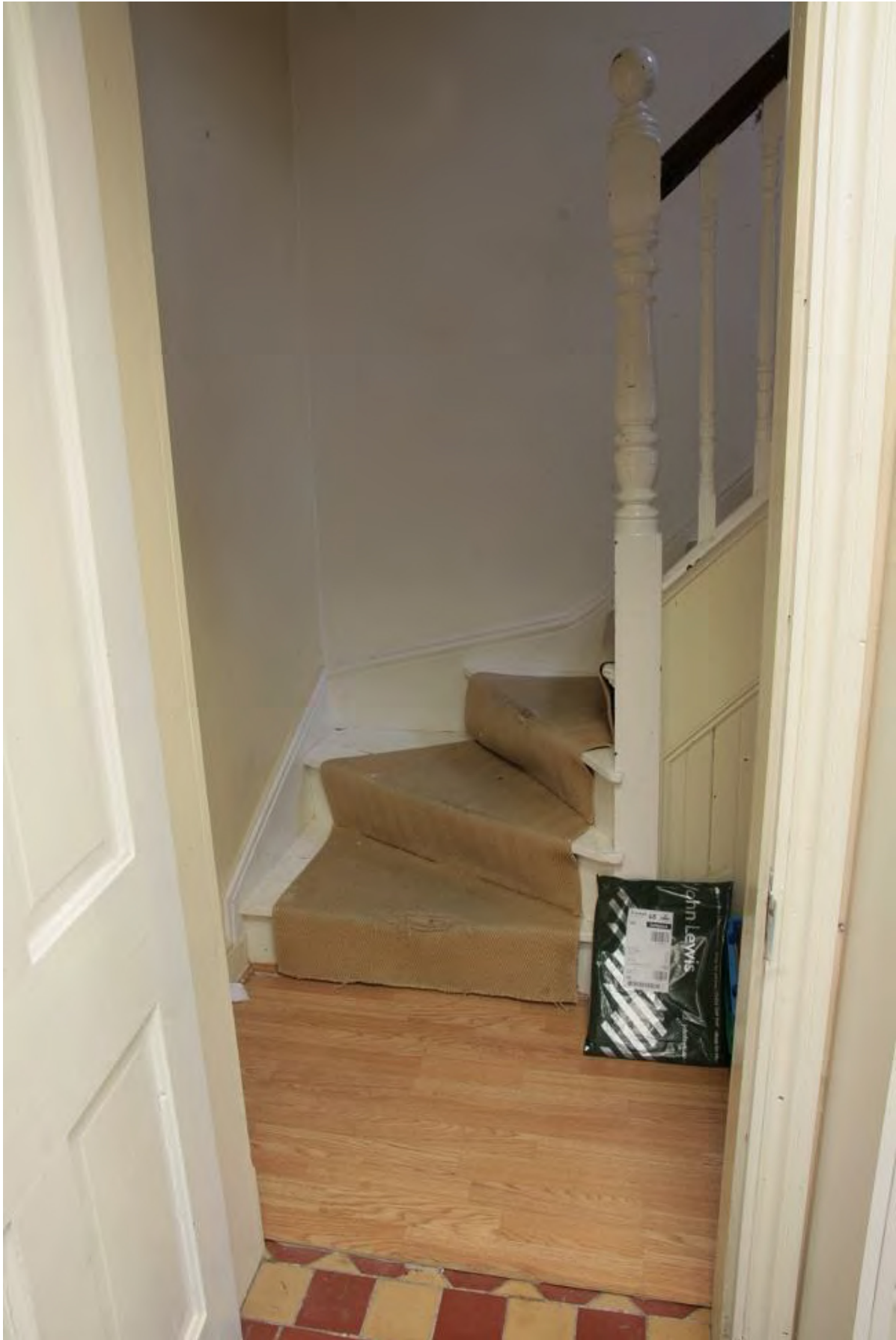
Plate 46: Staircase to first floor in Entrance Lobby, looking north (LMSC16 D100 (52))
