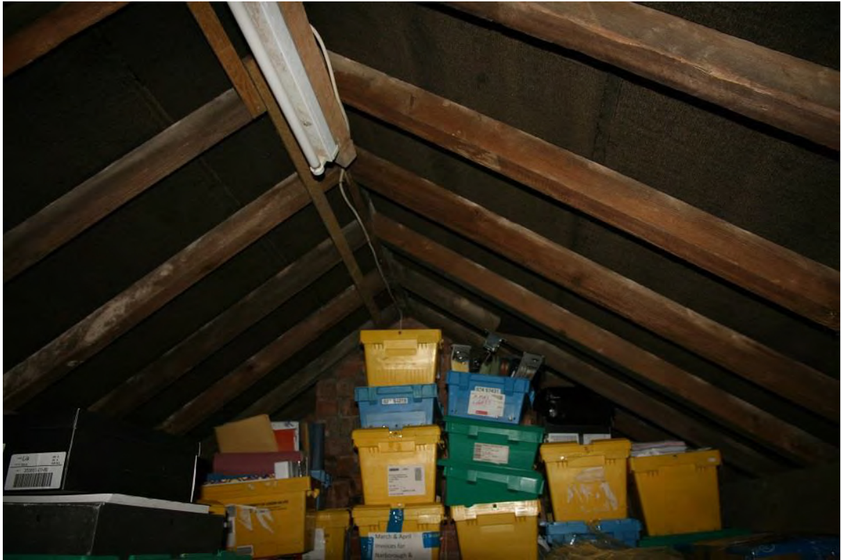
Plate 91: Attic space, looking south-west (LMSC16 D100 (91))
