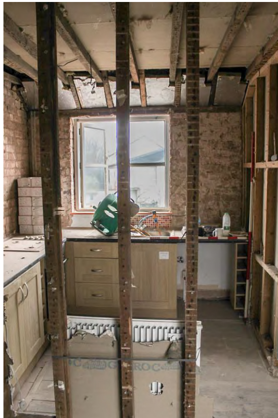
Plate 77: Kitchen following soft strip, looking north-west (LMSC16 D100 (80))
