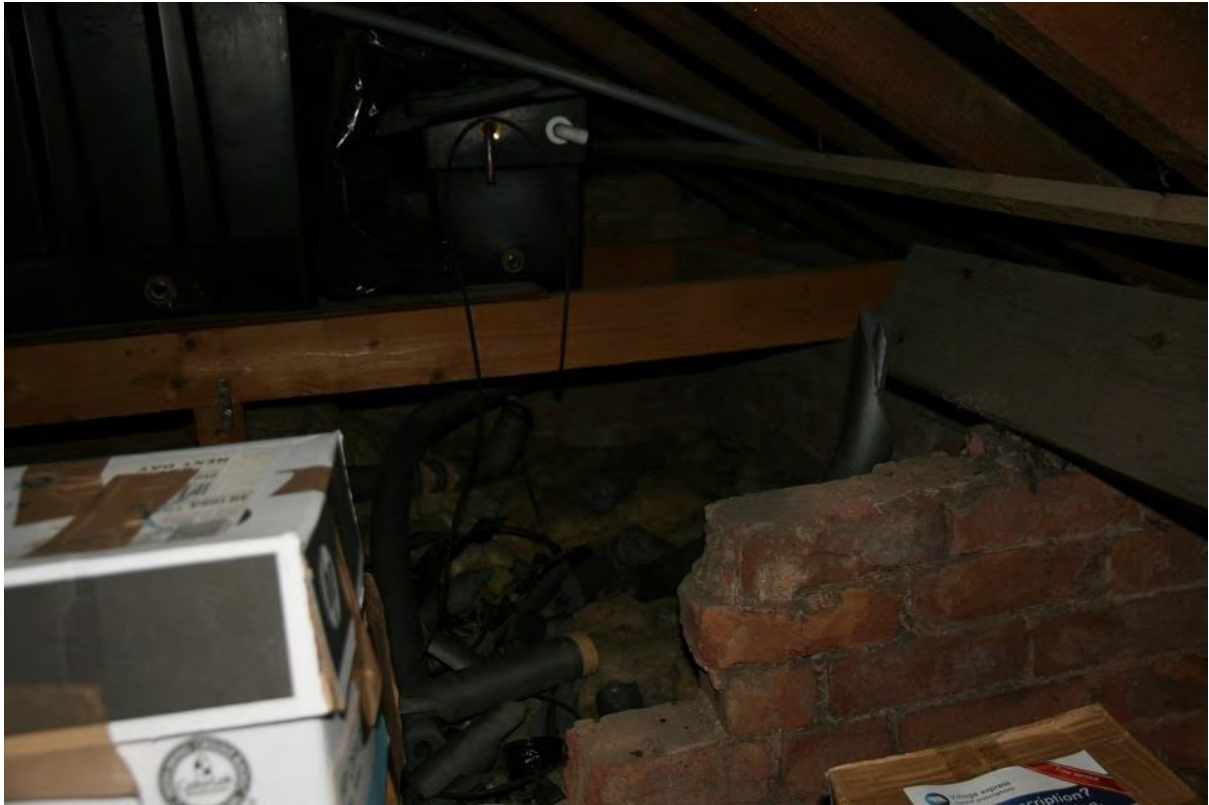
Plate 95: Attic space, looking east (LMSC16 D100 (101))
