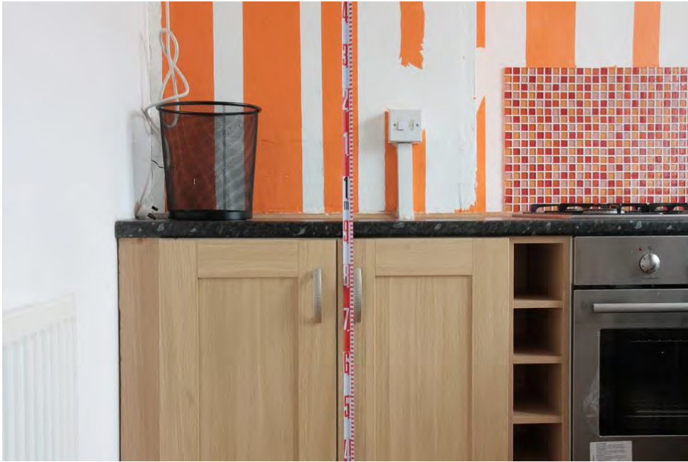
Plate 74: Original chimney breast in Kitchen, looking south-west (LMSC16 D100 (86))
