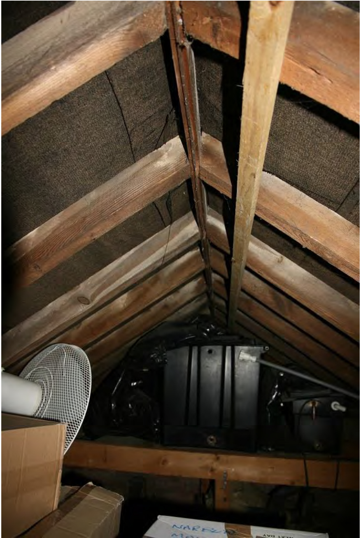
Plate 98: Attic space, looking up and north-east (LMSC16 D100 (105))
