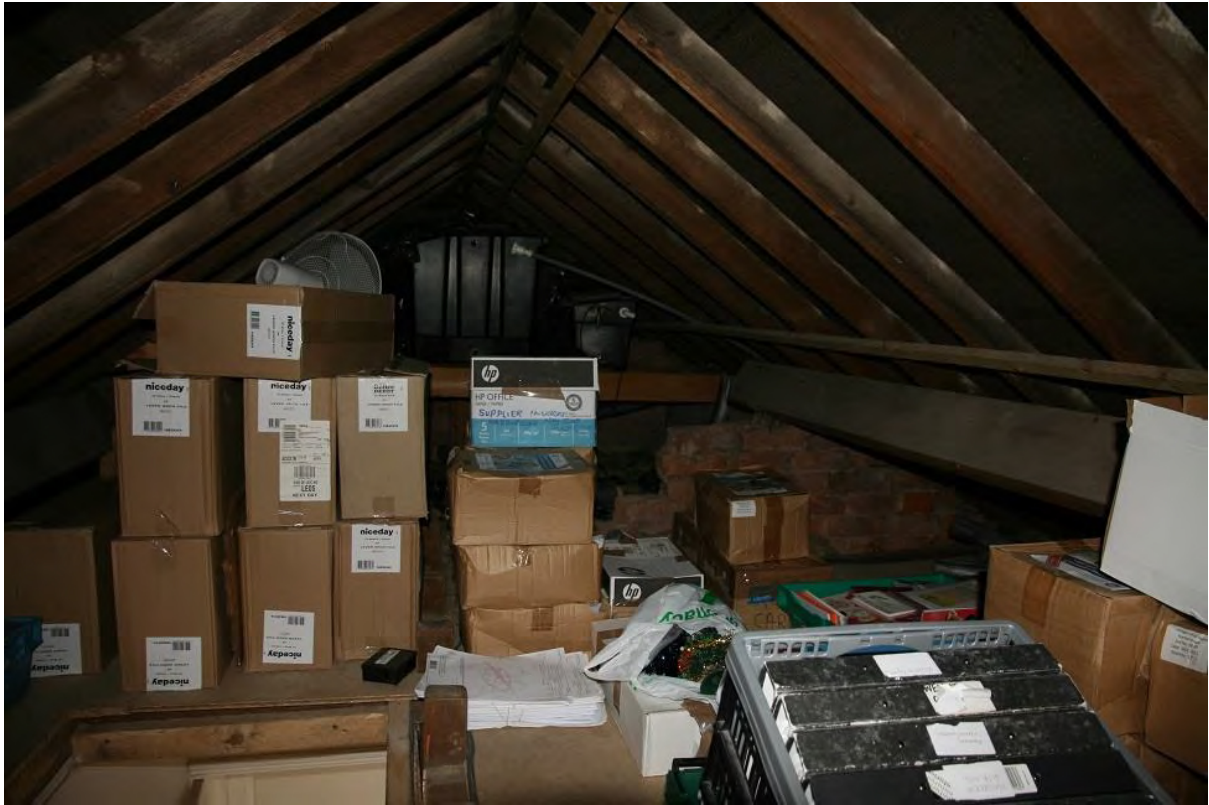
Plate 93: Attic space, looking north-east (LMSC16 D100 (96))
