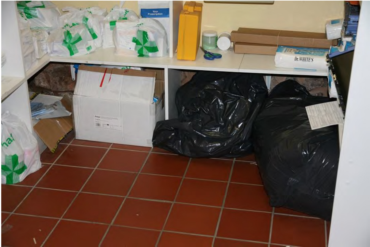
Plate 42: Stone rubble plinth visible at the base of the north-east wall in the Med. Store, looking north-east (LMSC16 D100 (48))
