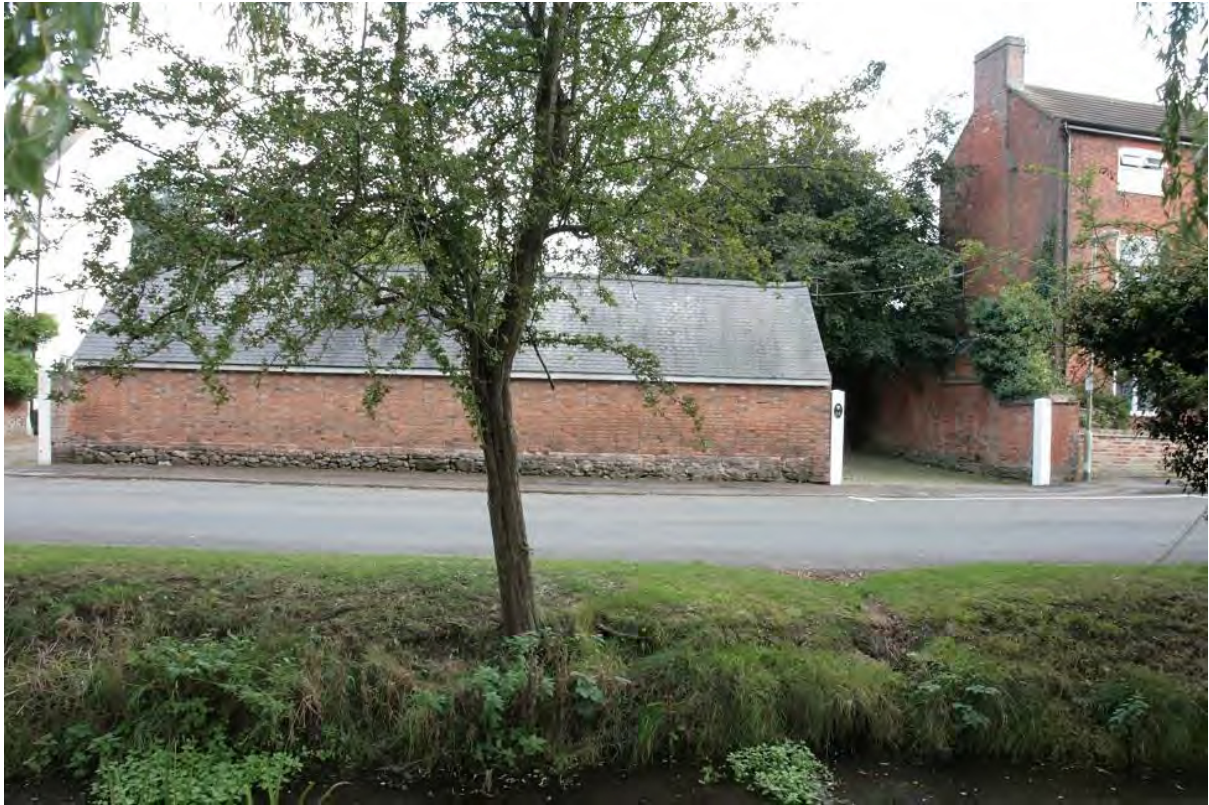
Plate 99: Stone rubble plinth at base of brick building on the south-east side of Main Street, Cosby, looking south-east (LMSC16 D100 (131))
