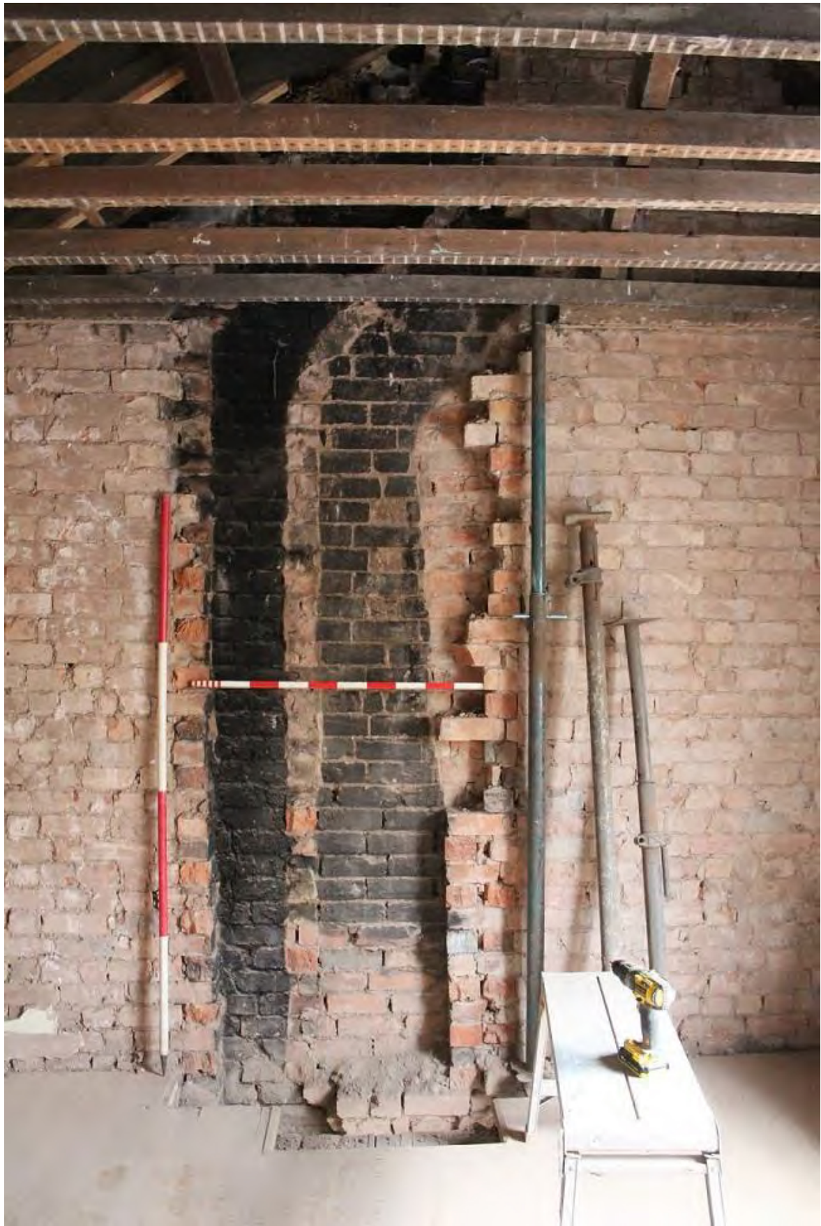
Plate 86: North-east wall of Staff Room following demolition, looking north-east (LMSC16 D104 (18))
