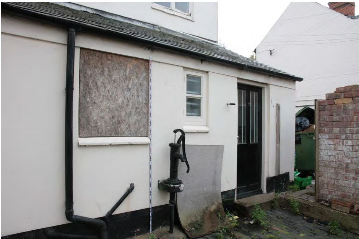
Plate 16: North-west (rear) elevation, looking south (LMSC16 D100 (120))
