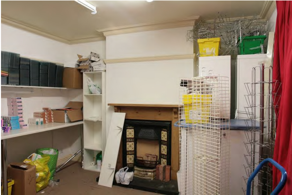
Plate 53: Staff/Store Area, looking north (LMSC16 D100 (60))
