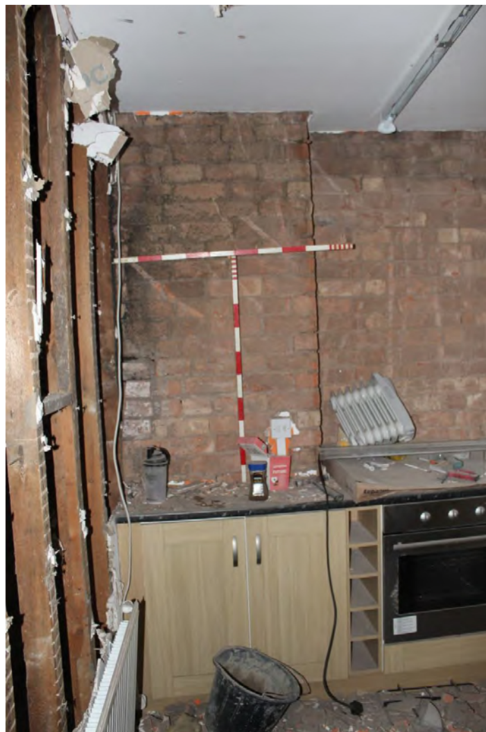
Plate 75: Kitchen, looking south-west (LMSC16 D100 (79))
