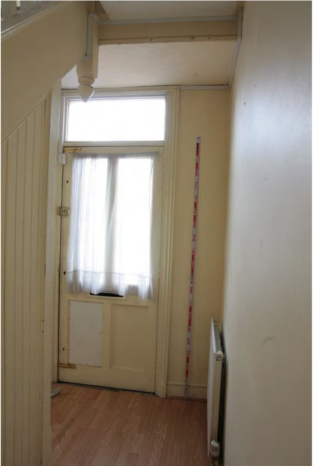
Plate 49: Front door in the Entrance Lobby, looking south-east (LMSC16 D100 (53))
