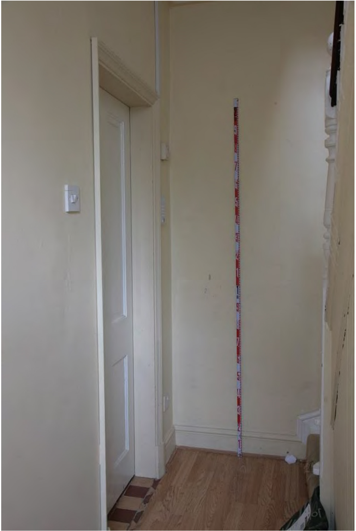
Plate 47: Entrance Lobby, looking north-west (LMSC16 D100 (55))
