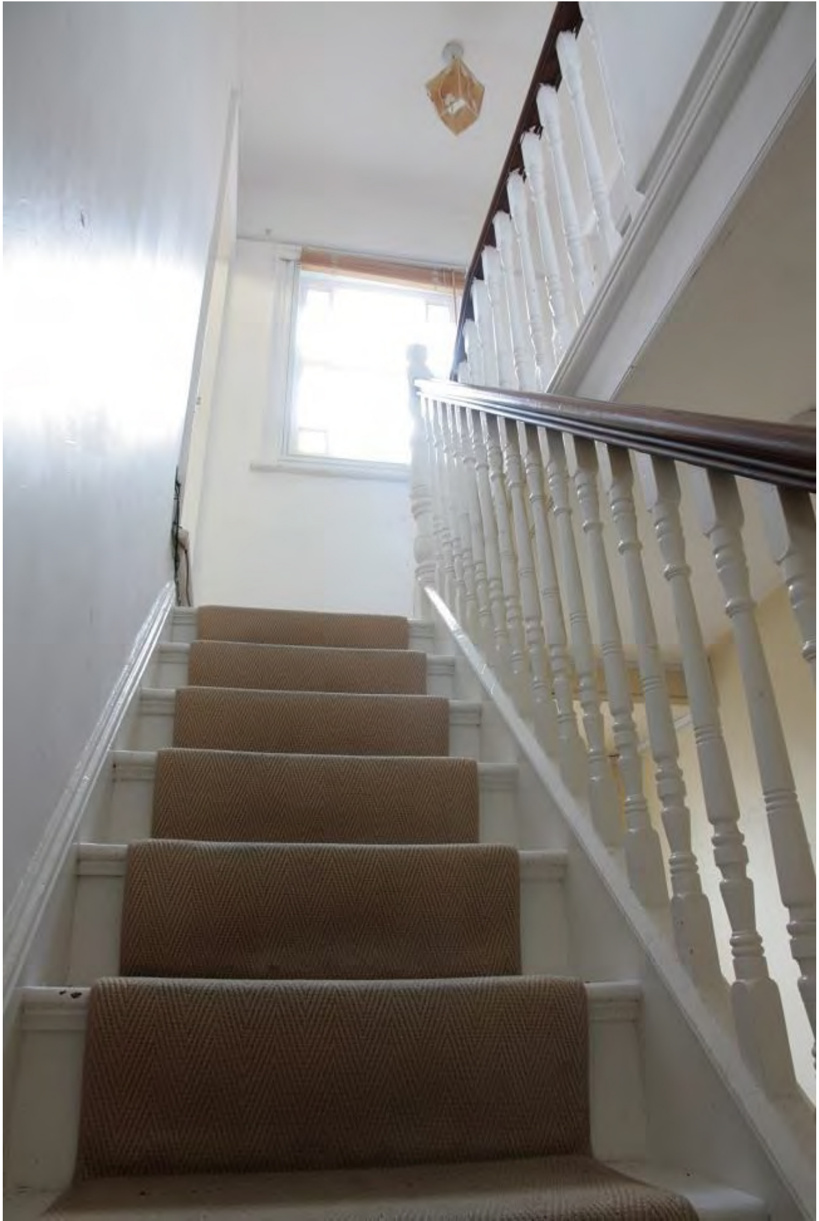
Plate 62: Staircase viewed from ground floor, looking southeast (LMSC16 D100 (71))
