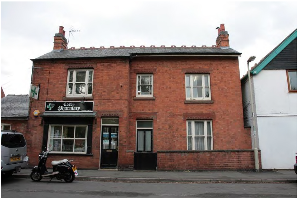
Plate 5: South-east (front) elevation, looking north-west (LMSC16 D100 (18))
