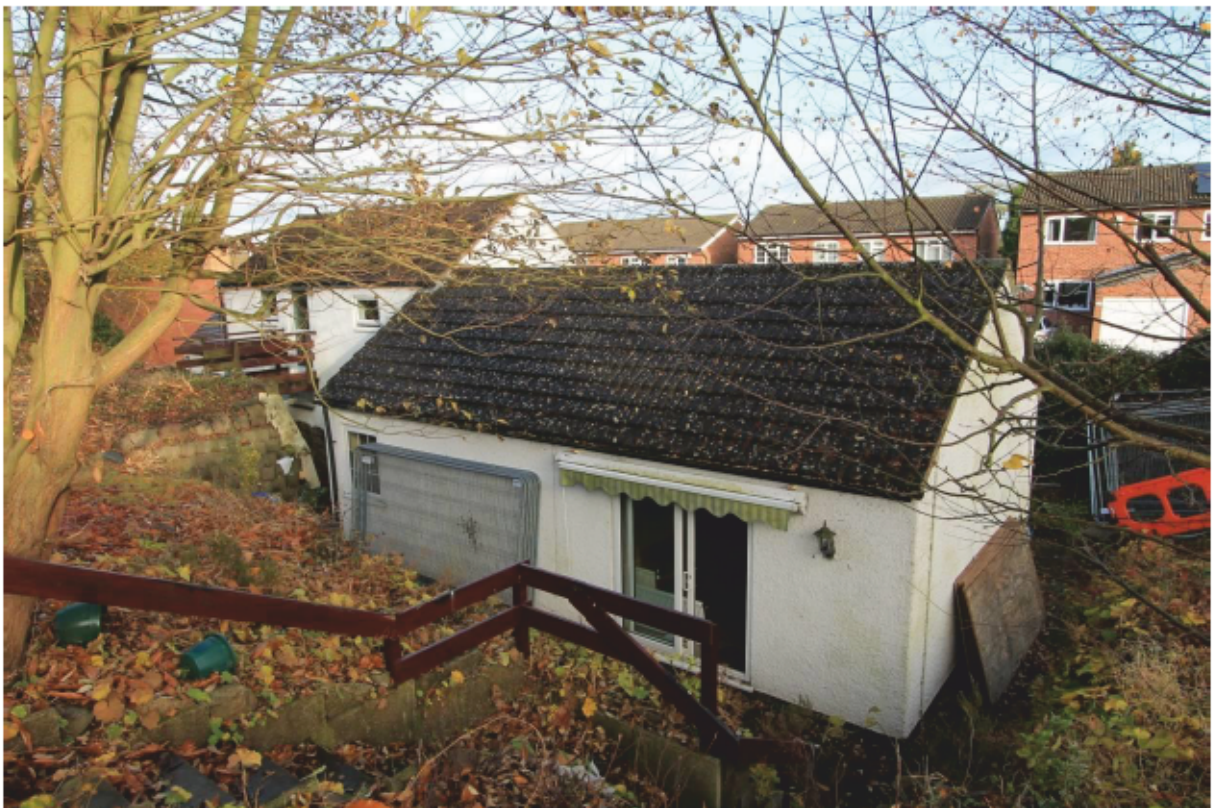
Plate 10 South-east extension, looking north
