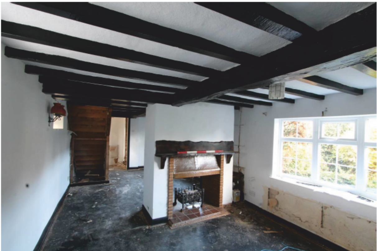
Plate 12 Lounge (G1), looking north
