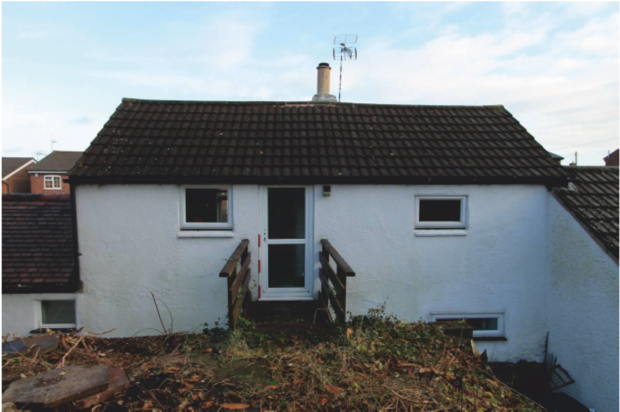
Plate 7 South-west rear elevation, looking north-east
