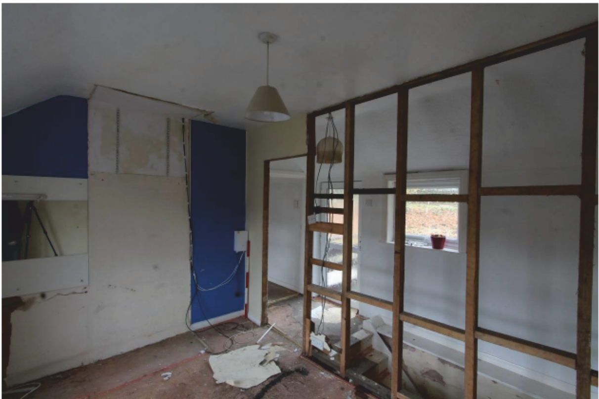
Plate 24 Bedroom (F6) showing inserted stud wall, looking south
