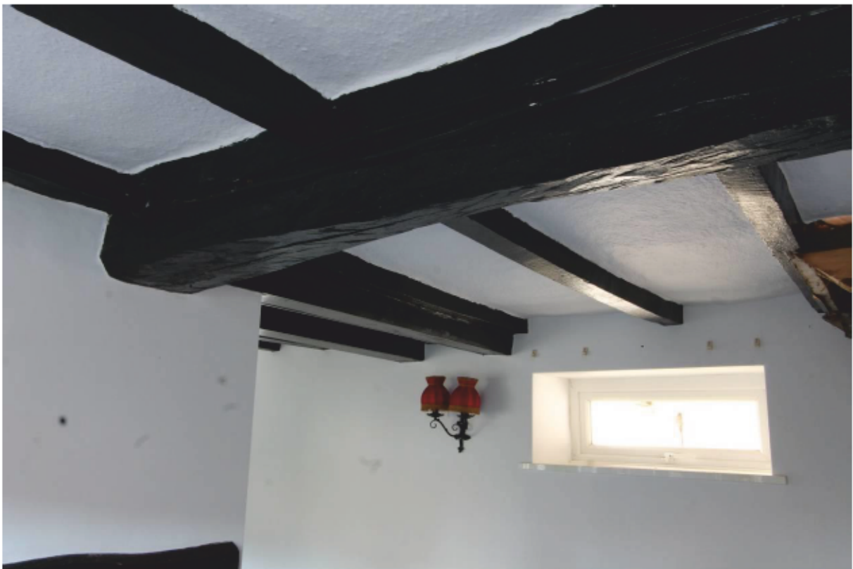
Plate 14 Detail of bridging beam (G2), looking south
