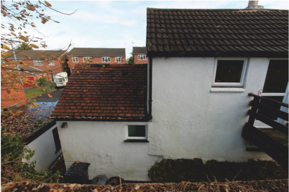
Plate 11 North-west extension, looking north-east
