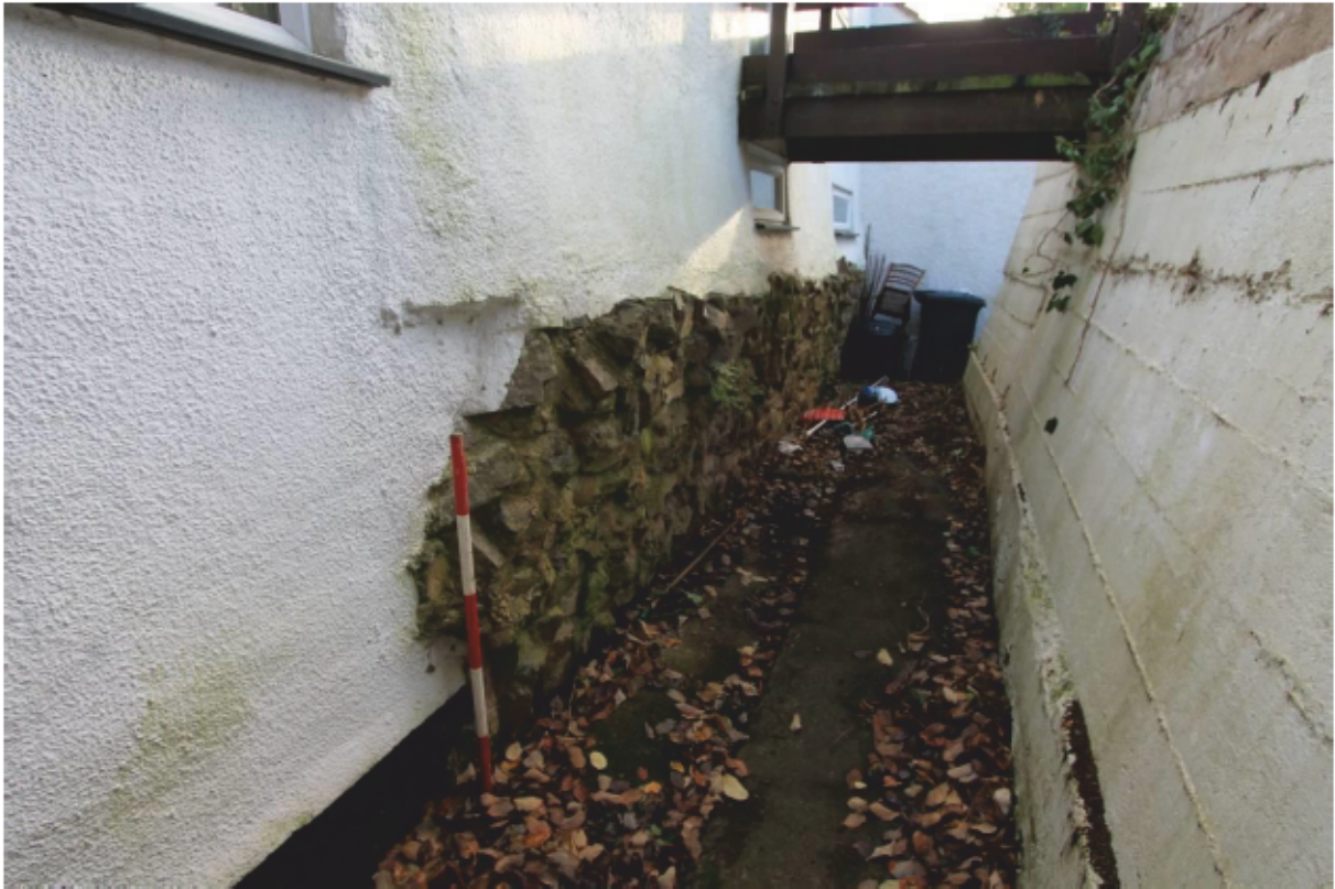
Plate 9 Masonry lower wall/foundation and revetment, looking south-east
