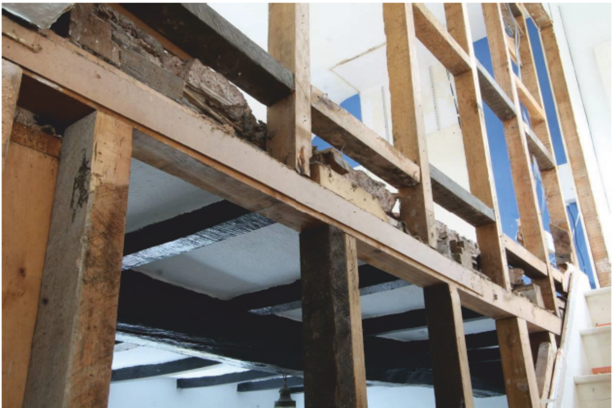
Plate 18 Modern stud wall enclosing staircase and bedroom (F6), looking east
