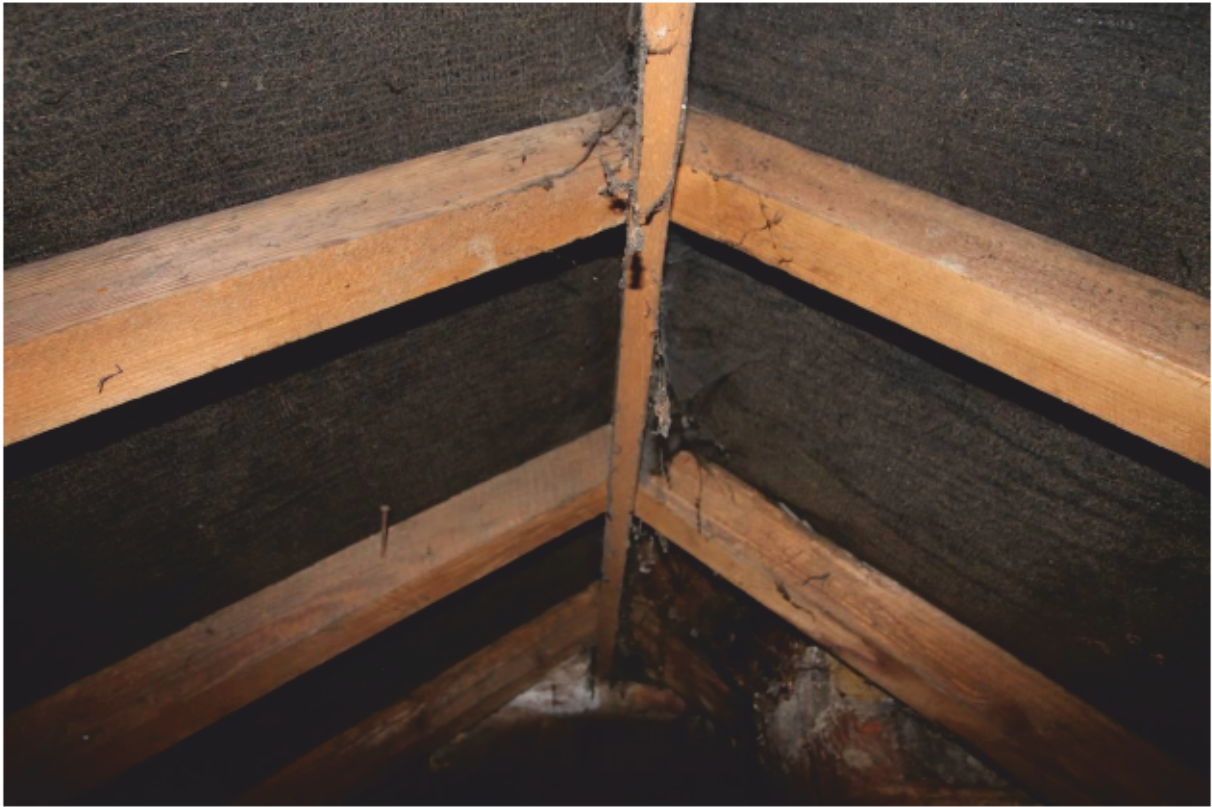
Plate 29 Replaced softwood roof structure
