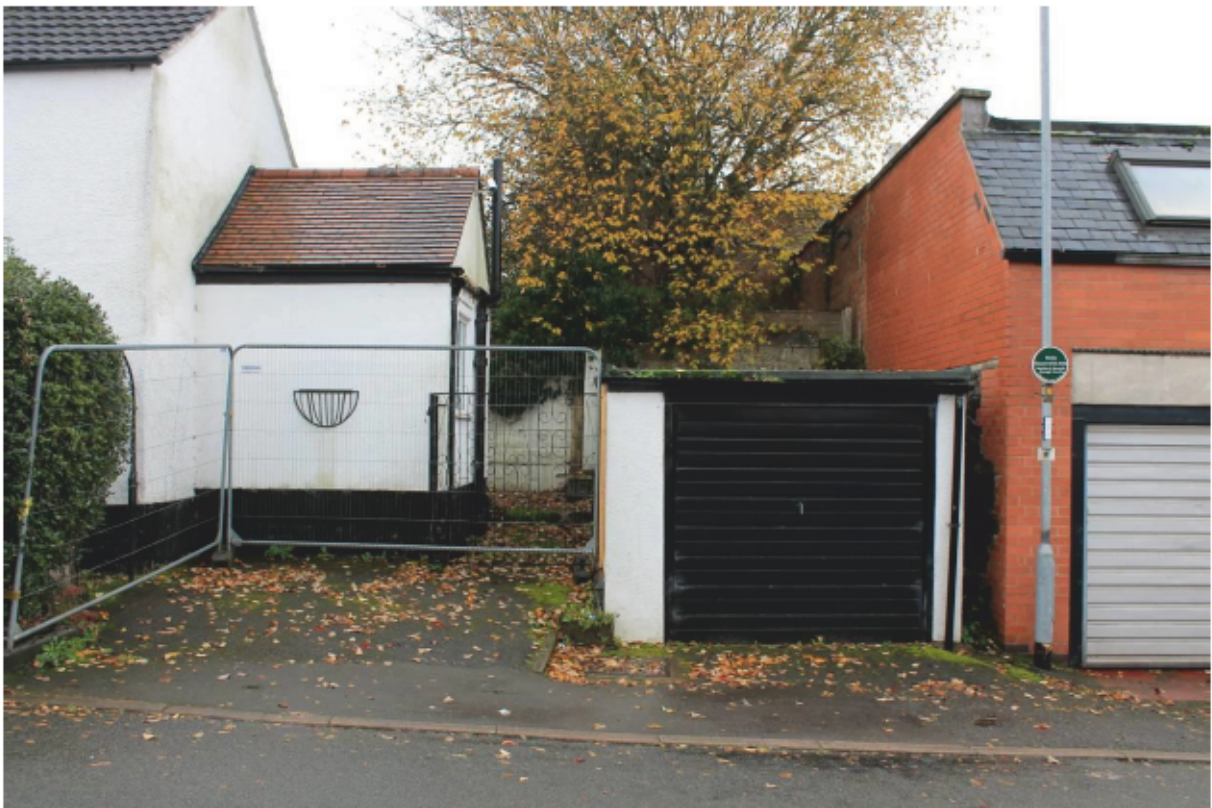
Plate 4 North-west extension and garage, looking south-west
