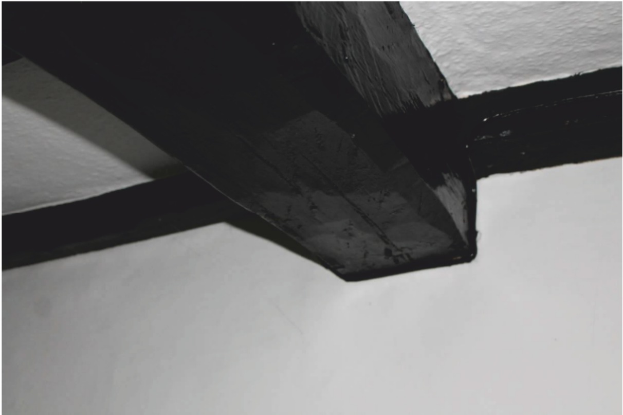
Plate 15 Run-out stop to soffit (G1), looking east
