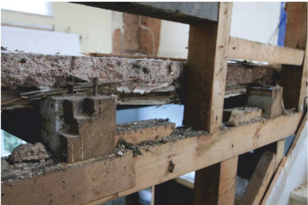
Plate 20 Corresponding (mirror) dovetail lap joint to north-west, looking east
