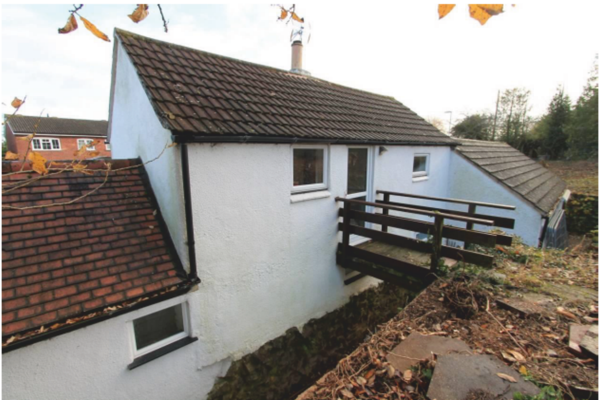
Plate 8 South-west rear elevation showing revetment/bank, looking east
