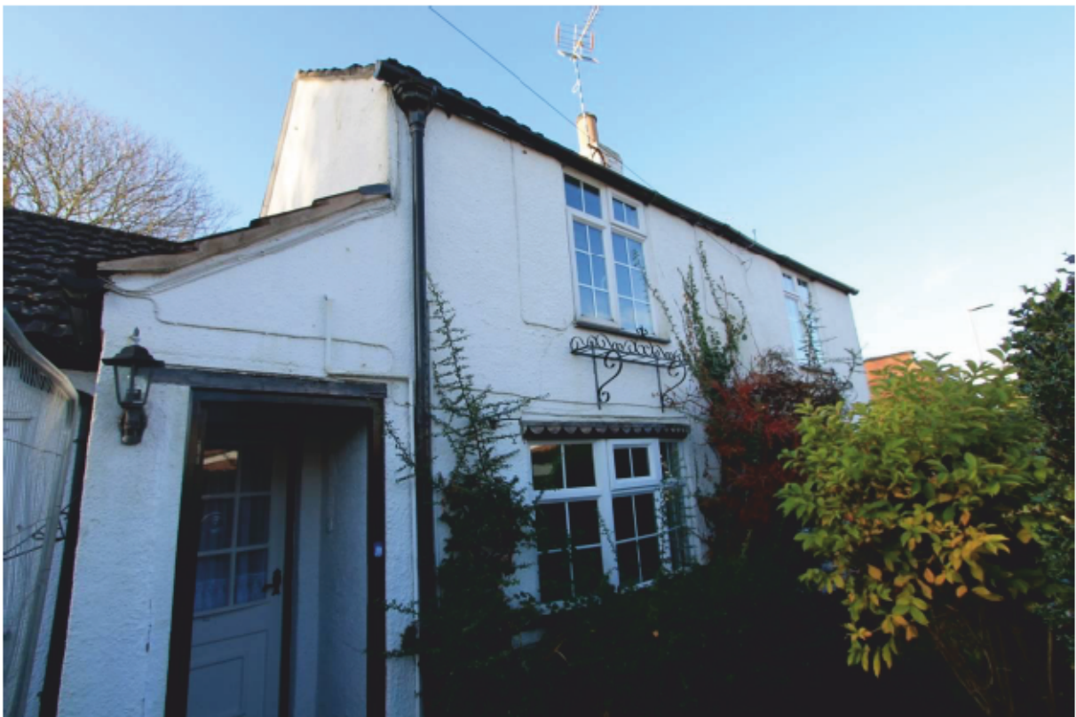
Plate 2 Facade of no. 20 Rookery Lane, looking north-west
