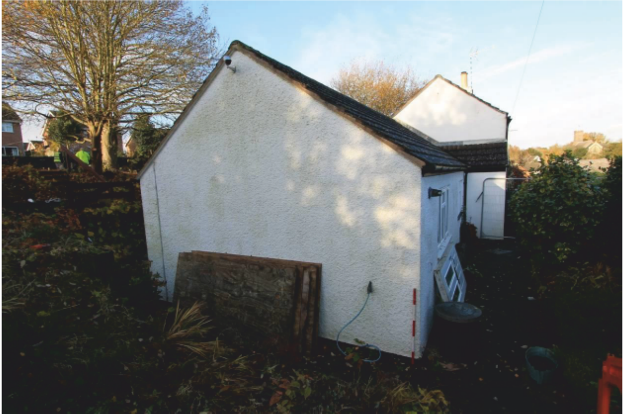
Plate 5 South-east extension, looking north-west
