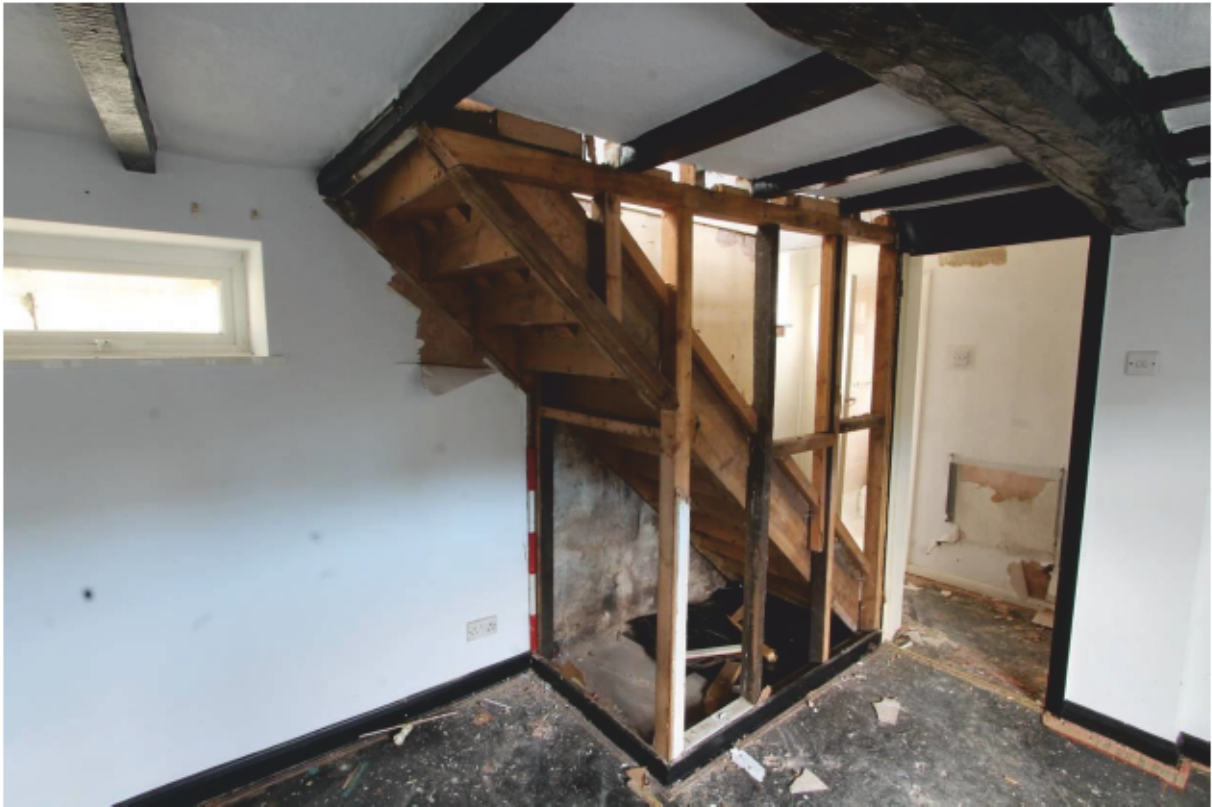
Plate 17 Modern inserted staircase (G2), looking west
