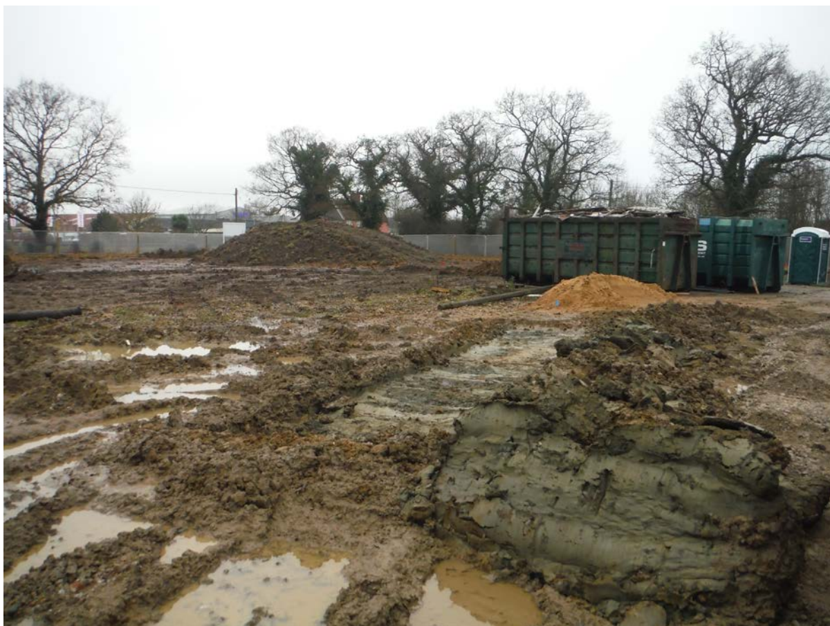
Plate 4: The site and Trench 9, view north
