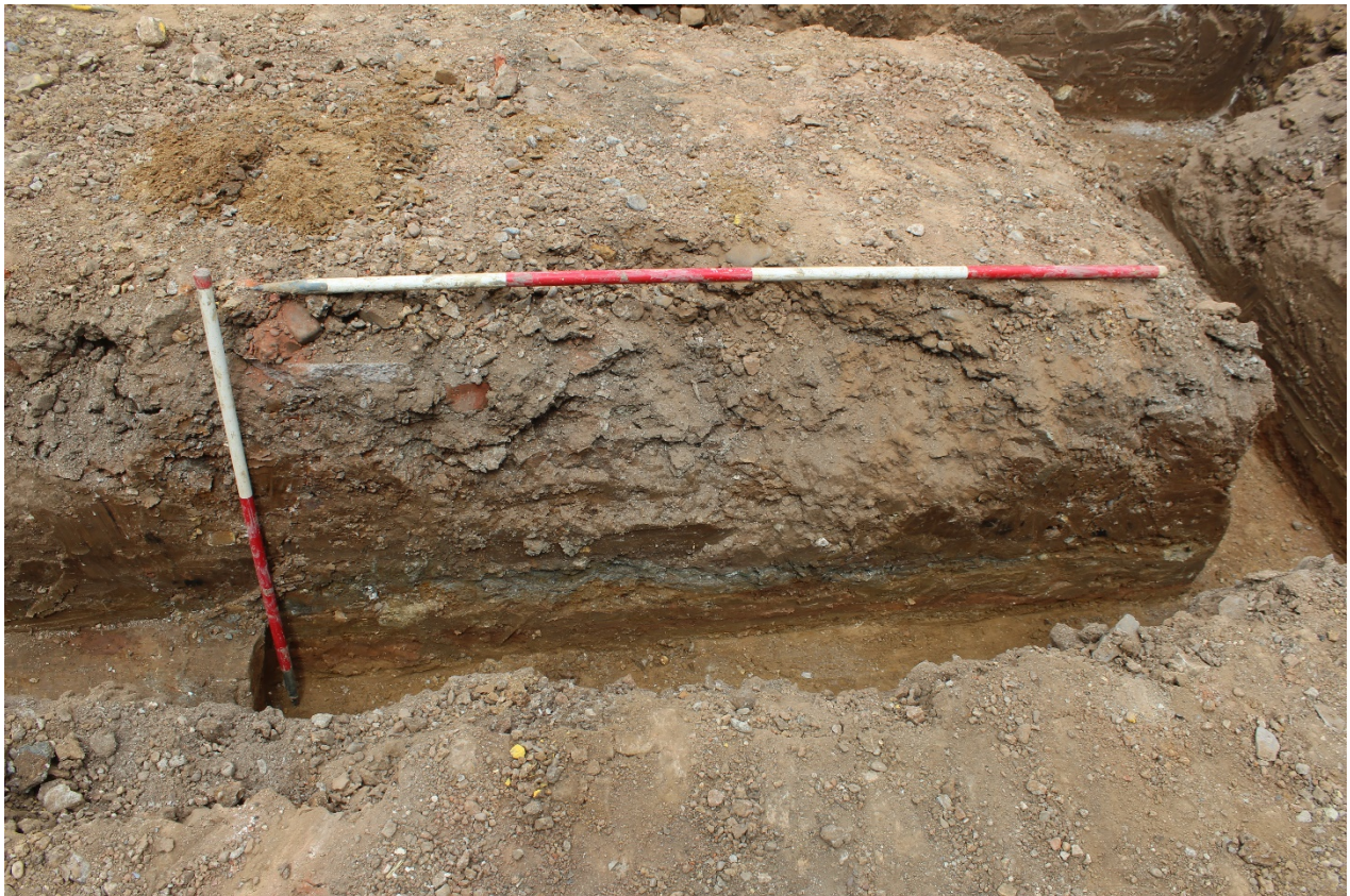
Plate 4: View of Section 3; taken facing north-northwest.
