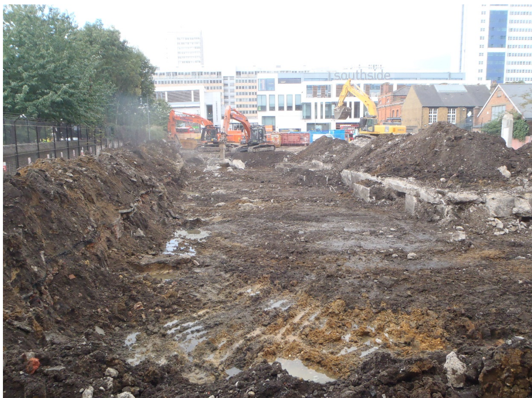
Plate 2. West facing shot of excavations, showing view towards Garratt Lane.
