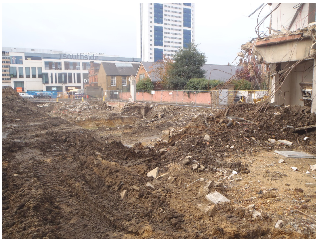
Plate 3. West facing shot of site, showing areas exposed during obstruction removal.
