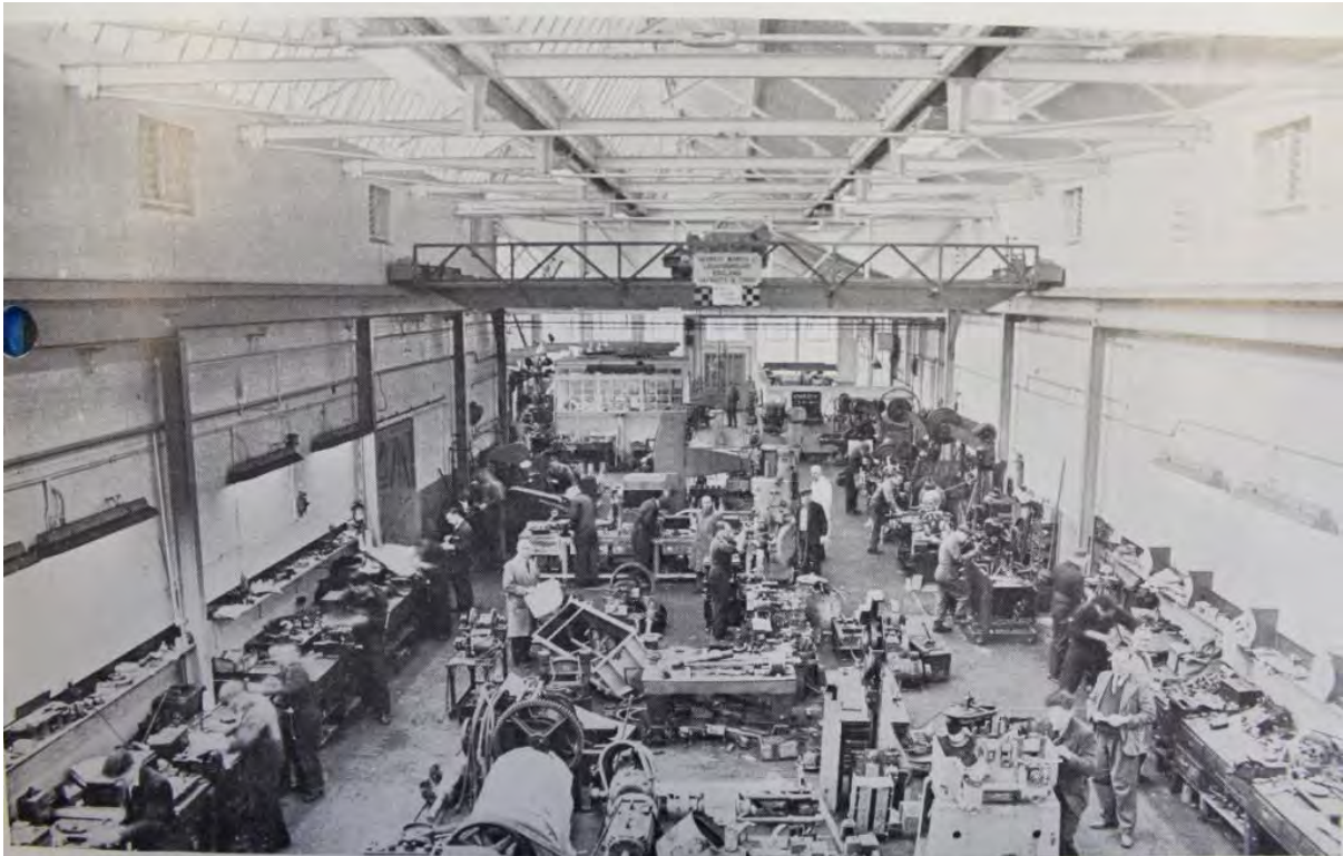
Plate 51: Photograph of the interior of Building 2, Fitters Shop from Promotional Brochure, 1953 (SRO Ref. HC 410/G57)
