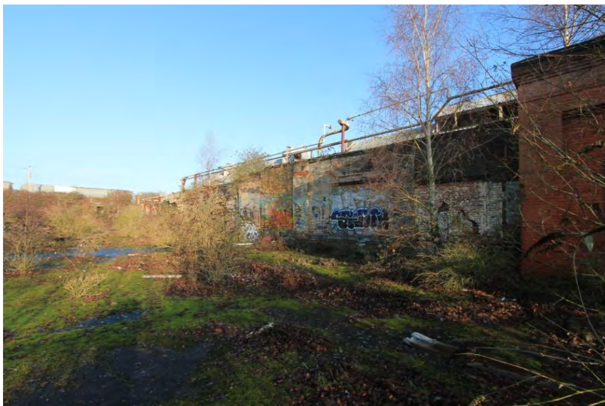
Plate 54: Building 3, viewed from south-west
