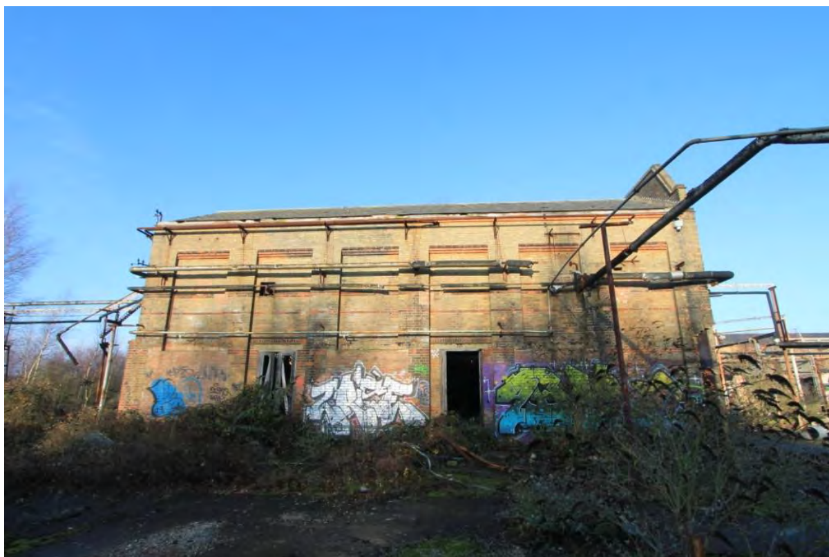
Plate 53: Building 3, viewed from south
