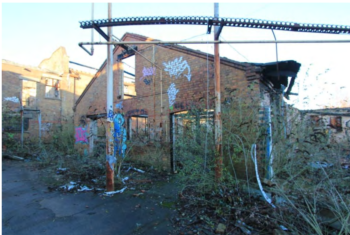
Plate 58: Building 4, viewed from south-west
