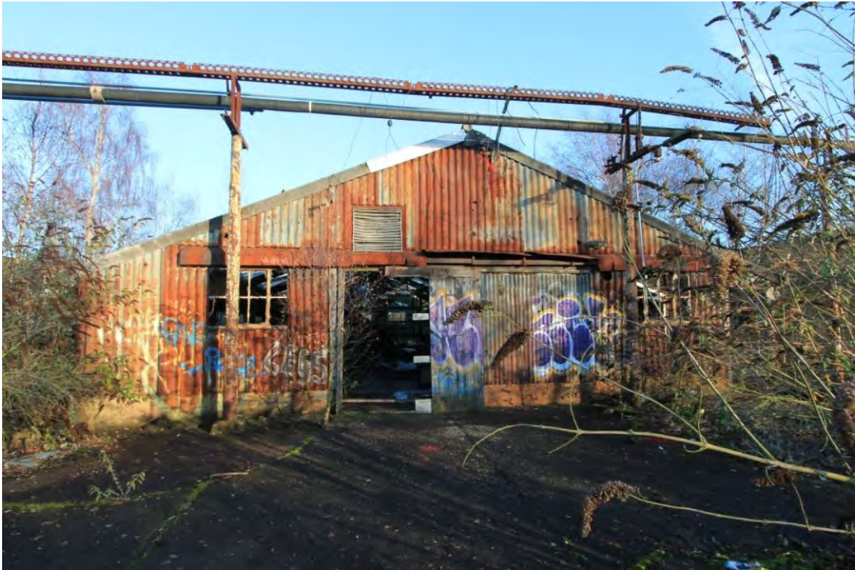
Plate 89: Building 16, viewed from south-west
