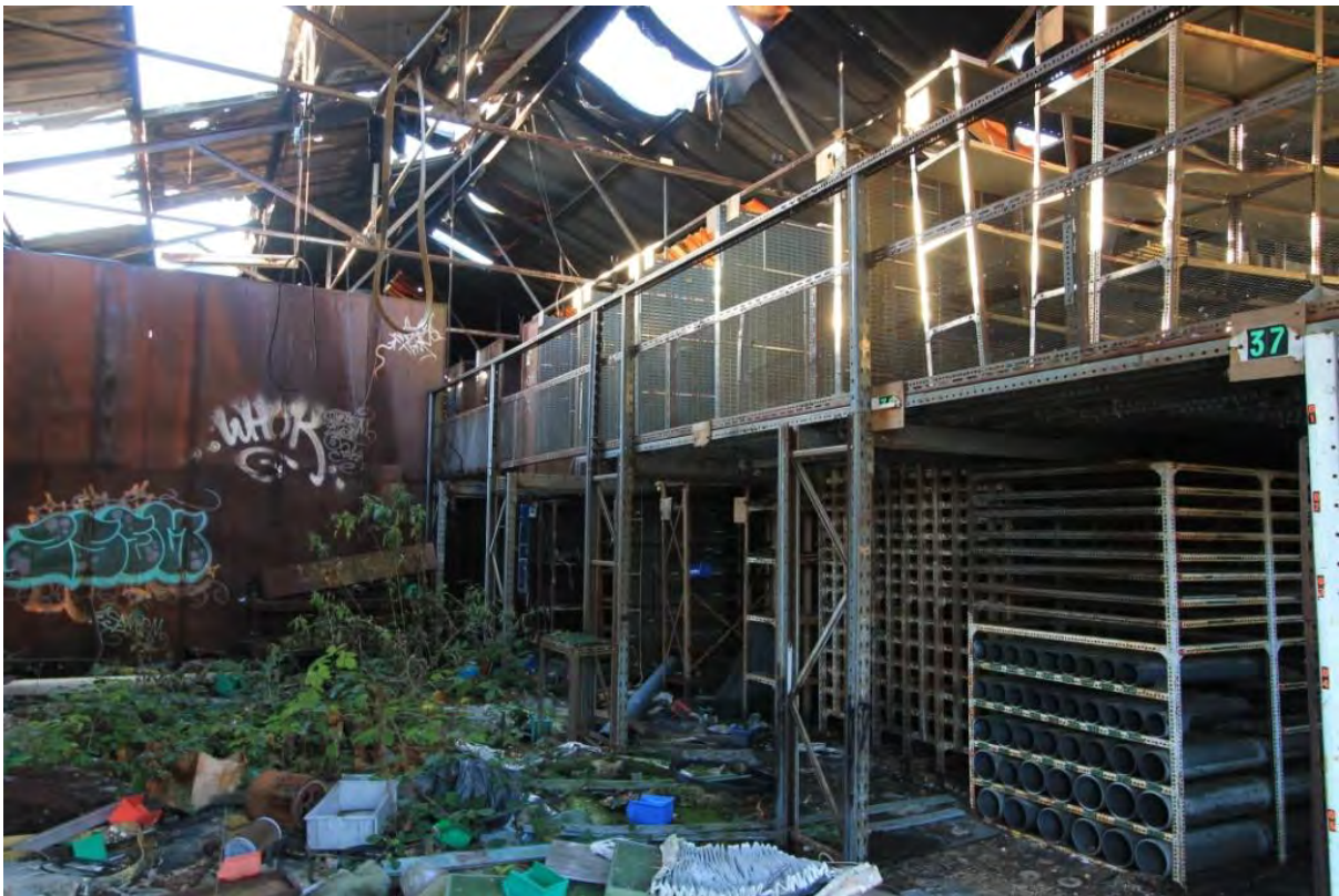
Plate 80: Building 13, interior view
