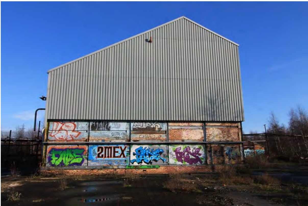
Plate 62: Building 6, viewed from south-west
