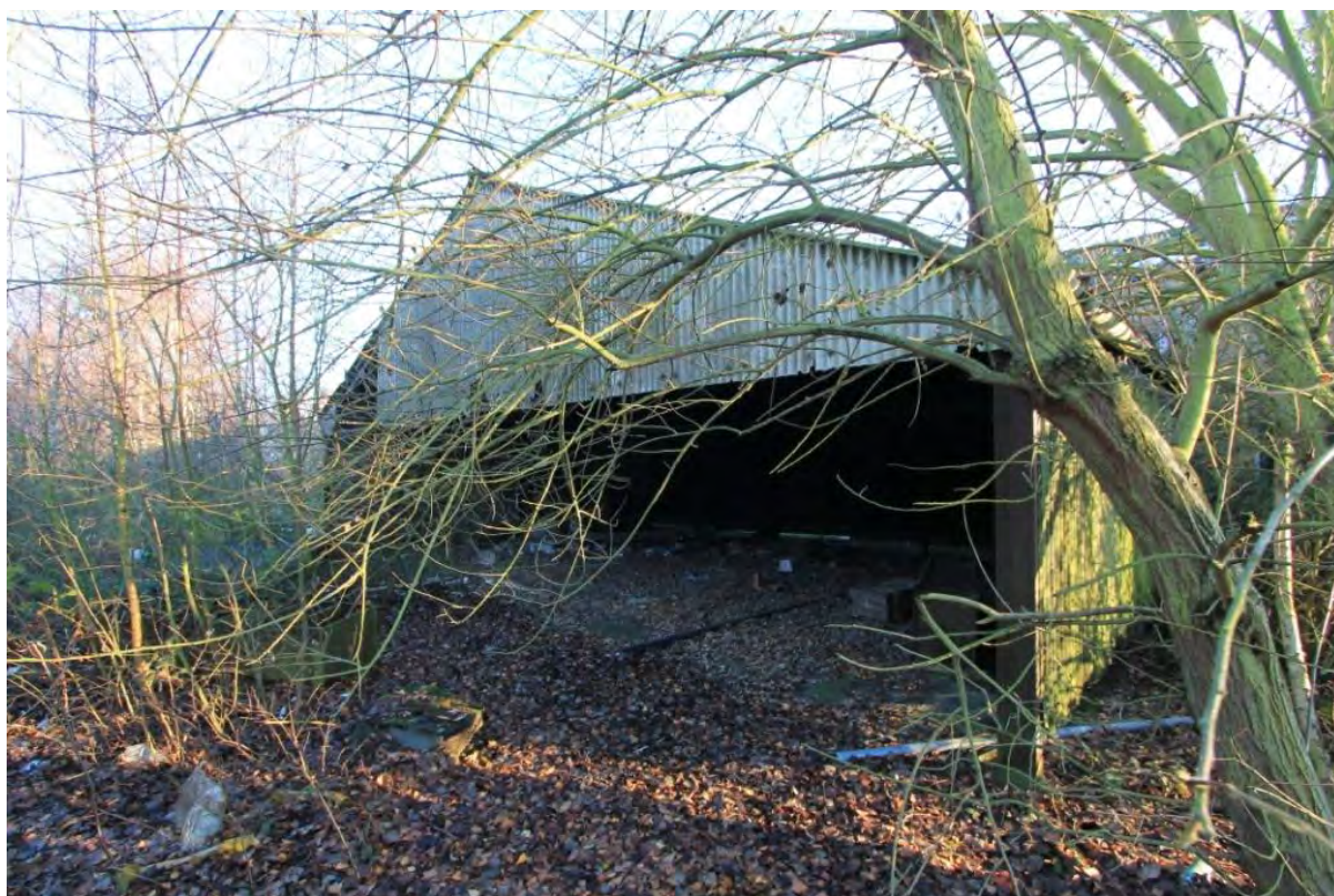
Plate 87: Building 15, viewed from north-west
