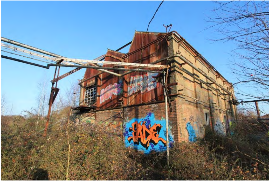
Plate 55: Building 3, viewed from south-west
