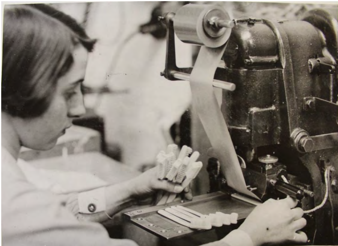
Plate 12 : Finishing toothbrush handles (SRO Ref. HC 410/J1/2)
