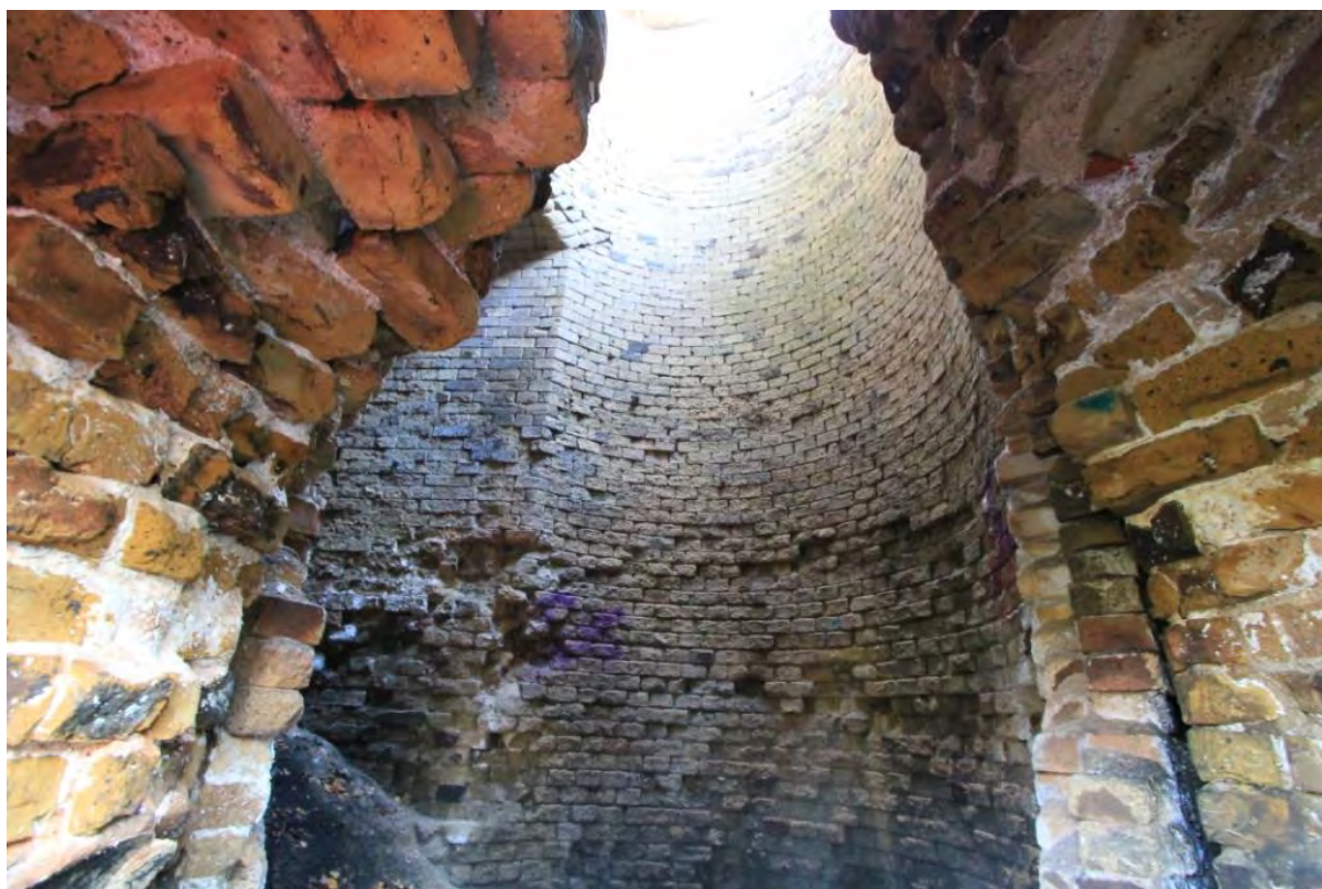
Plate 57: Building 3, detail of stack base interior
