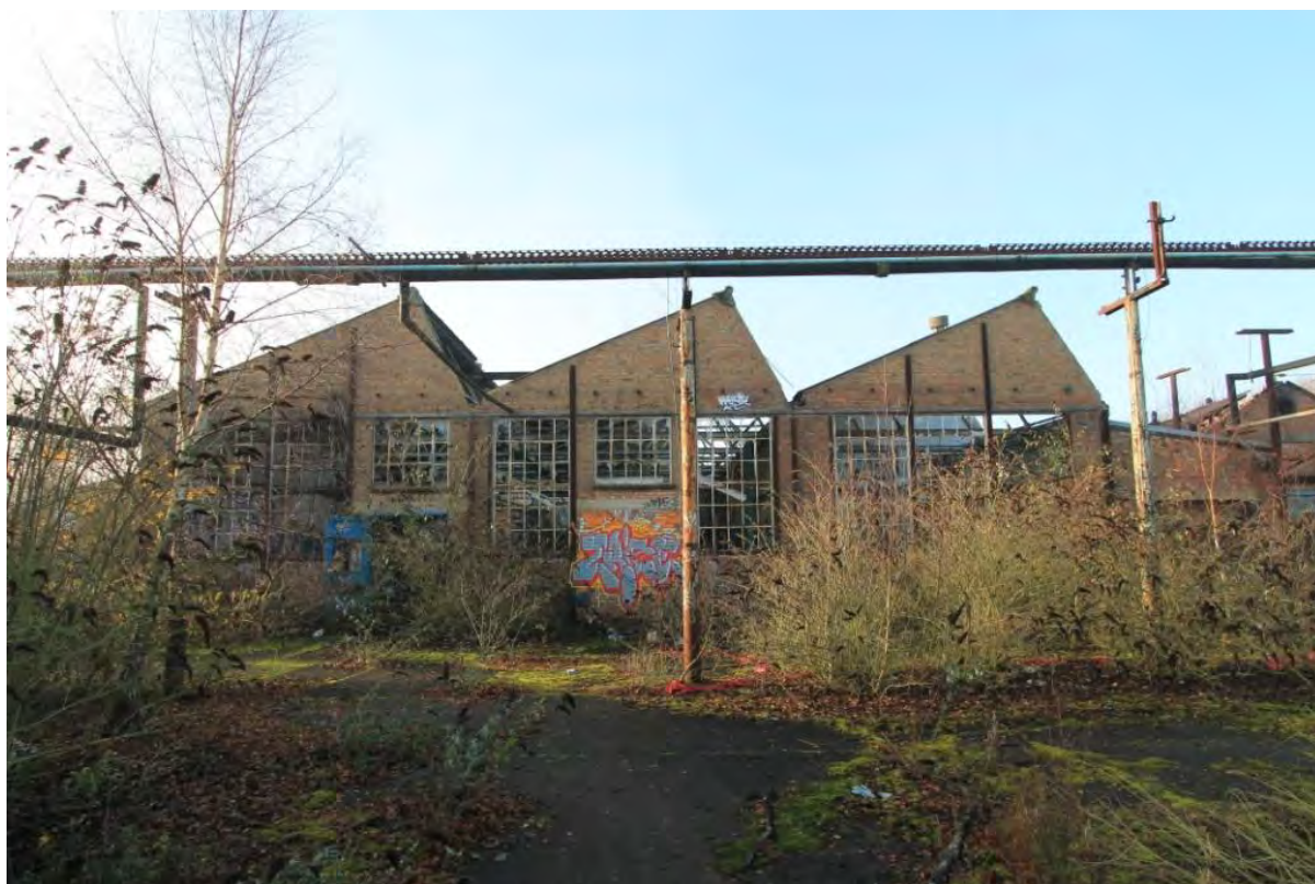
Plate 47: Building 2 as viewed from north-east
