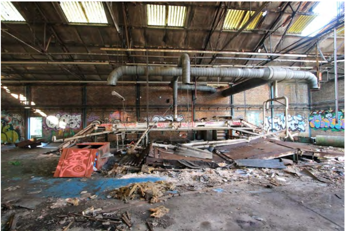
Plate 76: Building 11, interior view
