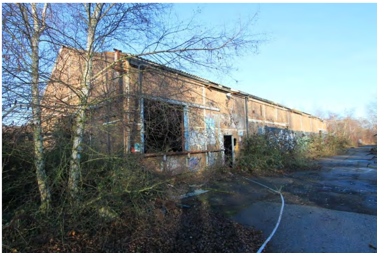
Plate 73: Building 11, viewed from south-west
