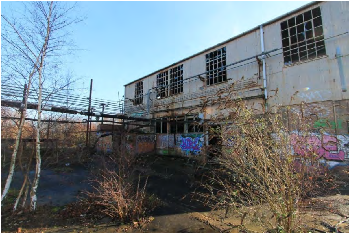
Plate 63: Building 6, viewed from north-west
