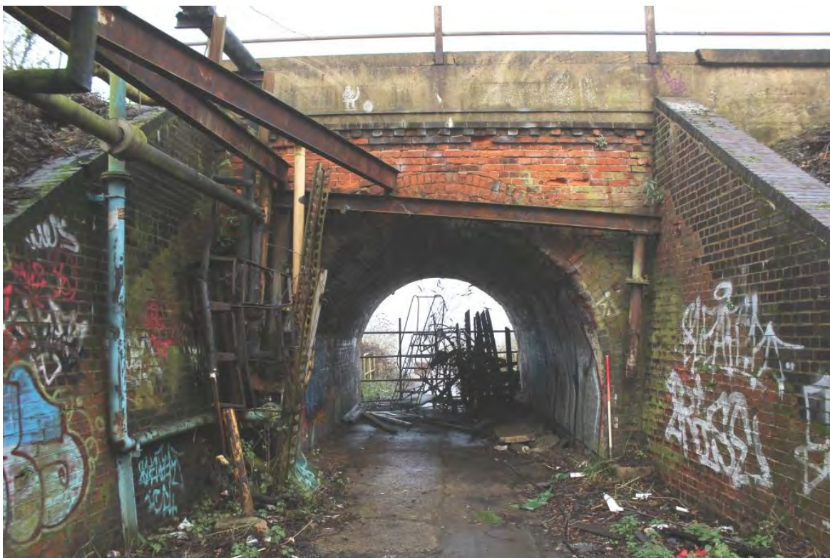
Plate 36: Tunnel beneath railway line as viewed from the south side
