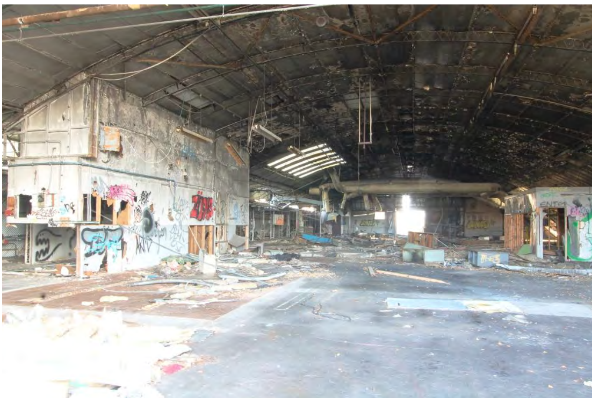
Plate 93: Building 18, interior view
