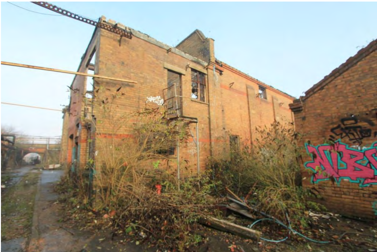
Plate 46: Building 2 as viewed from south
