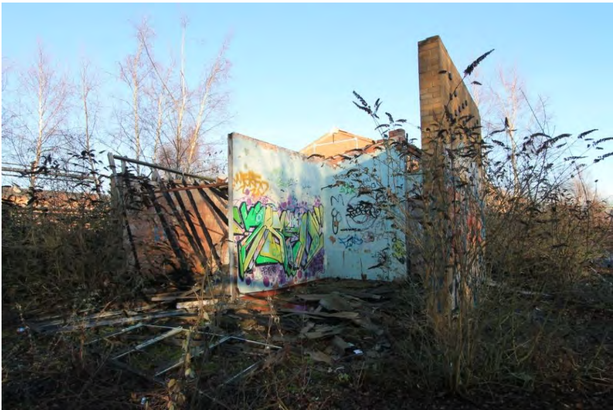
Plate 72: Building 10, viewed from south-west
