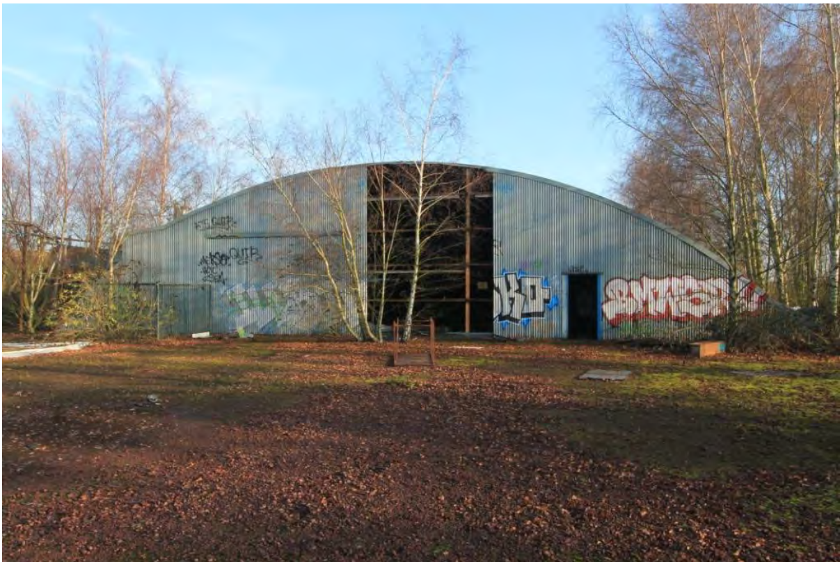
Plate 92: Building 18, viewed from south-west
