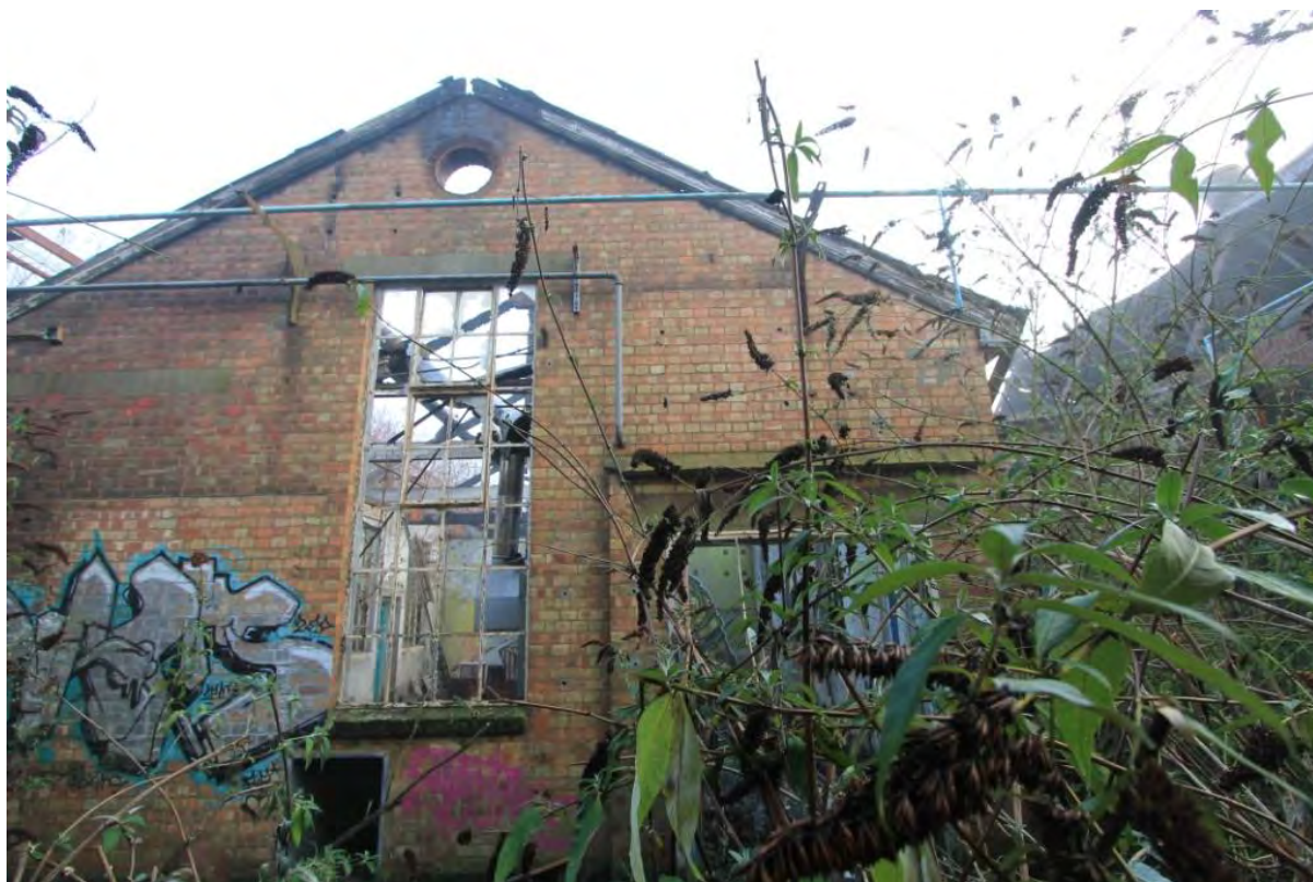
Plate 49: Building 2 as viewed from north-east
