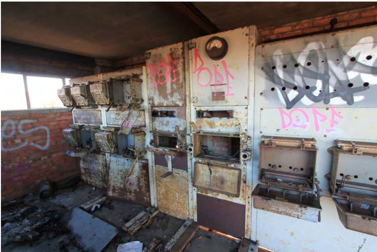
Plate 66: Building 7, interior view
