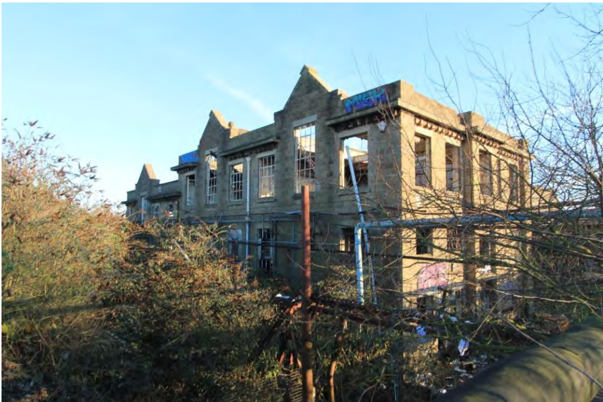
Plate 38: Building 1, as viewed from railway embankment
