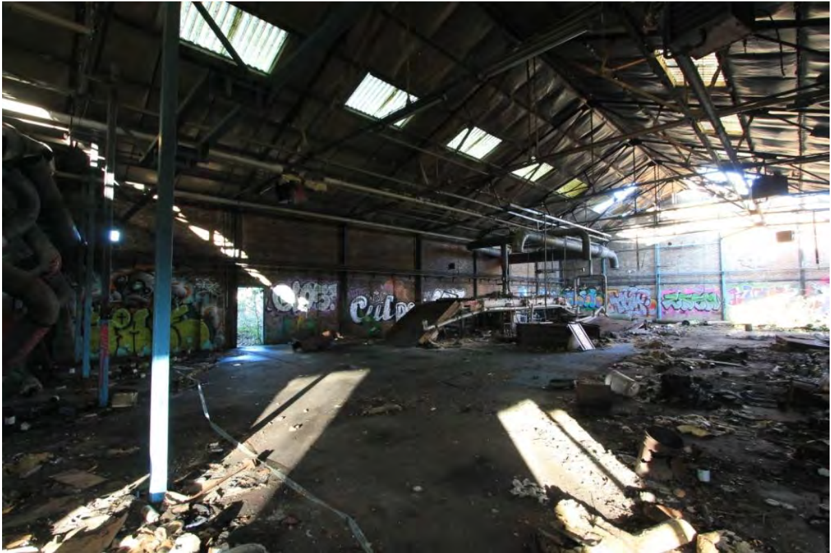
Plate 75: Building 11, interior view
