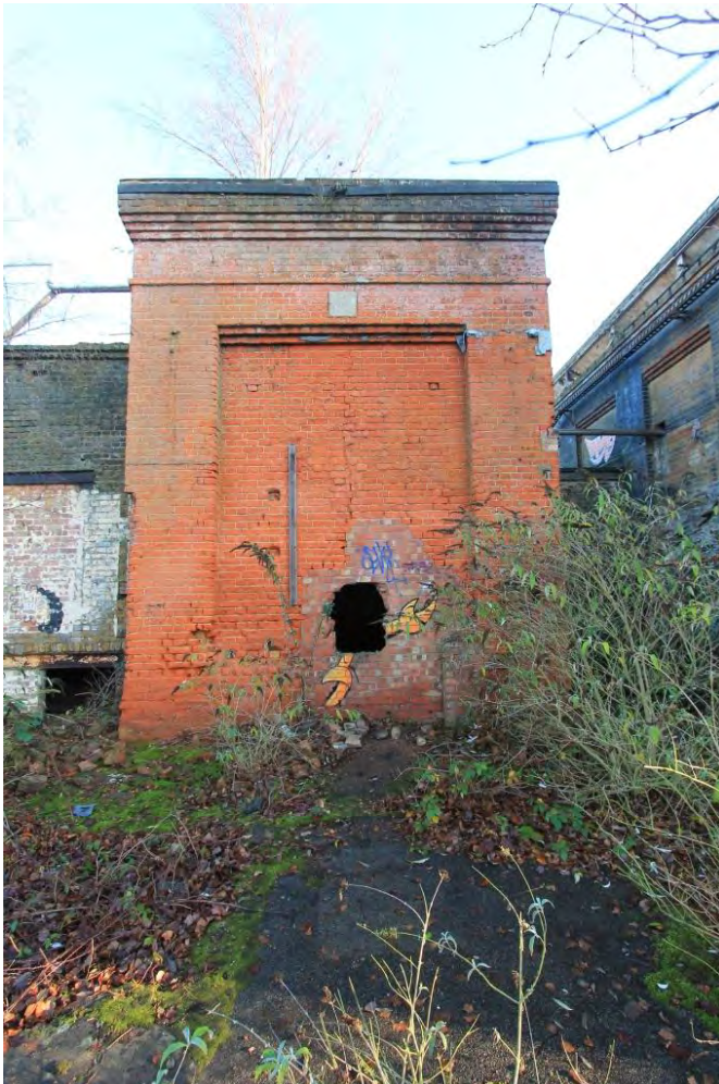
Plate 56: Building 3, detail of stack base
