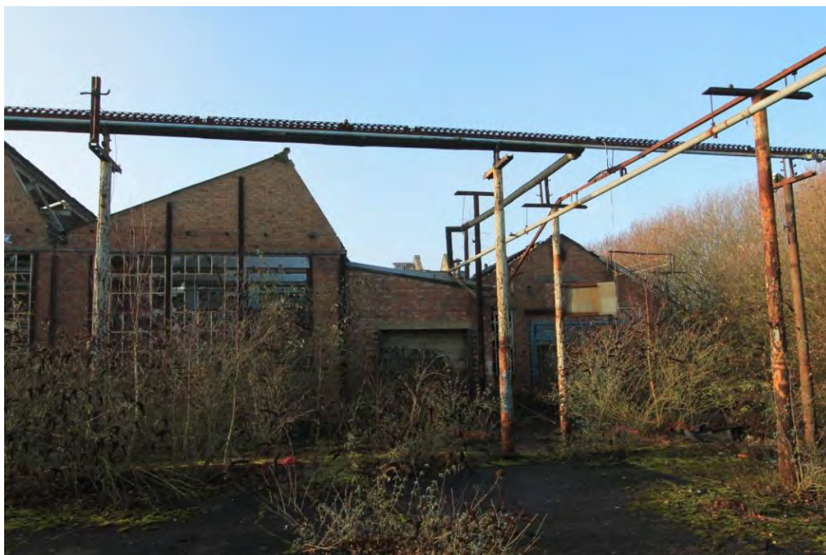
Plate 48: Building 2 as viewed from north-east
