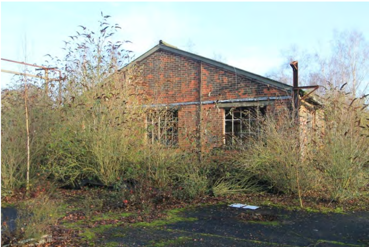
Plate 82: Building 14, viewed from south-west
