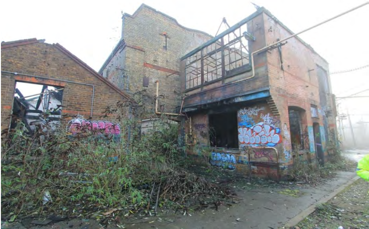
Plate 45: Building 2 as viewed from north-west
