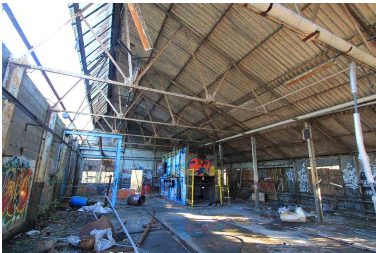
Plate 70: Building 9, interior view
