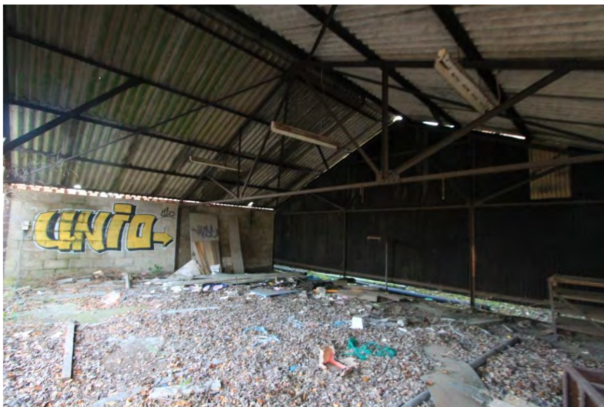
Plate 88: Building 15, interior view
