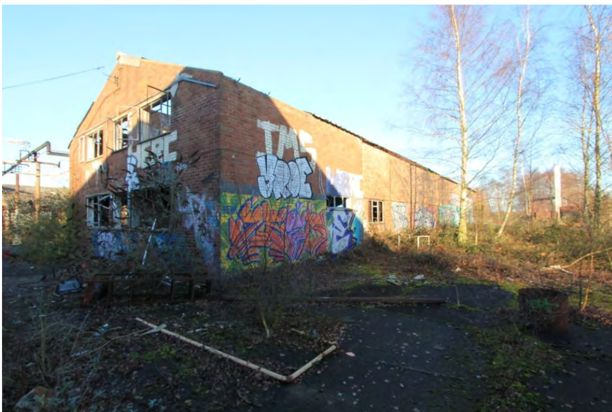
Plate 78: Building 13, viewed from south-west
