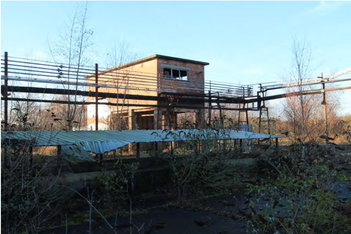
Plate 65: Building 7, viewed from south-west
