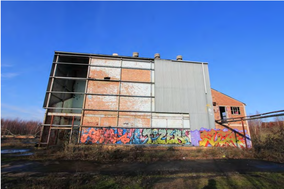
Plate 61: Building 6, viewed from south
