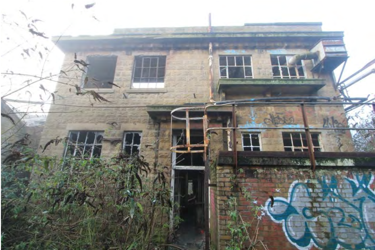
Plate 39: Building 1, north-east facing elevation
