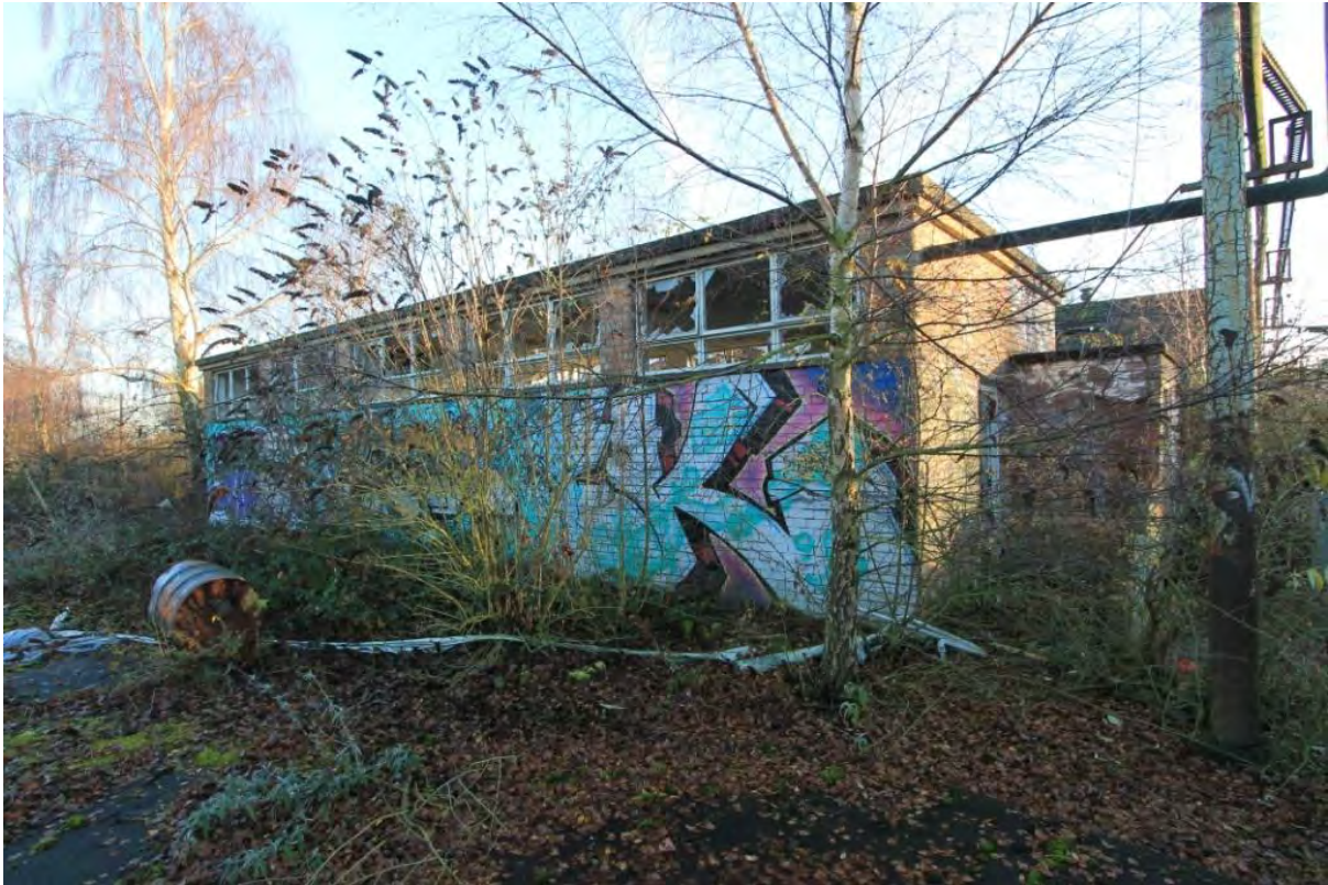
Plate 91: Building 17, viewed from north
