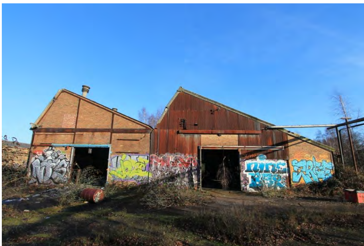
Plate 68: Building 9, viewed from south-west
