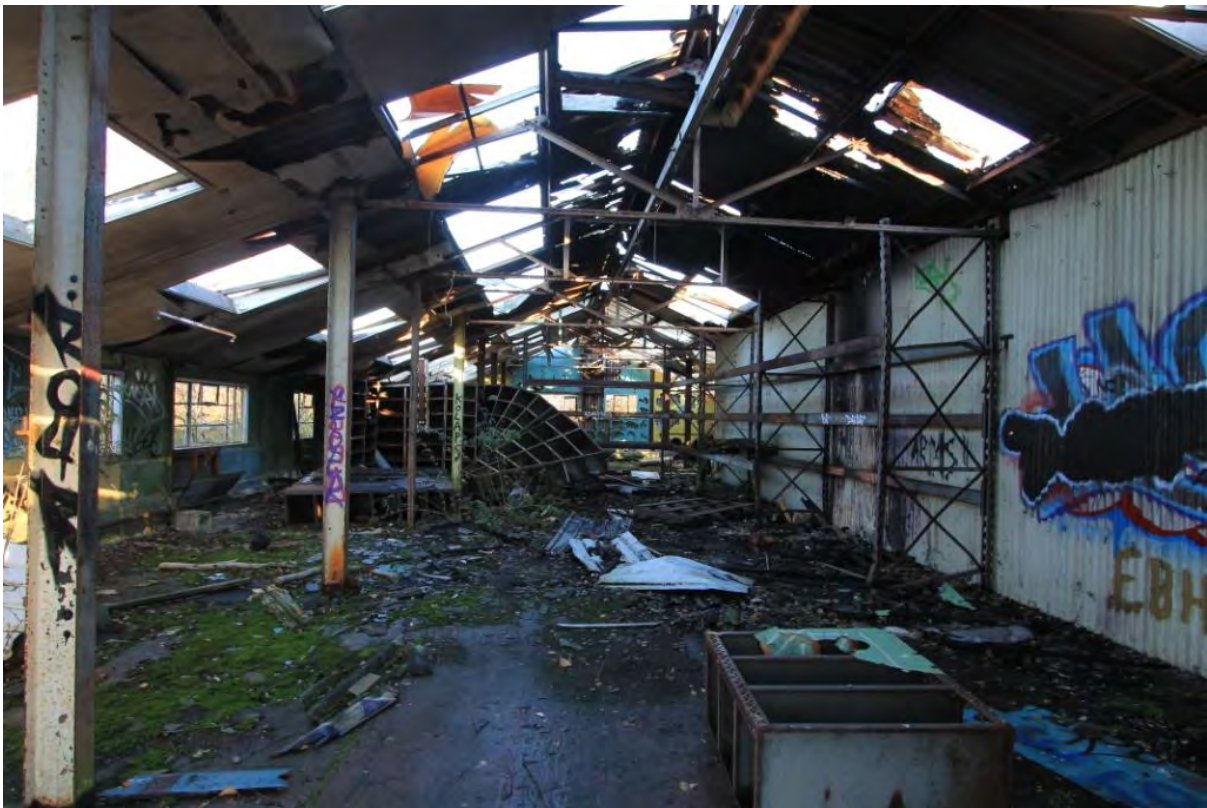
Plate 90: Building 16 interior view
