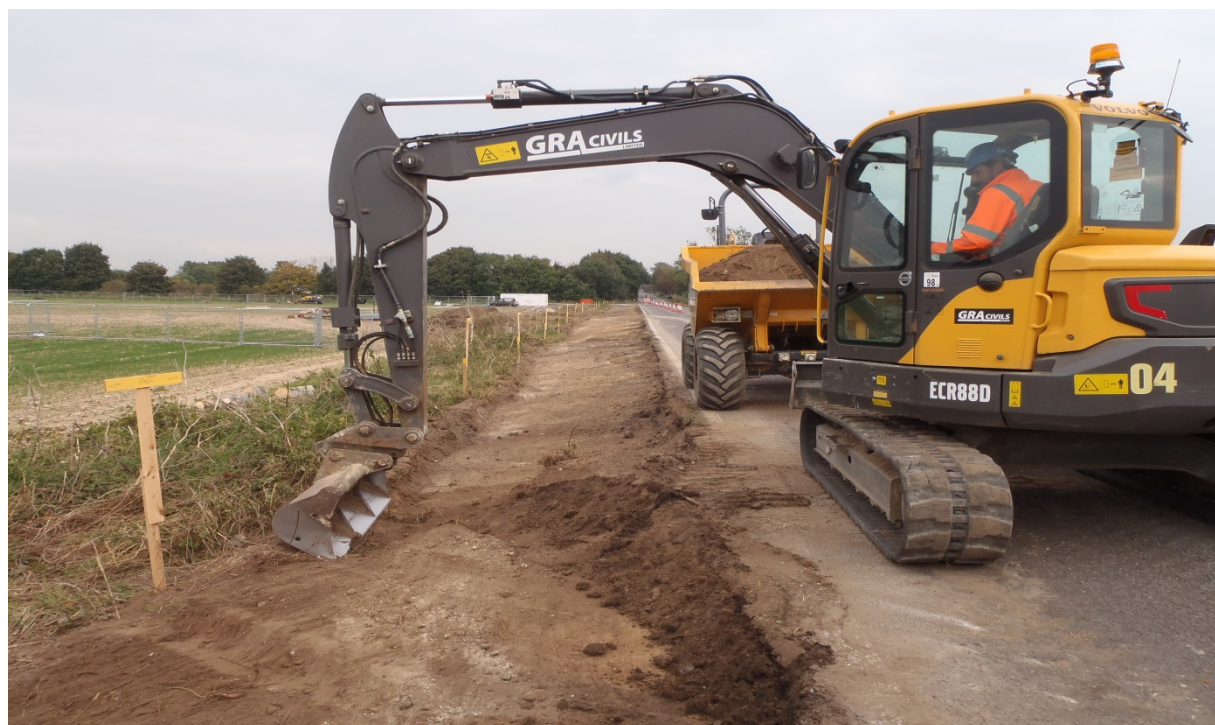
Plate 2: Edge of road stripping
