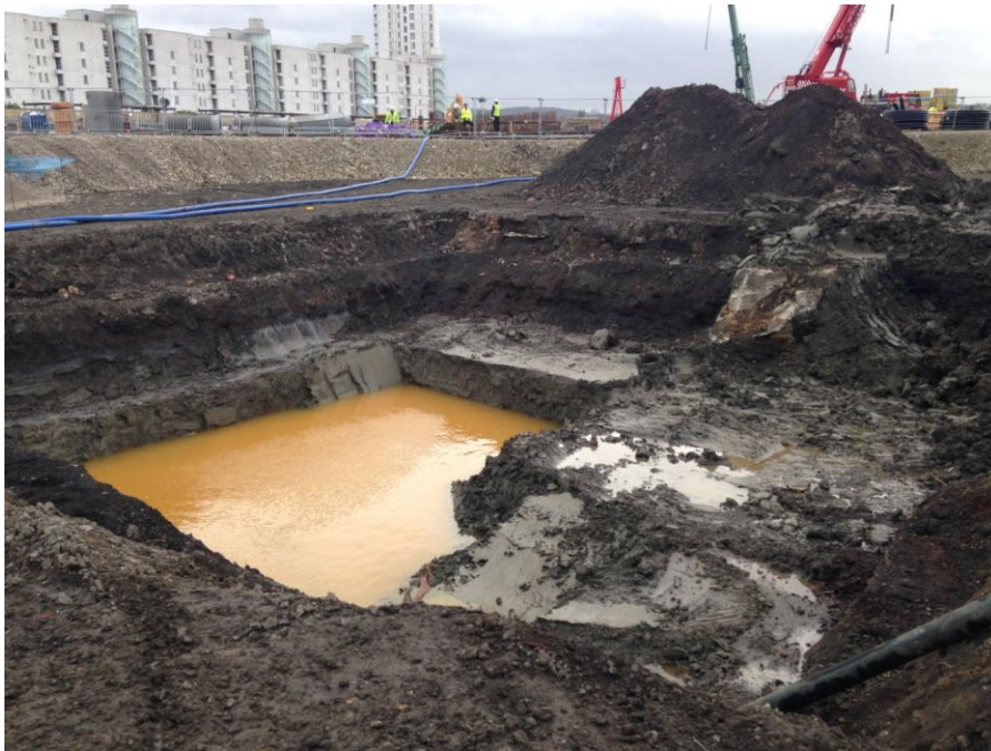
Plate 1: Trench 1 under excavation, looking south-east
