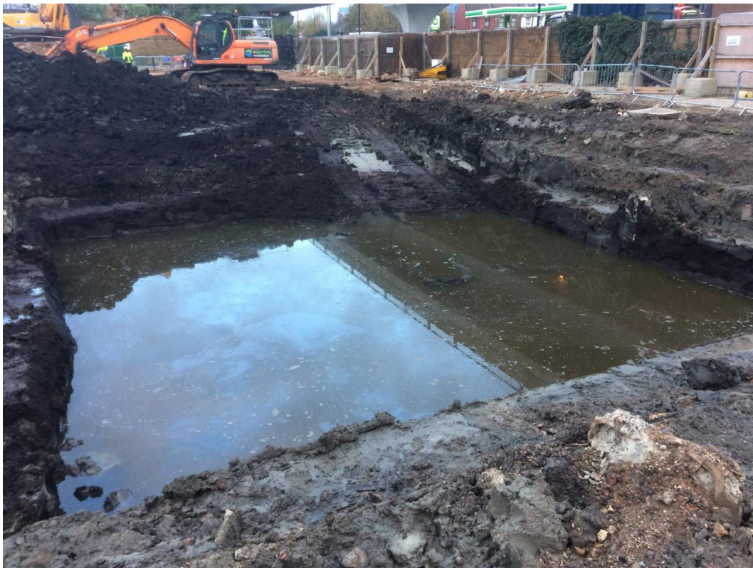
Plate 6: Trench 3 after full excavation, photograph looks north northwest.
