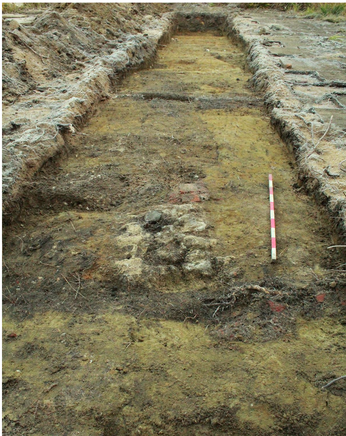
Plate 8: General view of Trench 8 looking north with flint foundation [5] (1m scale) in the foreground.
