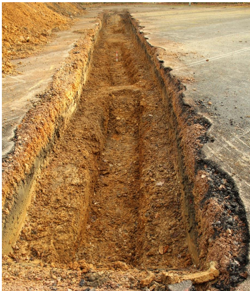
Plate 3: General view of Trench 2, looking SE
