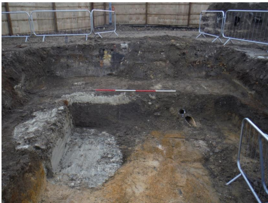
Plate 8: Trench 5, view south showing Section No. 15
