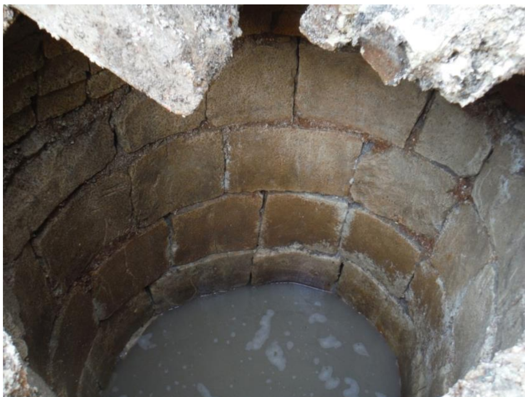
Plate 6: Trench 3, view east showing detail of Clunch Lining of Well [154]
