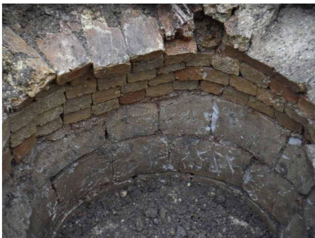
Plate 12: Trench 6 detail of Clunch Lining [121] and Brick 'Dome' [122]
