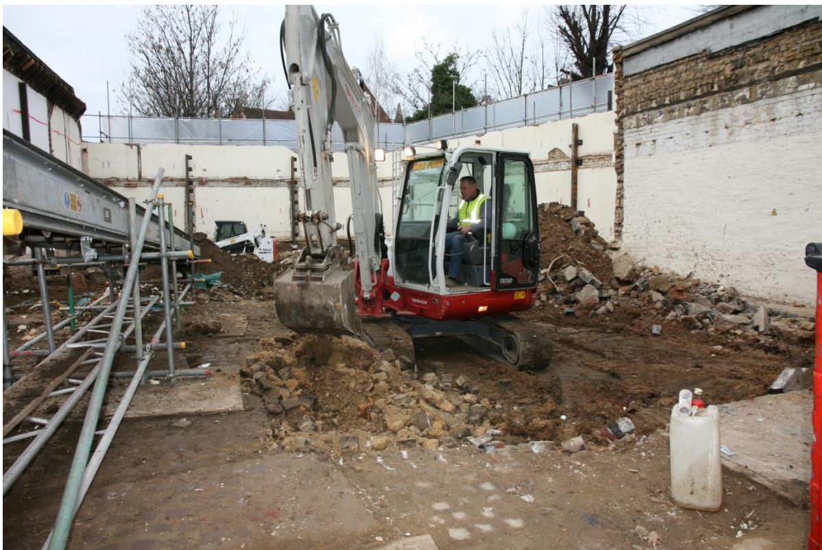
Plate 5: Excavation of Trench 6, looking north-west (BAM16 D2 011)
