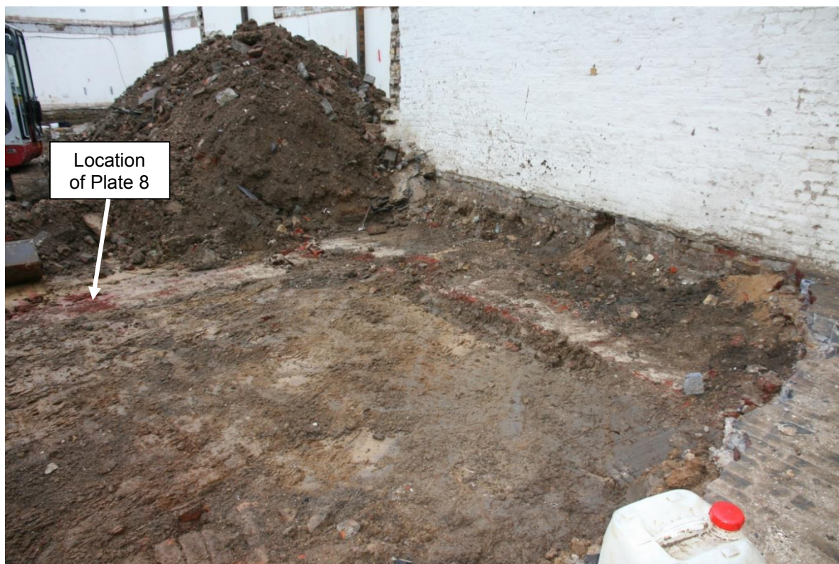
Plate 7: Nineteenth century L-shaped brick wall foundation [17] Trench 6, looking north-west (BAM16 D2 024)
