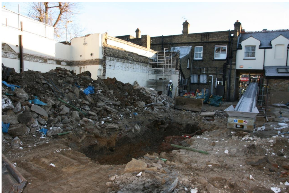
Plate 1: Excavation of Trench 5, looking north-east (BAM16 D2 004)
