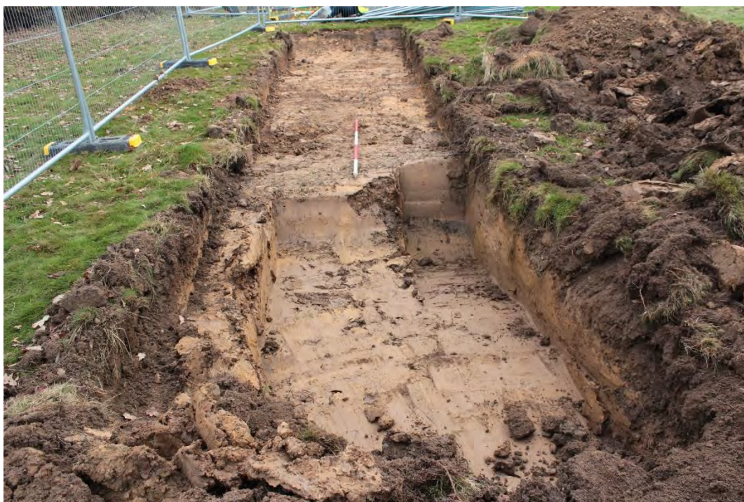
Plate 5: Trench 3 looking south showing natural clay [49], 2m scale
