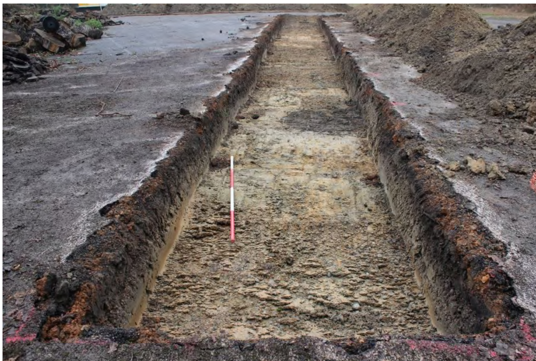
Plate 23: Trench 12 looking north showing contaminated pit [165] and natural clayey gravel [167], 2m scale
