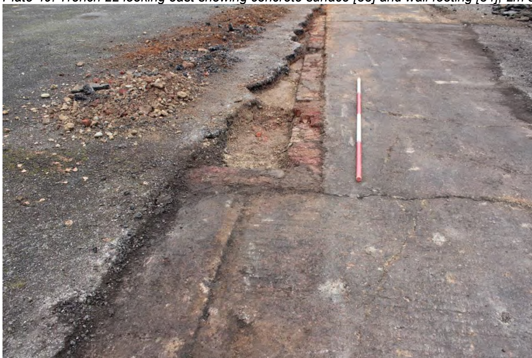
Plate 50: Trench 22 looking west showing wall footing [34] and concrete surfaces [33] and [35], 2m scale
