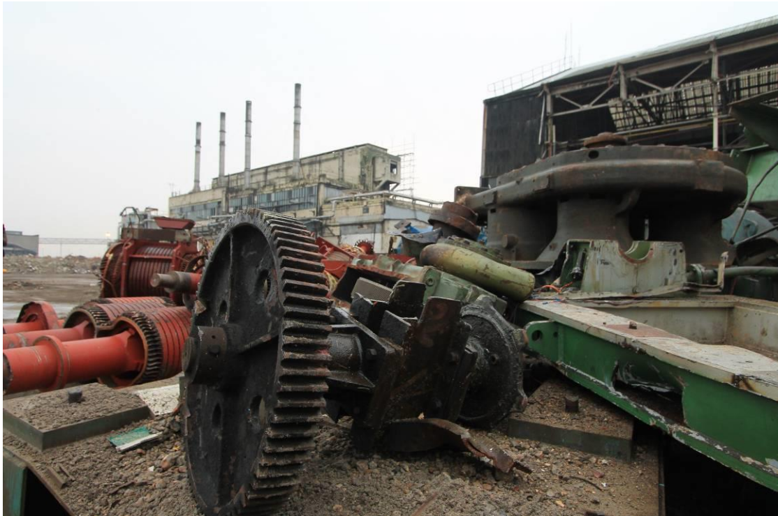
Plate 17 Examples of apparatus removed from demolished buildings
