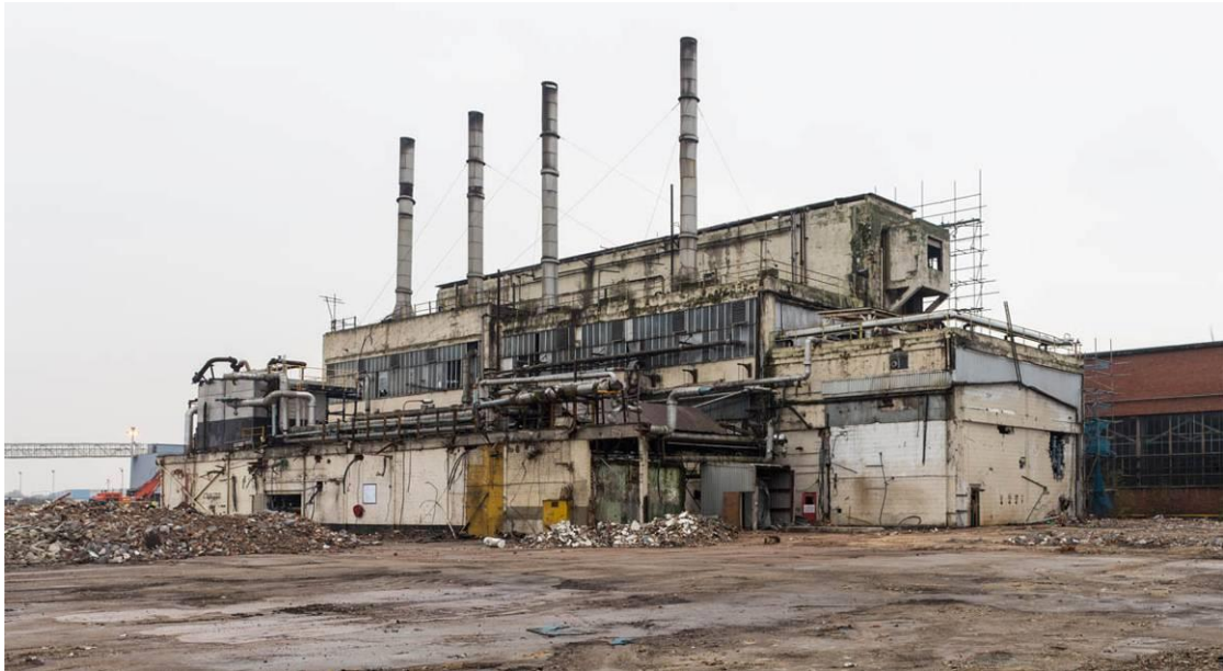
Plate 3 Northern Elevation looking south-east
