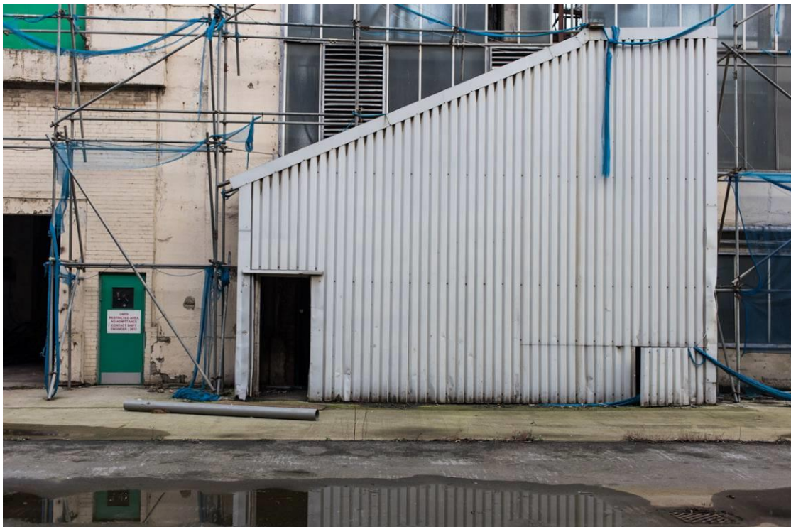
Plate 12 Southern Elevation, modern external stairwell
