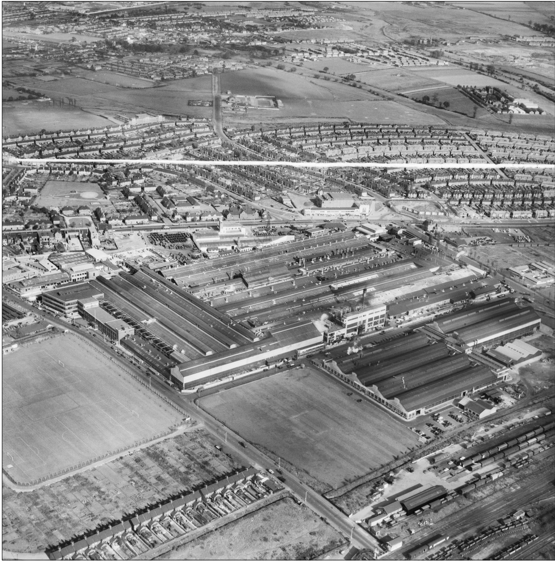
General View of Site
