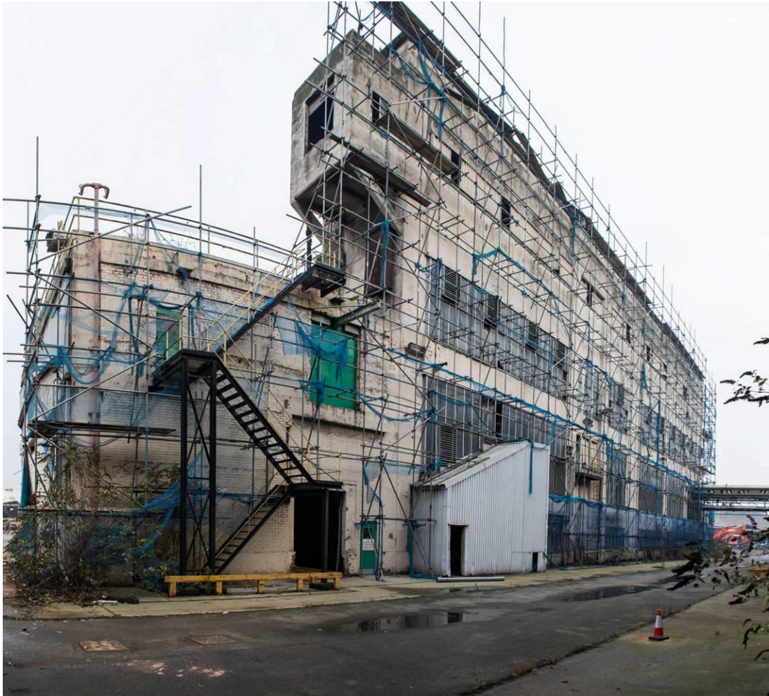
Plate 7 Southern Elevation looking north-east
