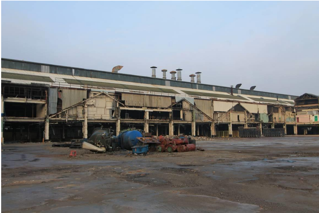
Plate 19 Adjacent production buildings during demolition
