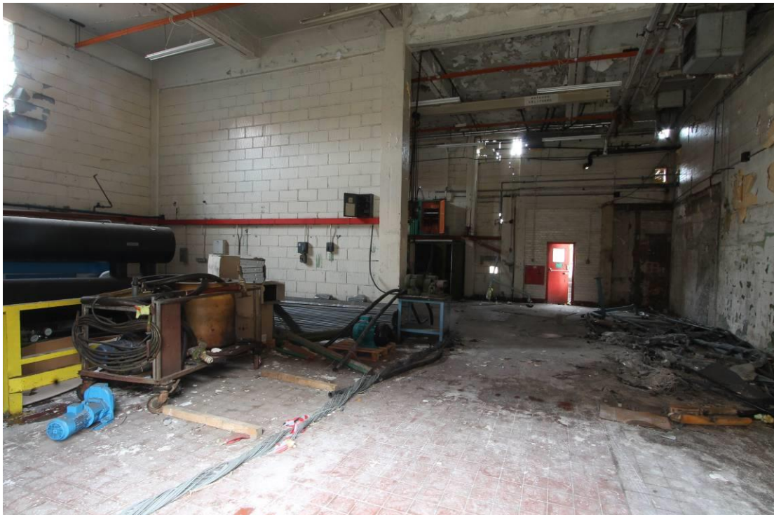
Plate 16 Internal view, western bays (former compressor house)
