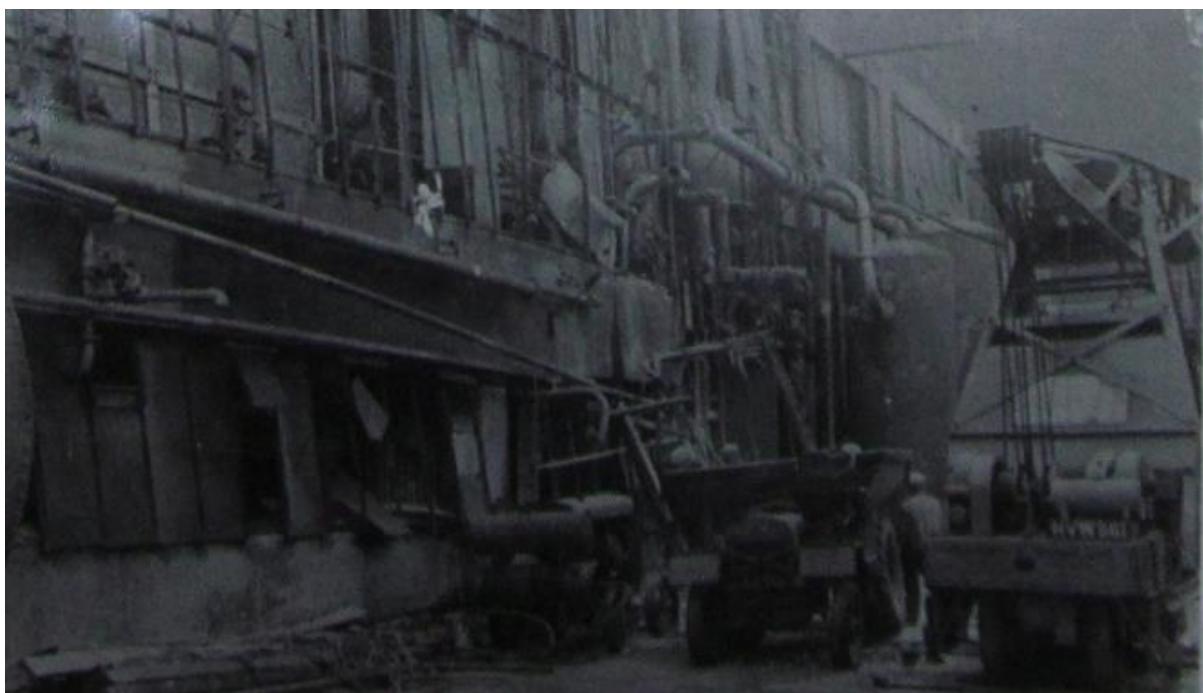
Plate C: Air raid damage at Briggs Motor Bodies Ltd, September 1940
