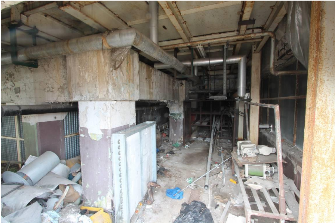
Plate 15 Internal views from eastern end wall
