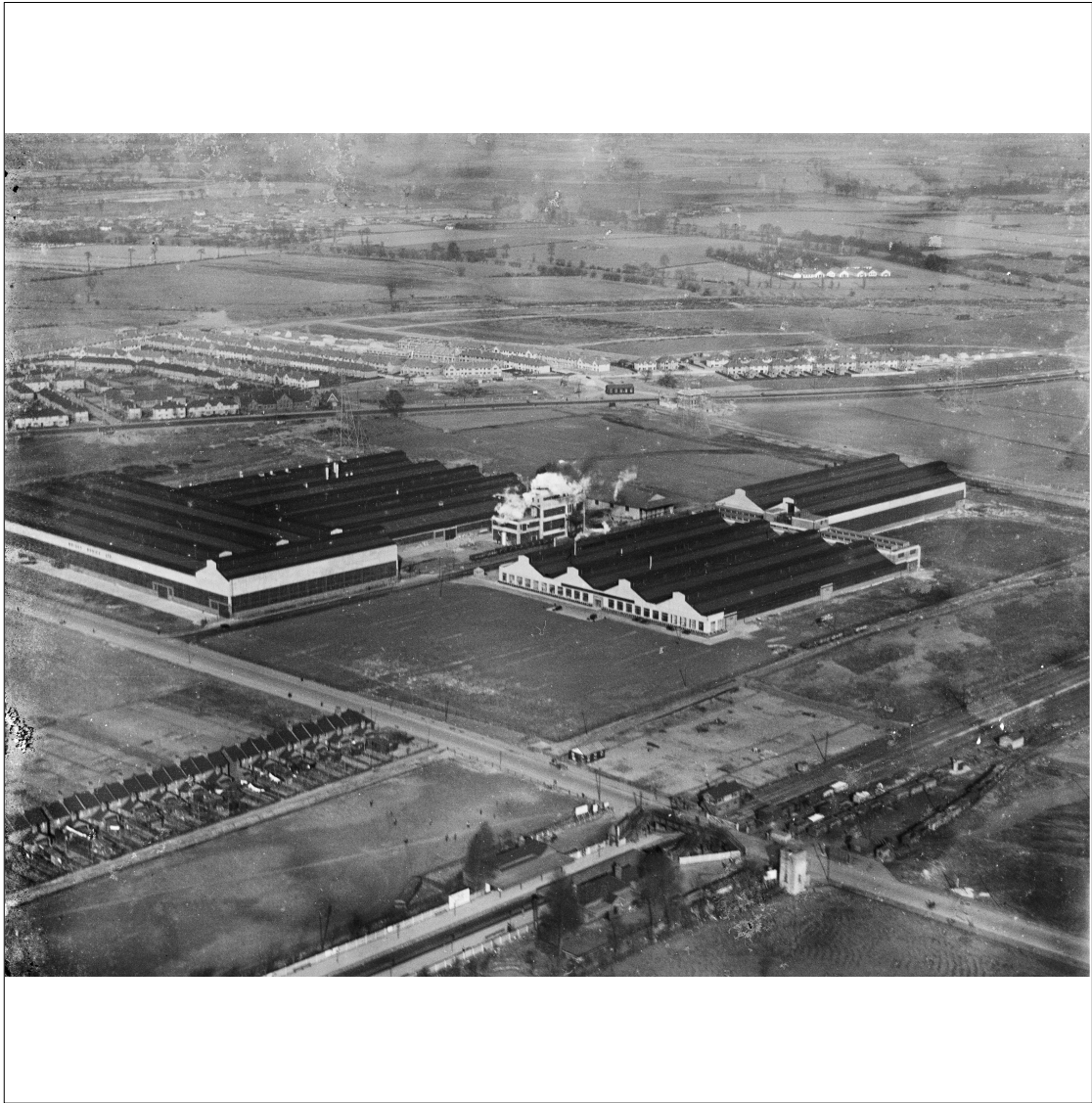
General View of Site
