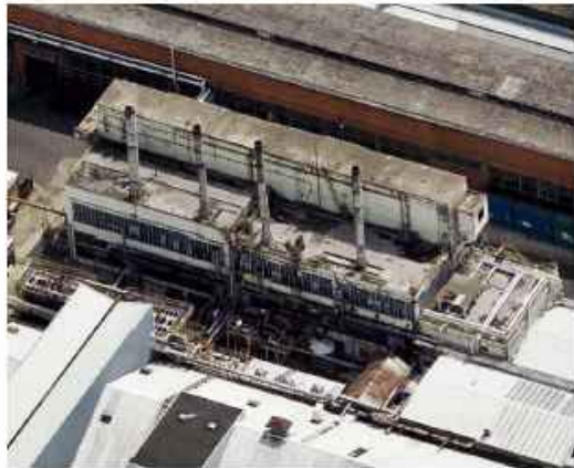
Detail of Former Compressor & Boiler Houses, Looking South
