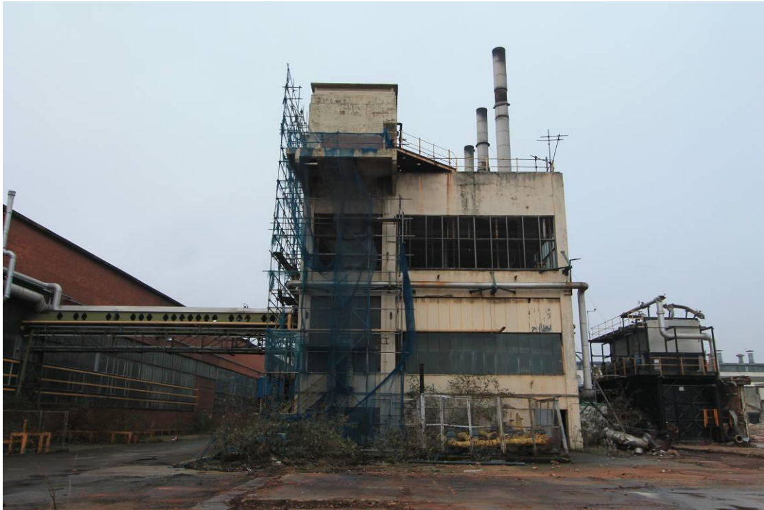
Plate 5 Eastern End Elevation looking west
