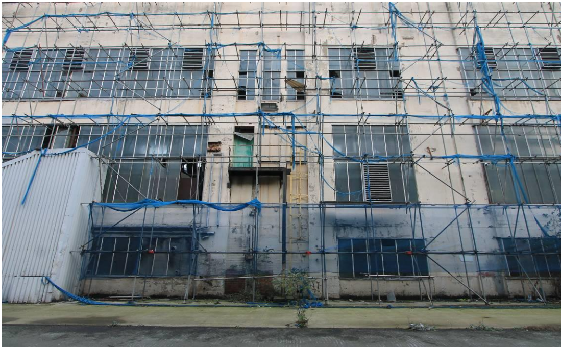
Plate 8 Detail of Fenestration, Southern Elevation
