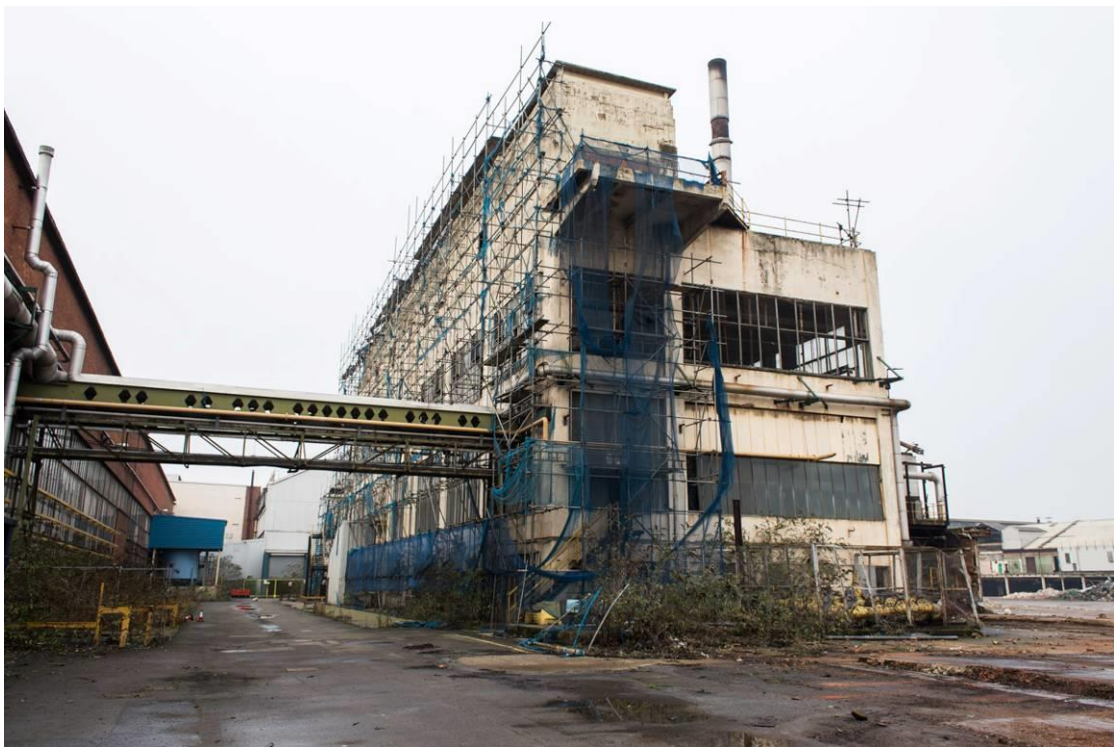
Plate 6 Eastern and Southern Elevations looking west
