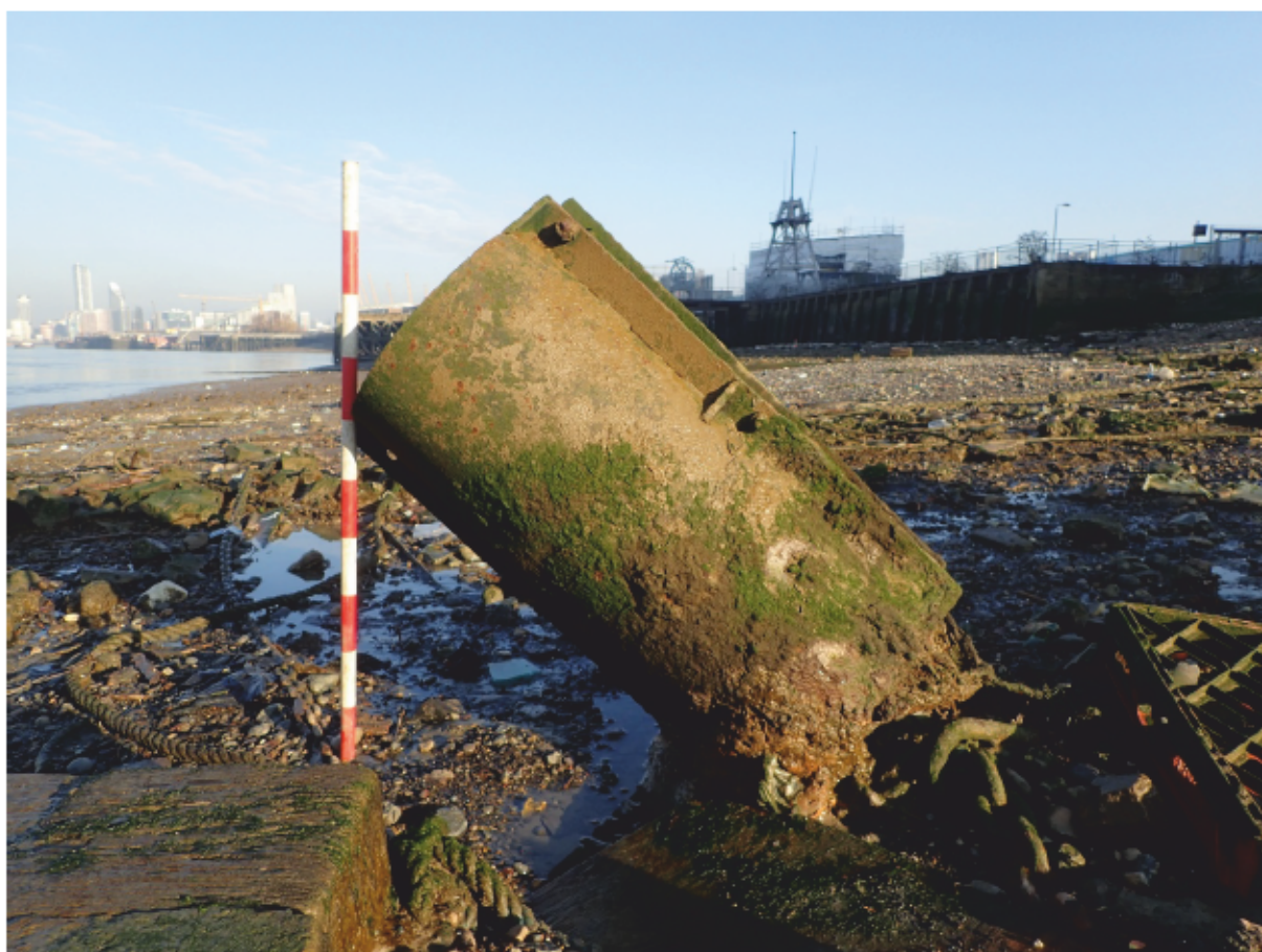
Plate 8: Mooring post [14] with metal cylinder or sheath, view to the north, scale 1m
