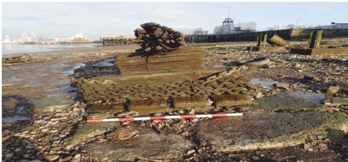
Plate 7: Barge-bed structure with horizontal beam [16] on three pillars [17] , [18] & [19], view to the north, scale 1m
