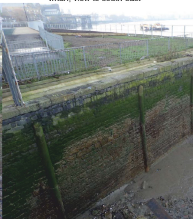
Plate 36: Granite Wharf, view to south-west
