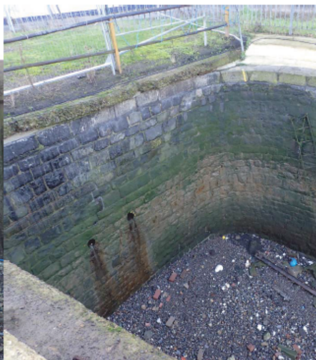
Plate 34: Southern limit, boundary of granite wharf, view to south-east
