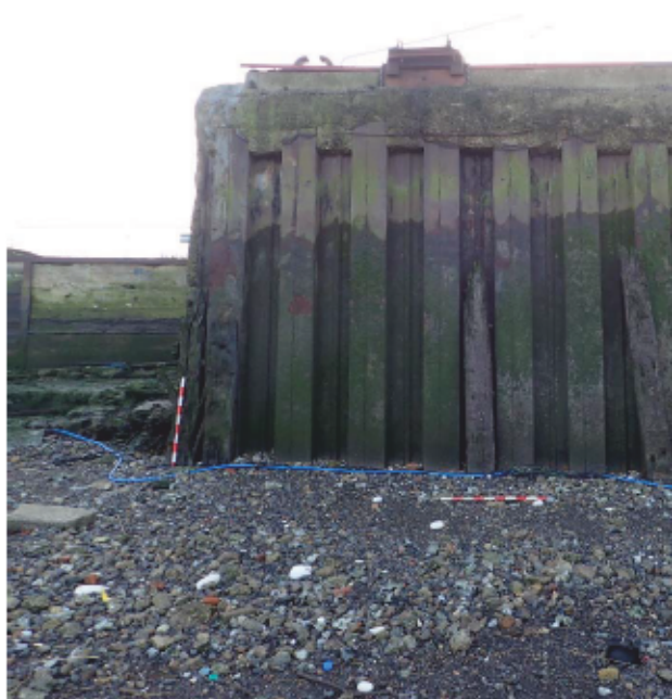
Plate 33: River wall shuttering, (Wharf 1) view to east, scale 1m
