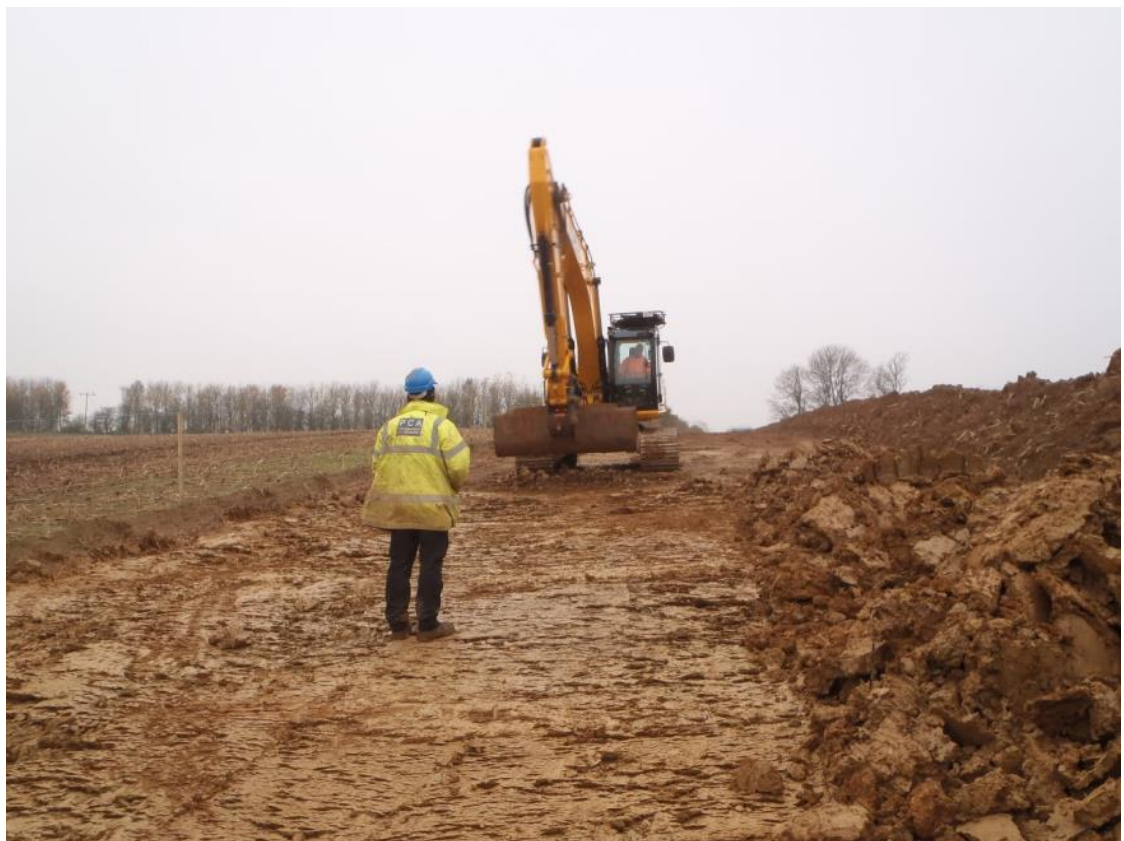
Plate 1: South-west view of machine stripping of Area 4
