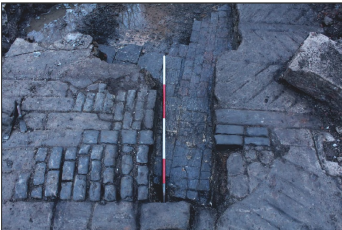
Plate 37: Dipping room floor surface [1261] below 20th century floor surface Group 69: view south-east. 2m scale
