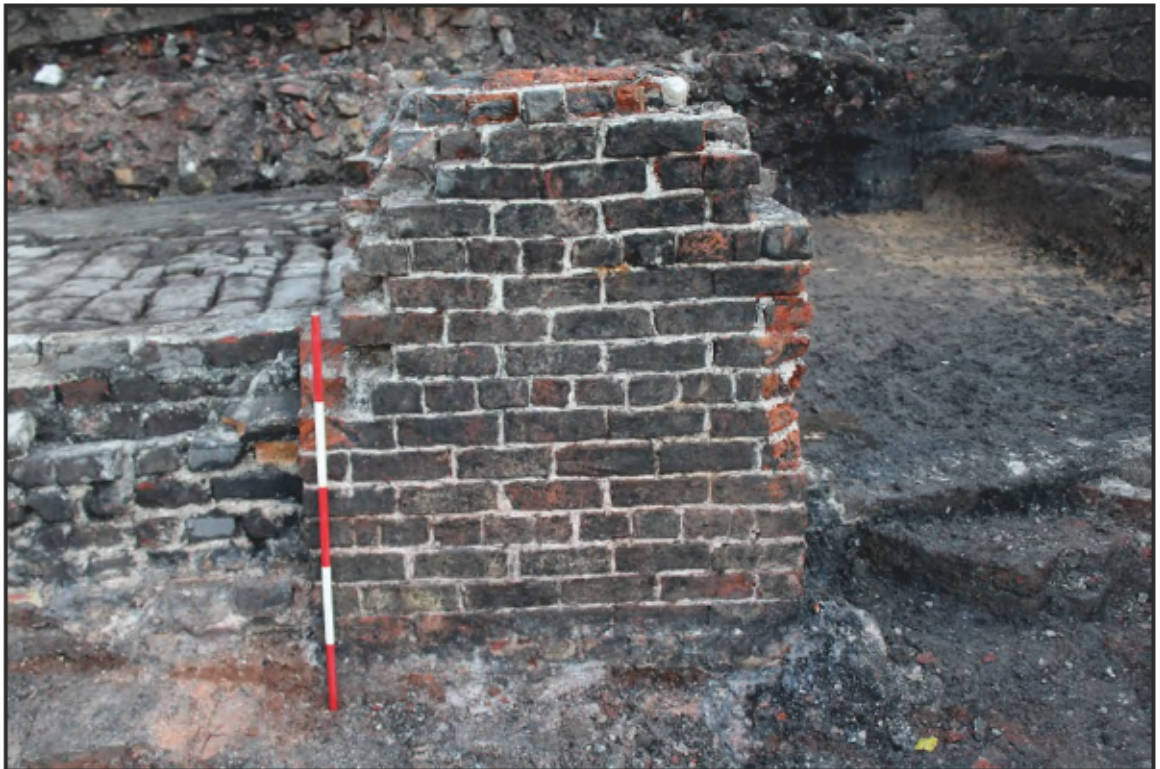
Plate 33: Wall [1005]: view south-east. 1m scale
