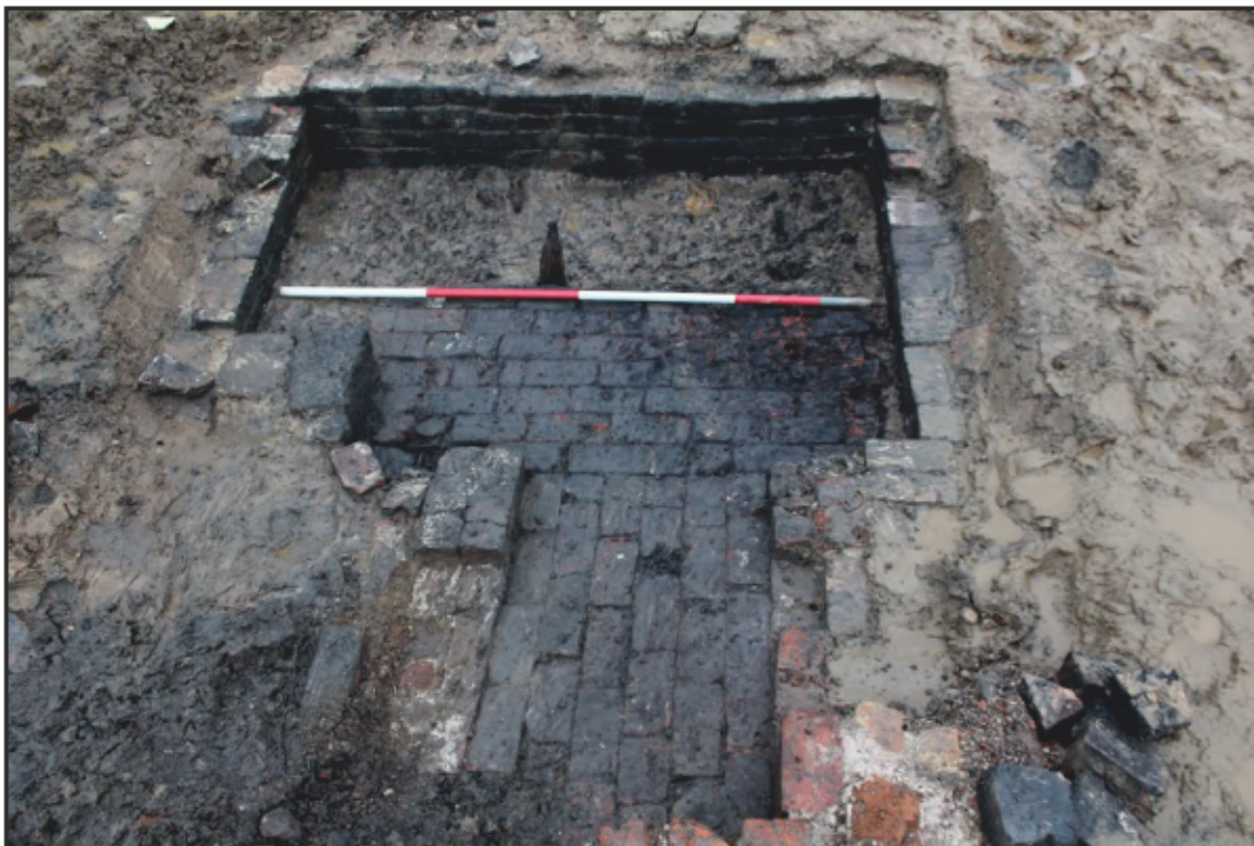
Plate 28: Coal store (Group 23): view south-east. 1m scale
