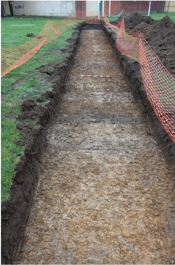
Plate 2: Trench 2 facing north
