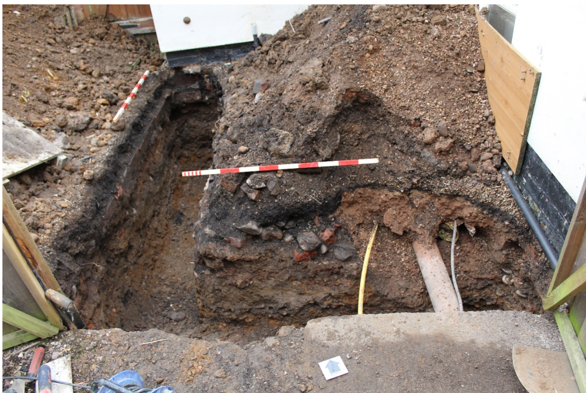
Plate 1: View facing north-northeast across house footings.
