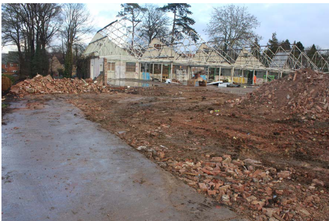
Plate 2: The eastern plot, view south-east
