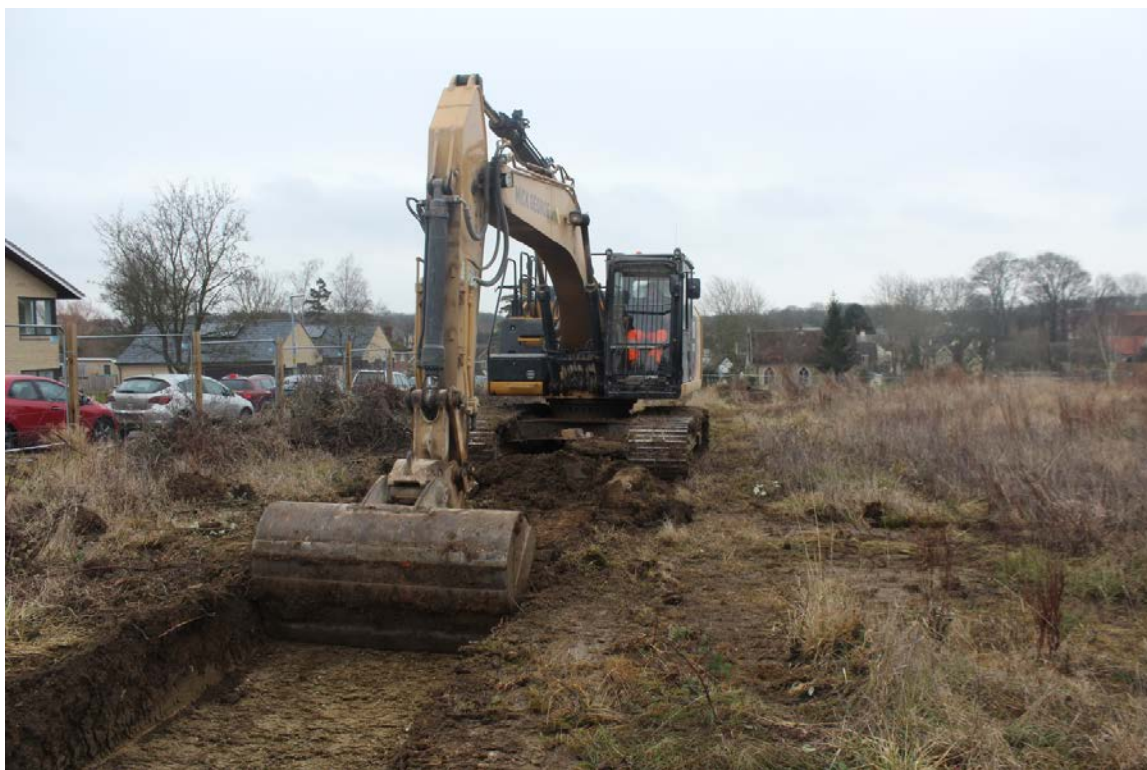
Plate 3: Machining the western plot, view north-east
