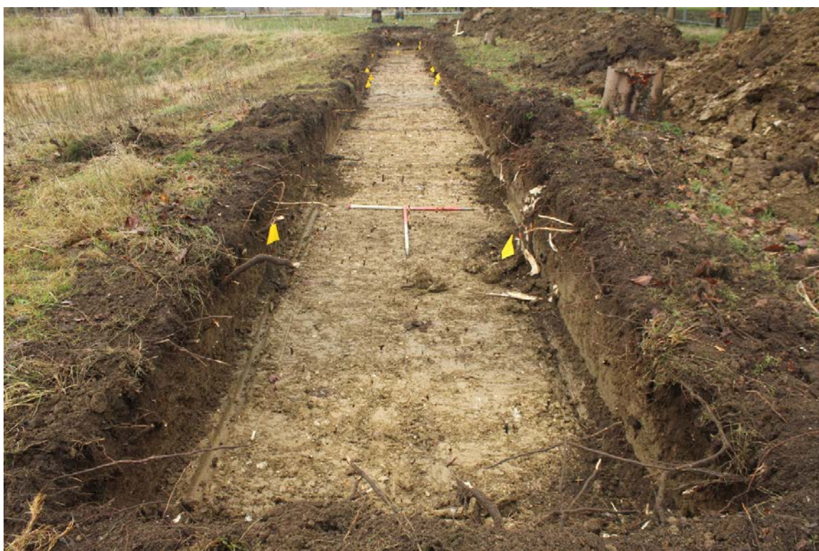
Plate 4: Trench 1 pre-excitation, view south-east
