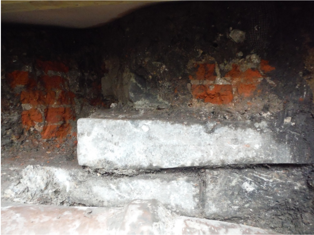
Plate 5: West facing view of detail of masonry of medieval wall [8]
