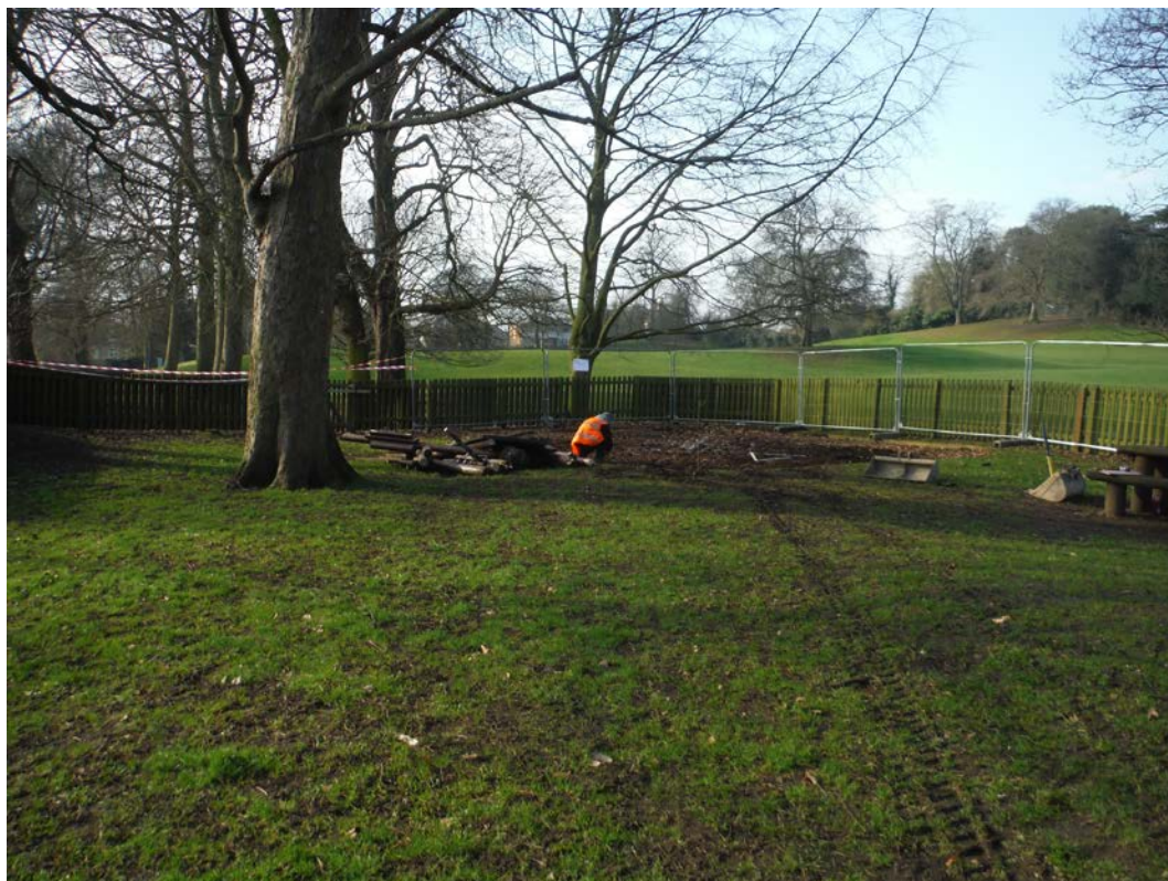
Plate 3: Area of Test Pits 11-20, view west
