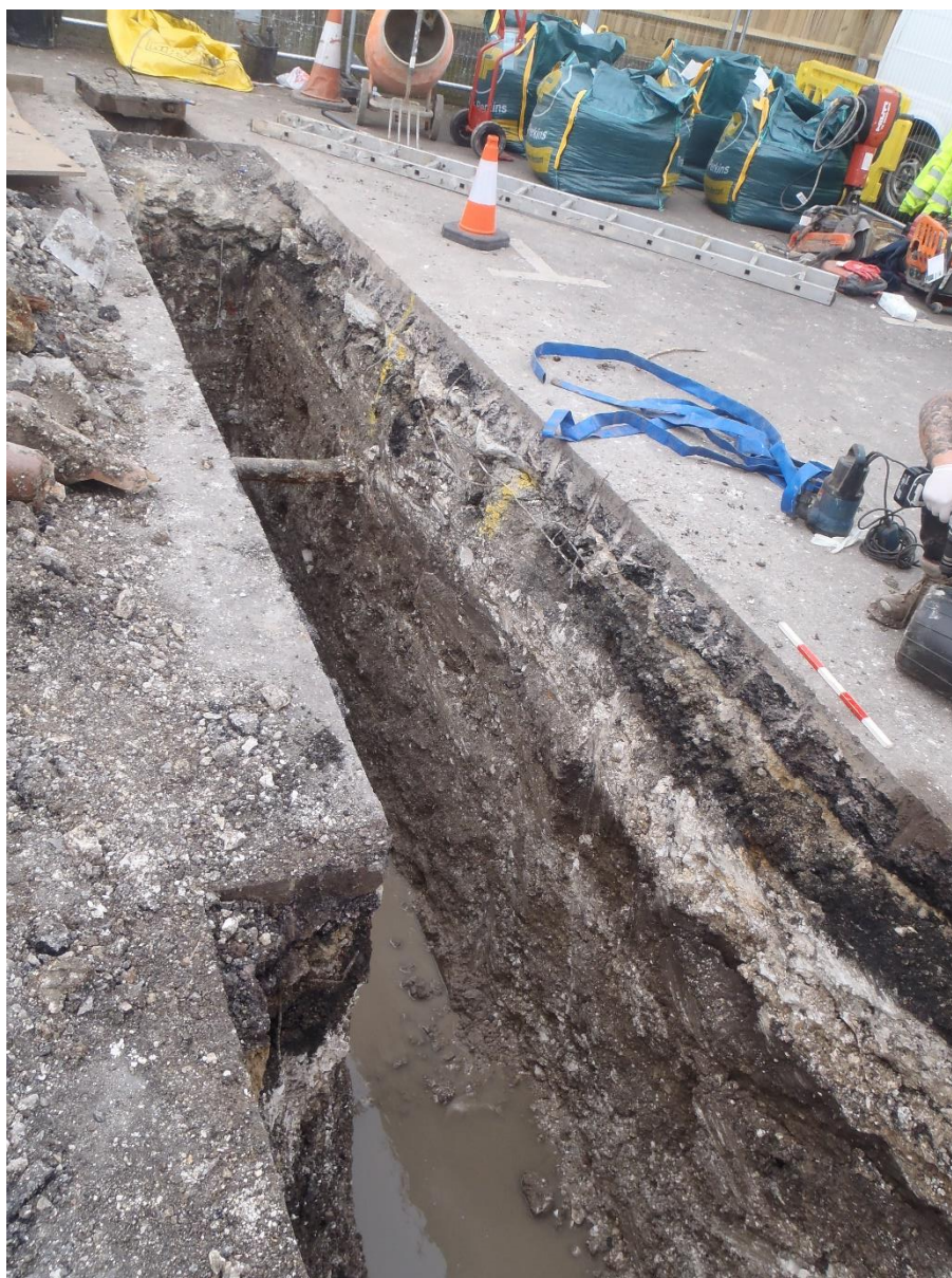
Plate 3 – Excavated trench, looking north west
