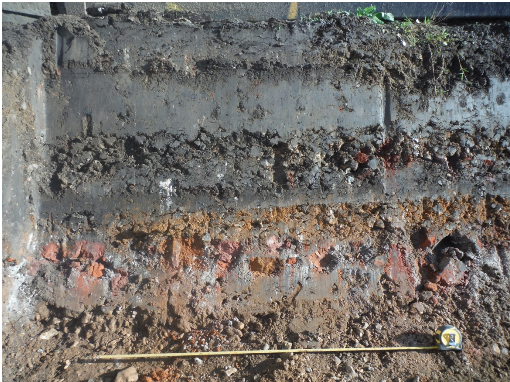
Plate 2: East facing section of ground reduction area. (1m scale).
