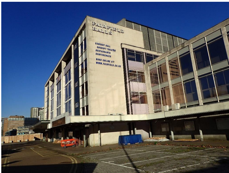
Plate 1: North Facing Photo of Fairfield Halls
