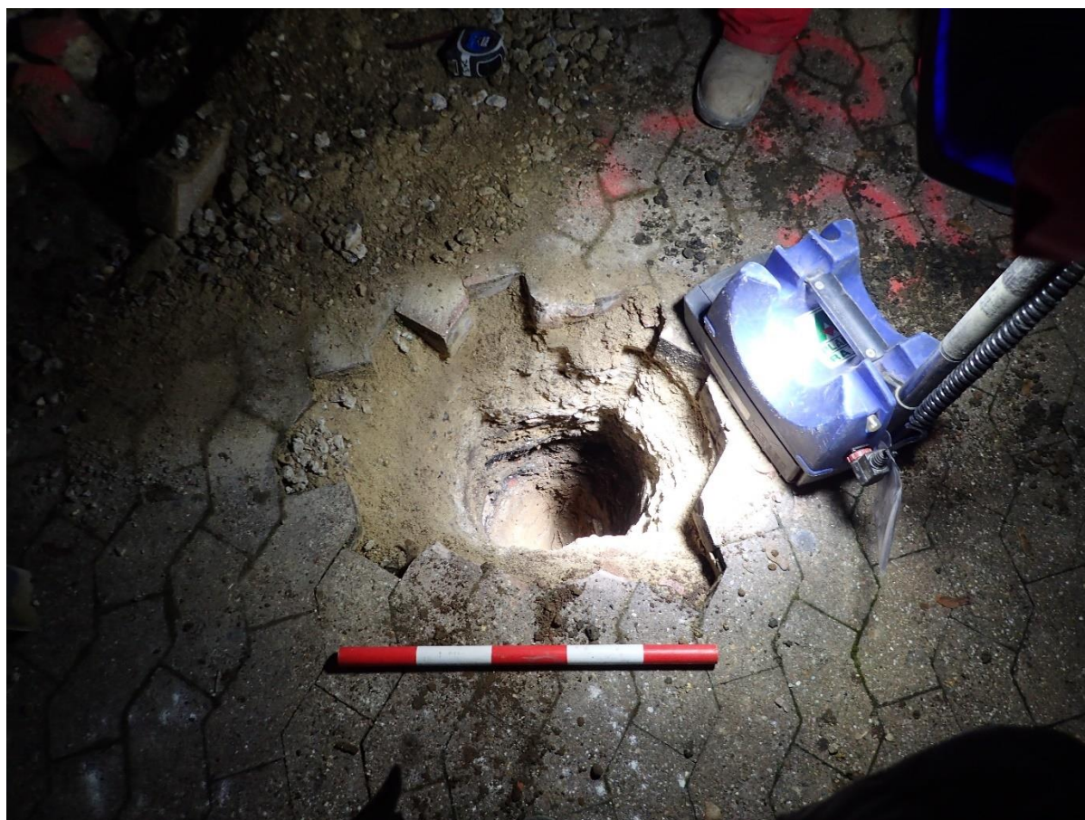
Plate 2: East Facing Photo of DCP01-01
