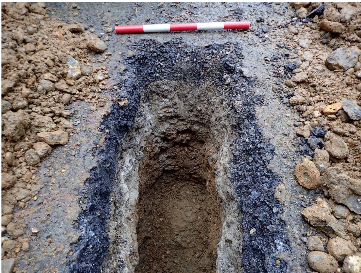
Plate 6: North Facing Photo of OP03-07 Showing Concrete Block
