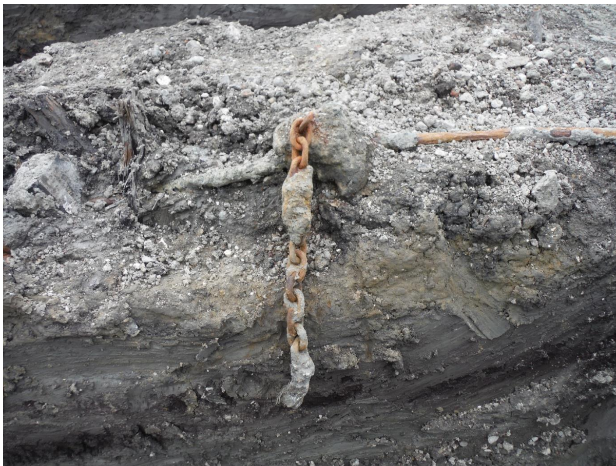
Plate 4: South facing view of detail of chain on canal tie back [542].
