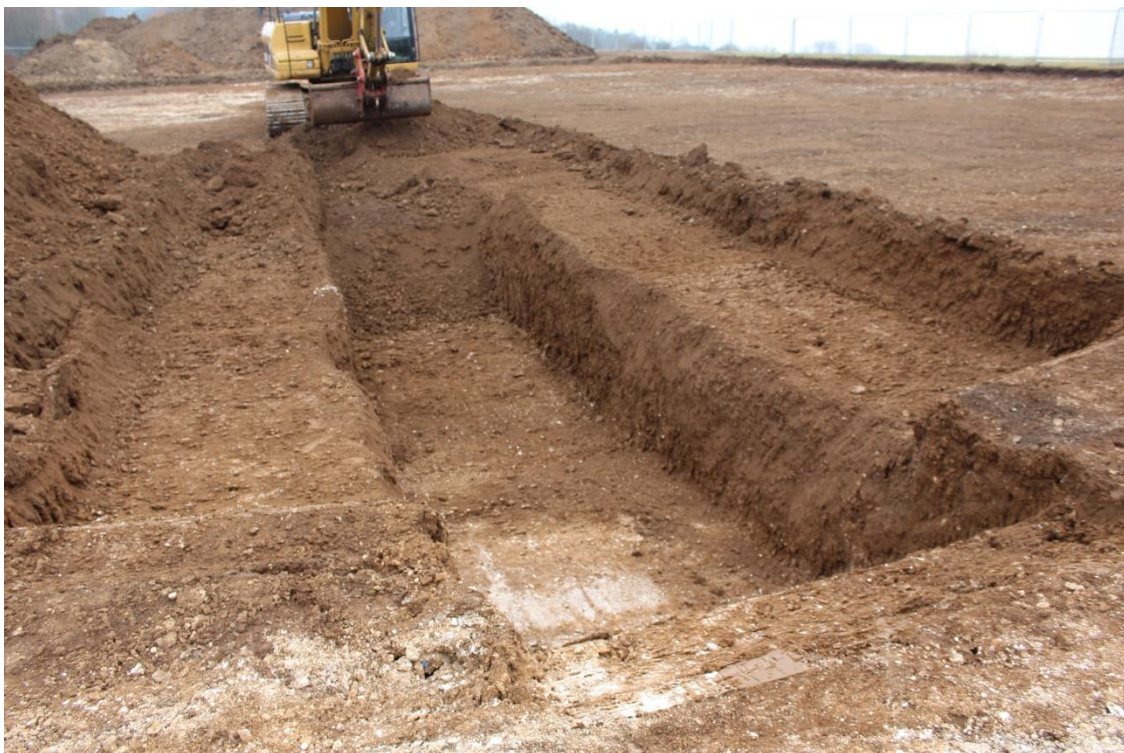
Plate 10: Machine Excavating [217] View North East
