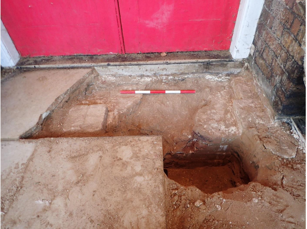
Plate 11: Service Trench side G, looking east, modern truncation through foundation wall of The Great Pagoda, 1m scale
