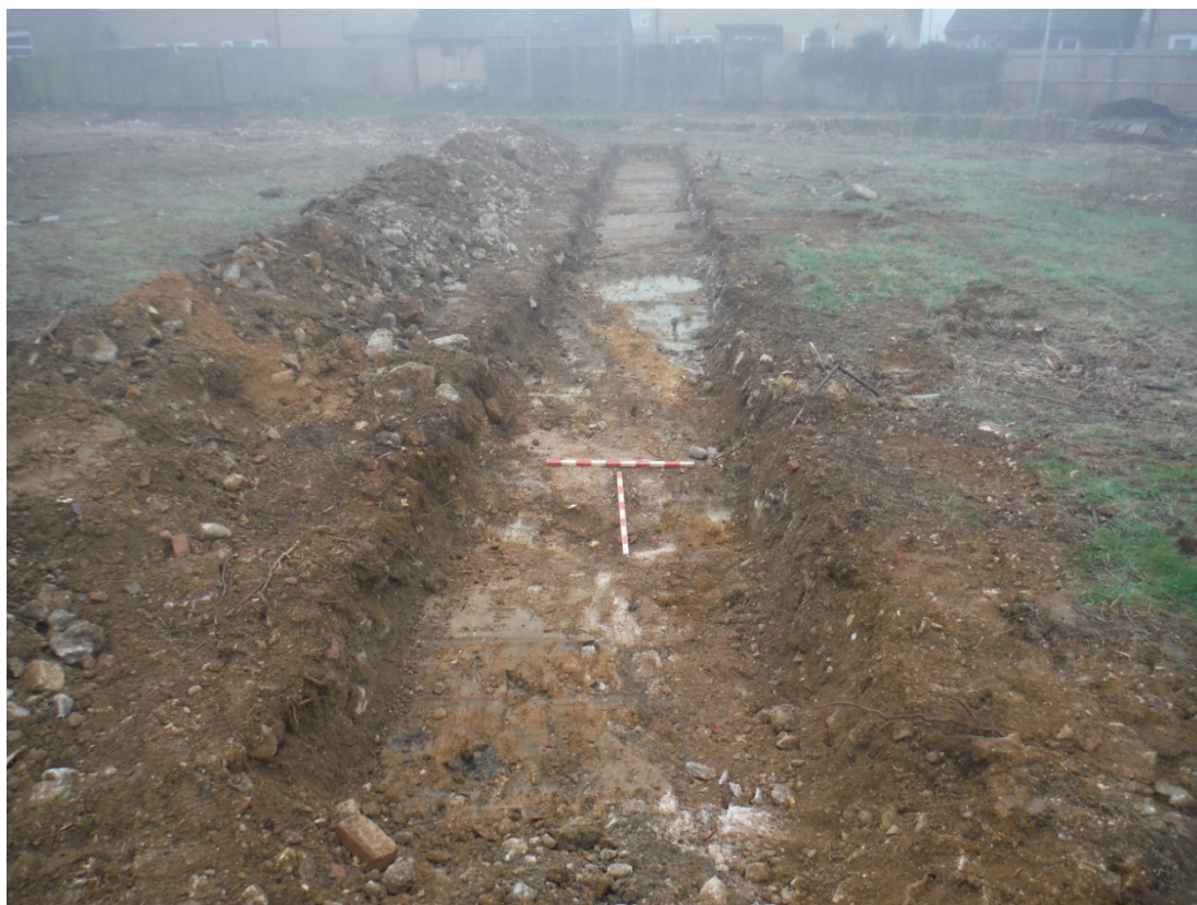
Plate 3: Trench 2, view south-west
