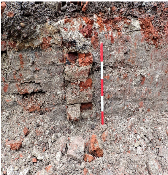
Plate 8: View to south-west. Internal wall [59] (centre) has been cut into the exterior north wall [51] (scale = 0.5m).
