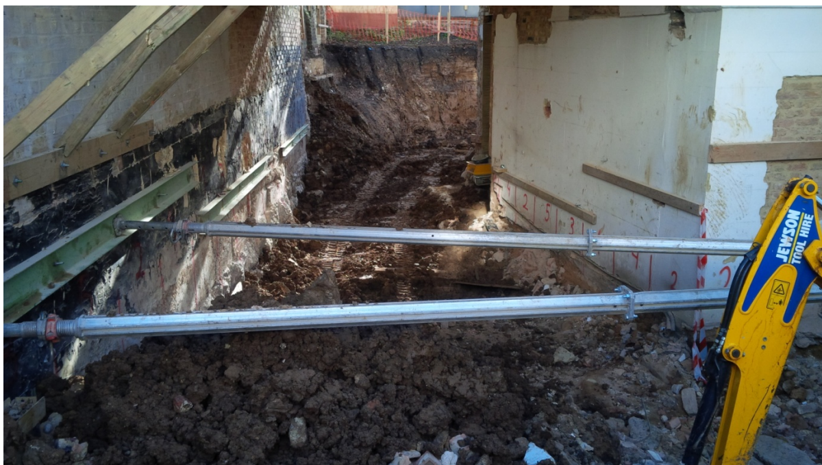
Plate 3: Ground reduction of existing basement, facing east
