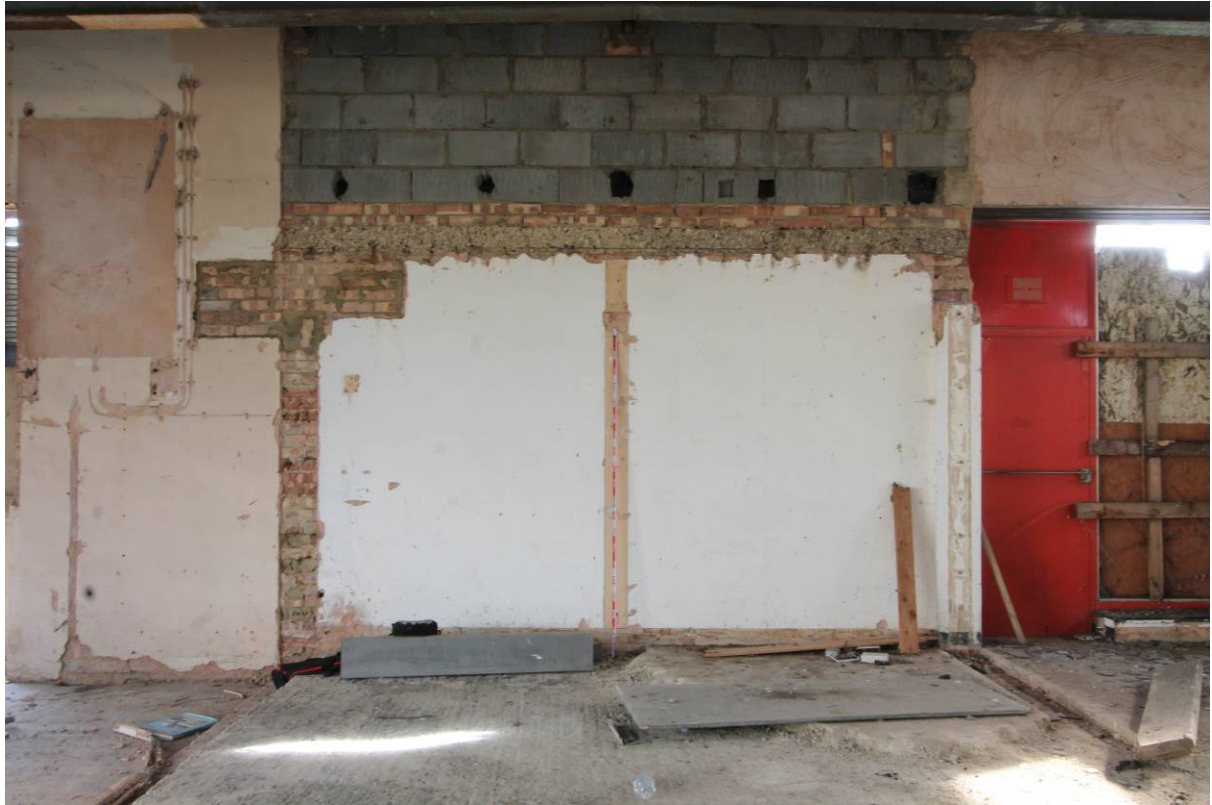
Plate 19 Isolated room with slab ceiling, looking east
