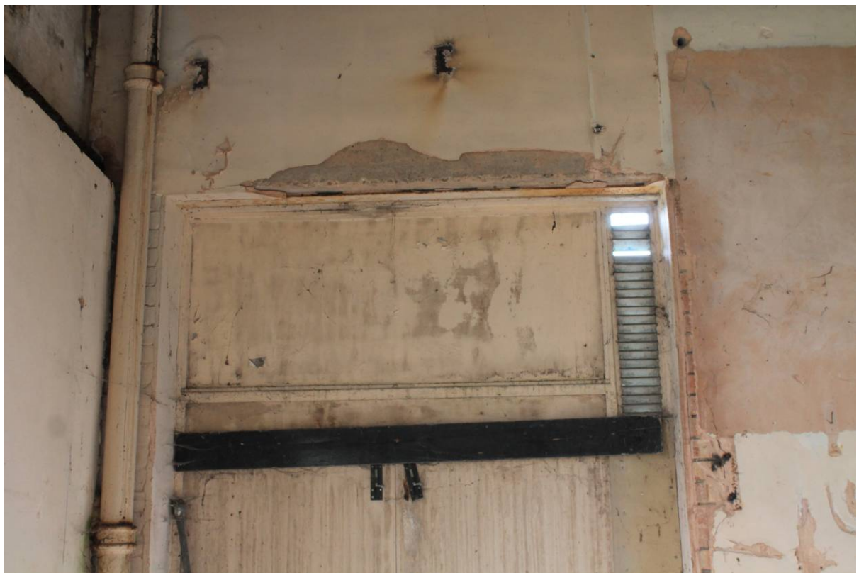
Plate 18 Door with blocked light and louvred vent, looking east
