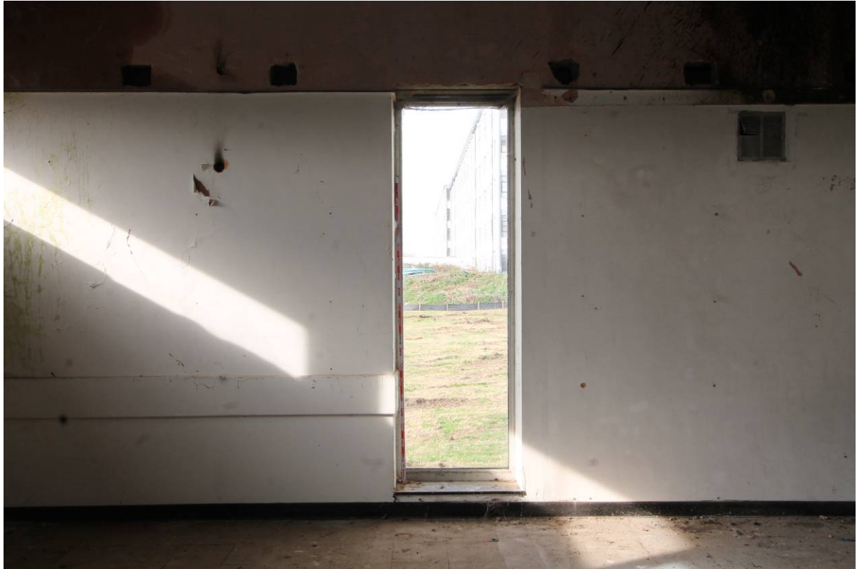
Plate 13 Detail of window, looking west
