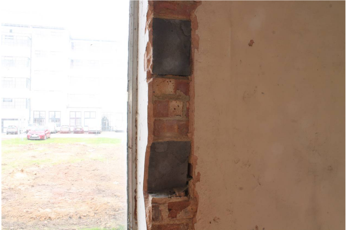
Plate 17 Fletton brick and blockwork elevation
