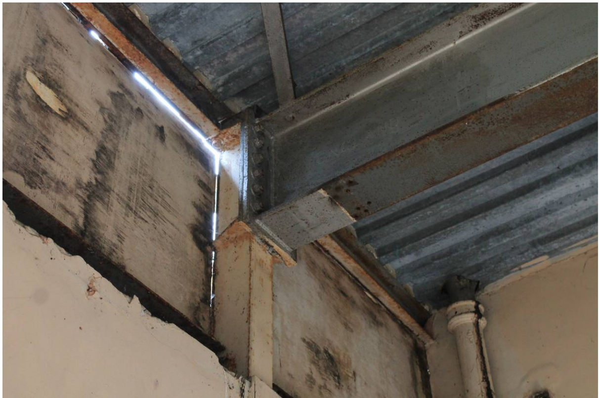
Plate 14 Detail of stanchion head and truss connection
