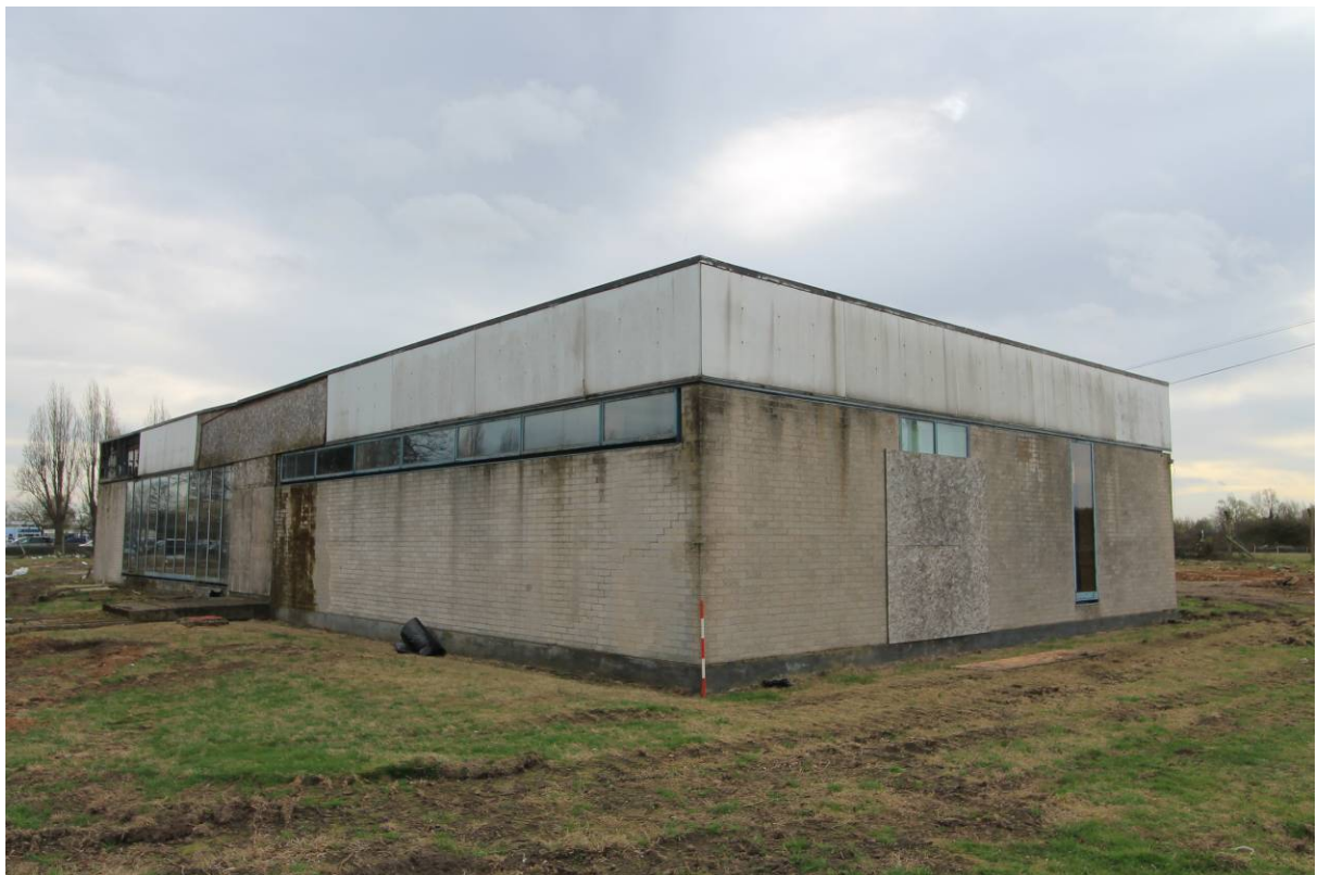
Plate 8 Computer Centre western elevation, looking south-east
