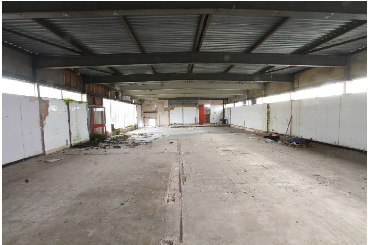
Plate 11 Internal view looking east
