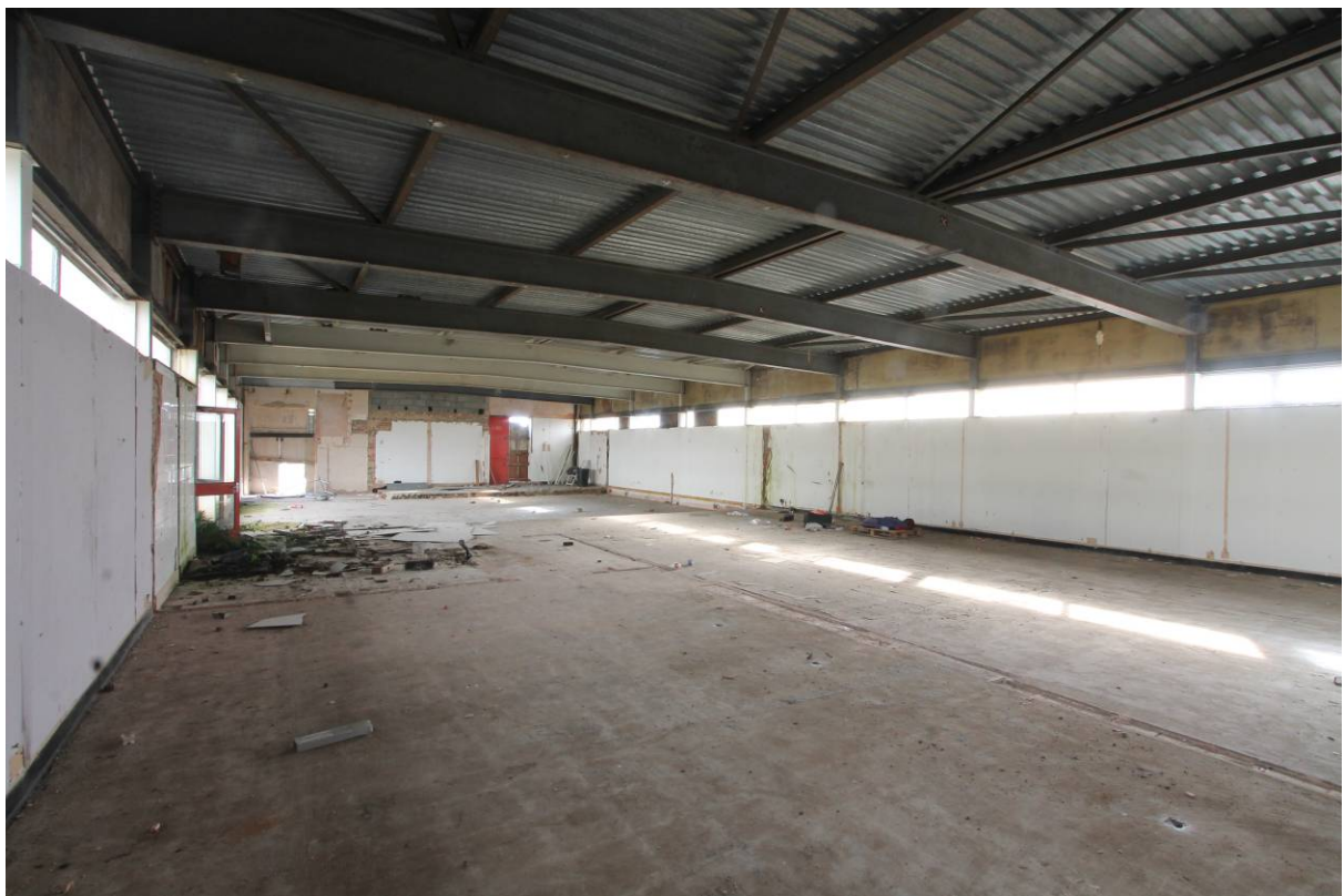
Plate 12 Internal view looking south-east
