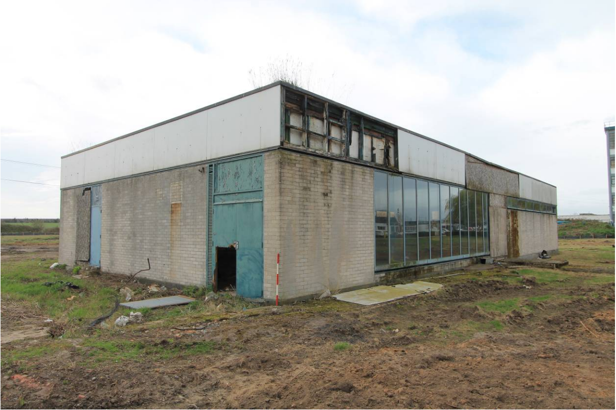
Plate 3 Computer Centre northern elevation, looking south-west
