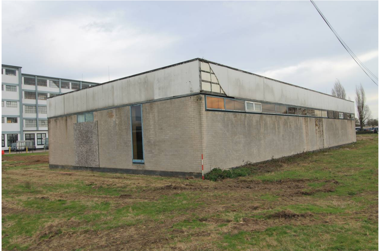
Plate 7 Computer Centre southern elevation, looking north-east
