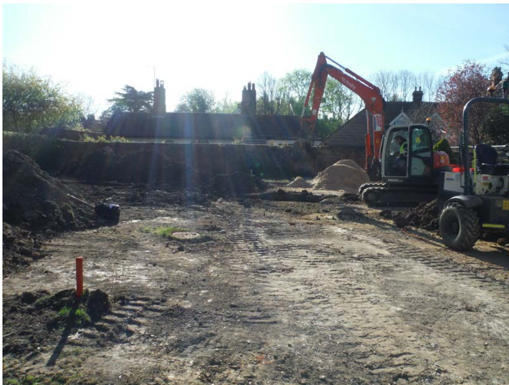
Plate 1: Site, view east
