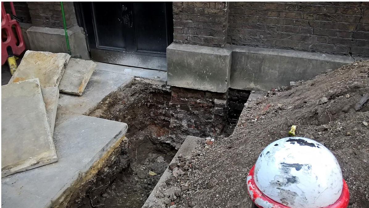
Plate 3: East facing section of wall foundation with central gate to south
