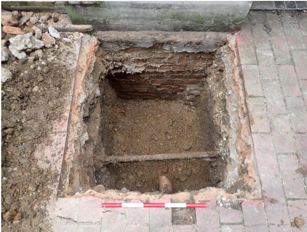
Plate 1: Looking south, Test Pit 1, northern wall of extension to Jackson's Corner truncating contexts [5], [9] and natural layer [10]
