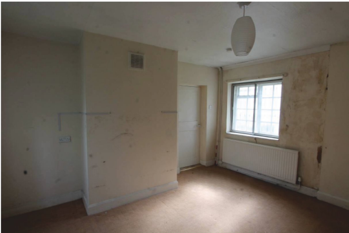
Plate 42 Unit 1 bedroom, showing inserted window (of 1961)
