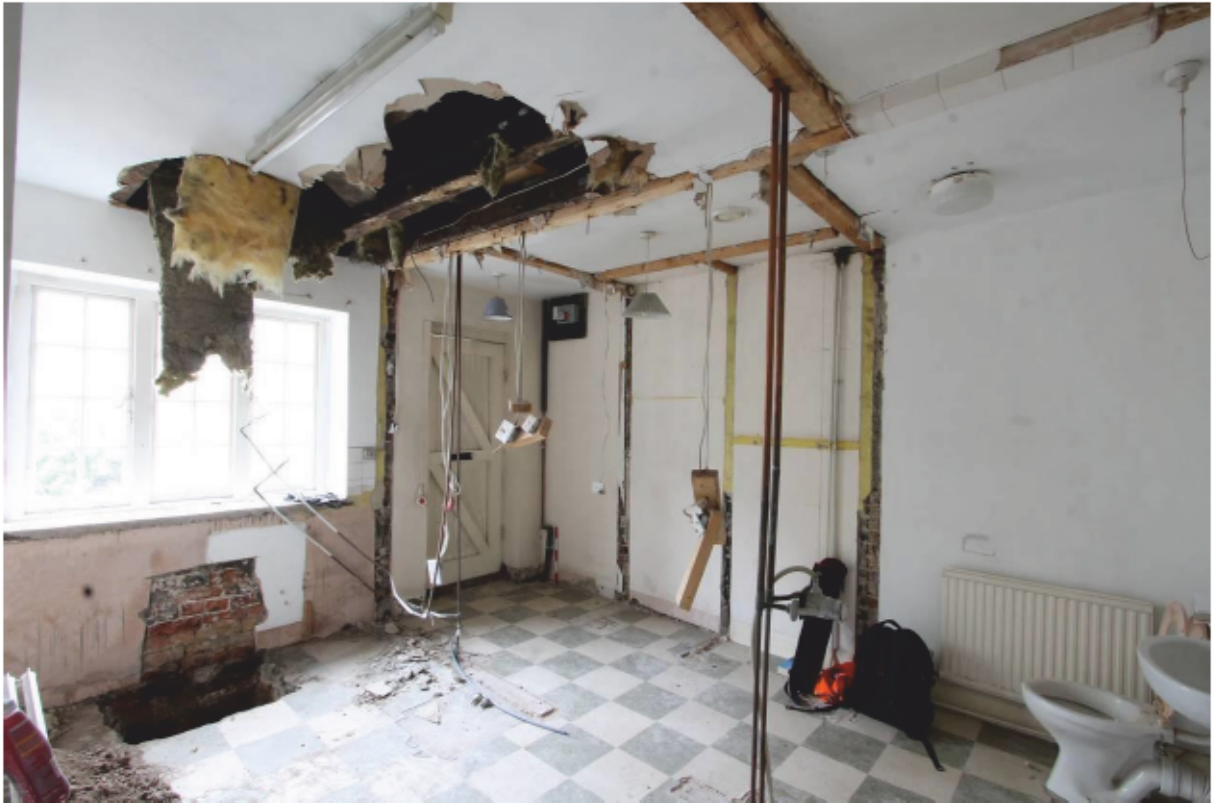
Plate 27 Unit 2, stripped out kitchen/shower/WC, looking north-west
