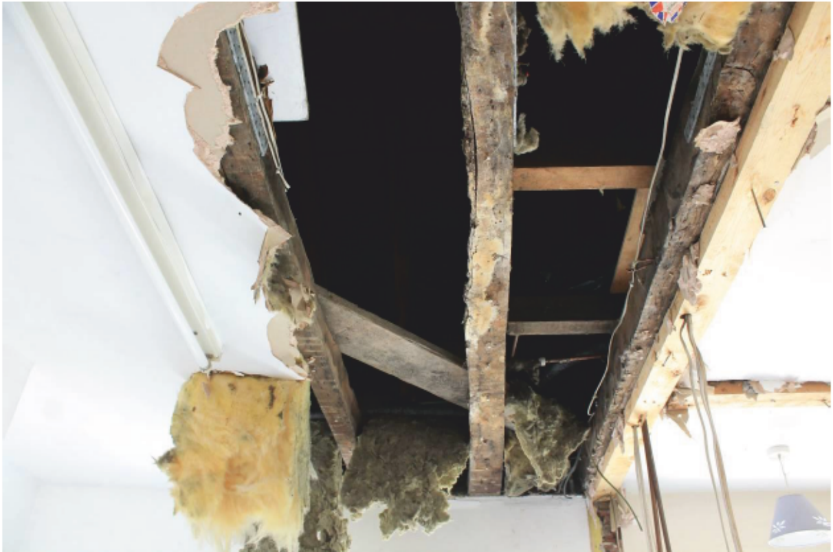
Plate 33 Common ceiling joists looking west
