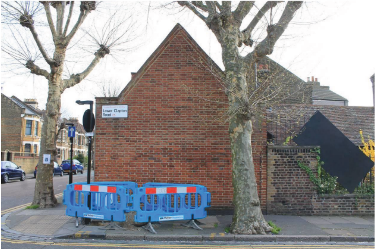
Plate 7 Rebuilt gable elevation of north range, looking east
