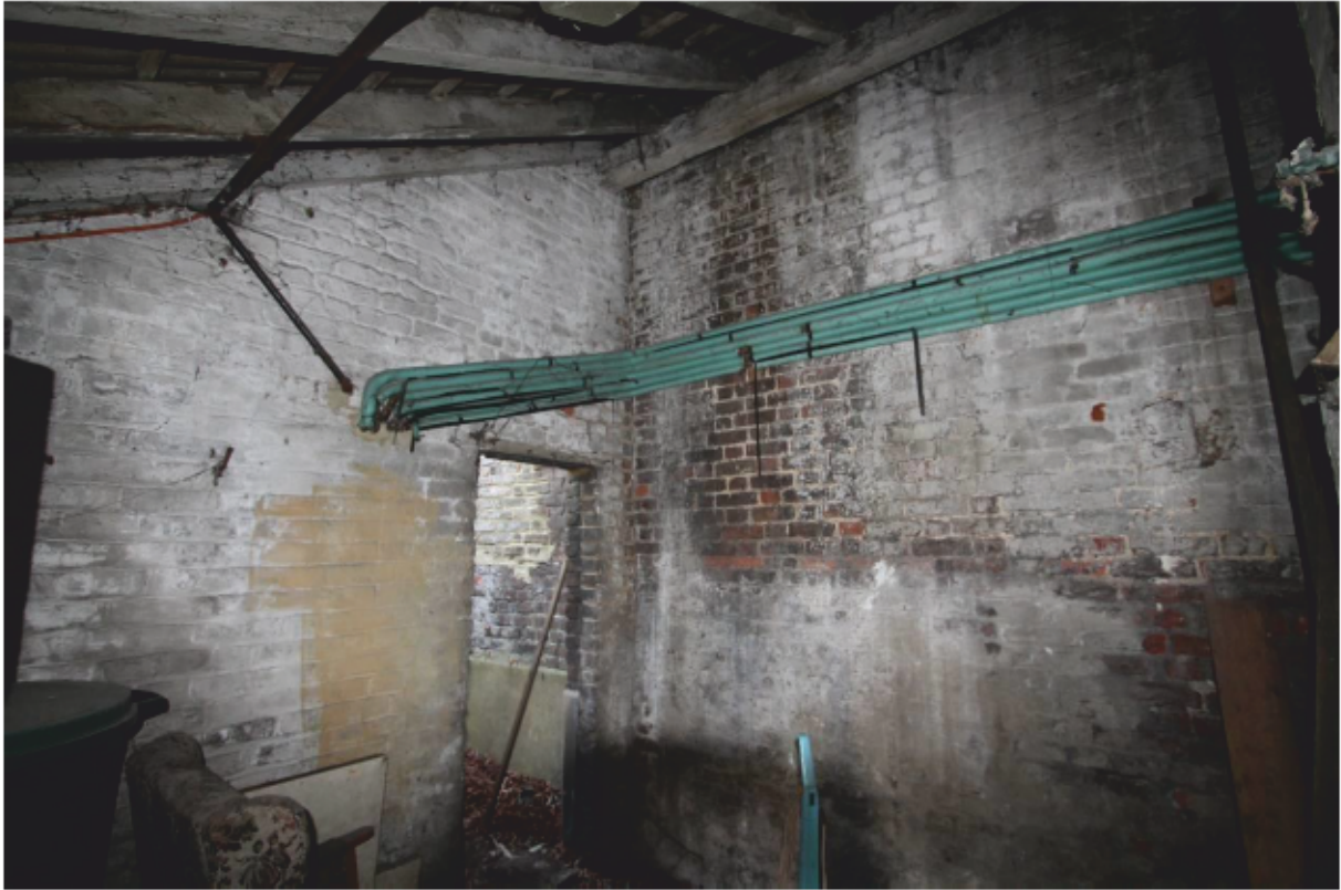
Plate 25 Former Scullery looking south-east
