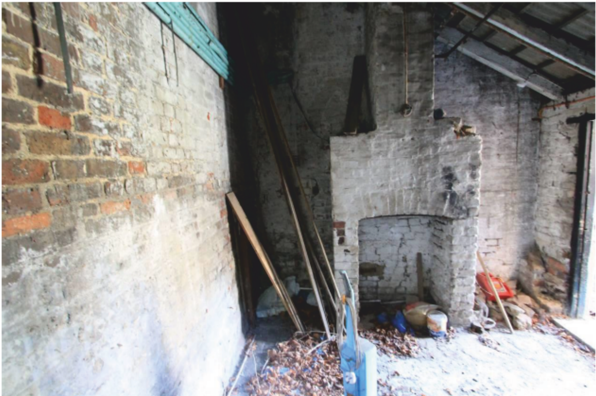
Plate 24 Former Scullery looking east
