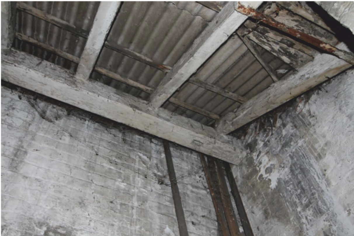
Plate 26 Lean-to roof structure, looking south-west
