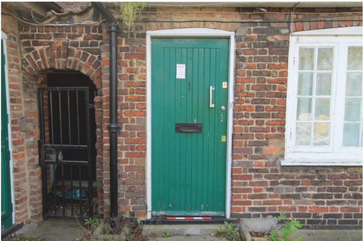
Plate 16 Typical main entrance door (Unit 1) and opening to former Scullery, looking south
