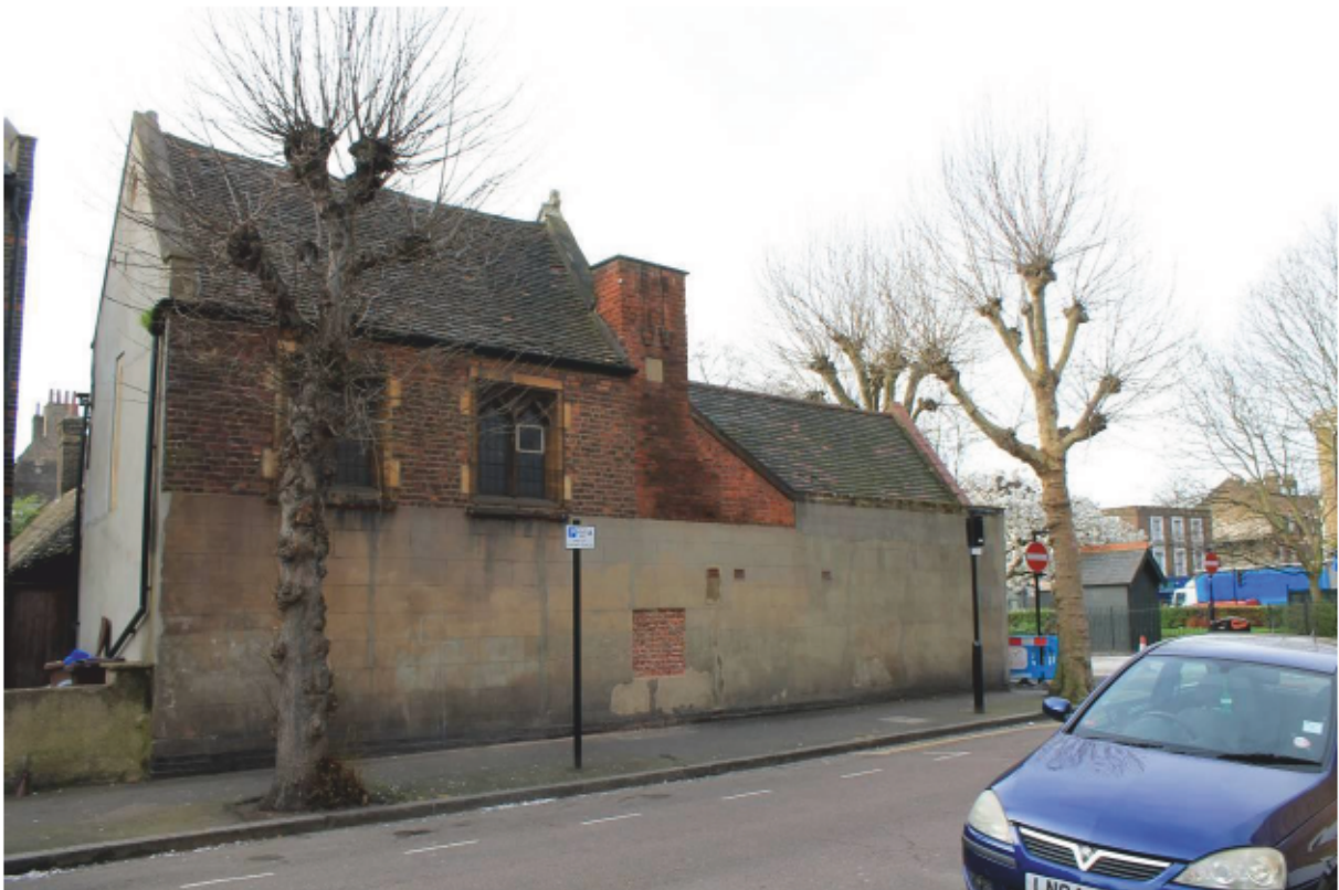
Plate 8 Northern elevation to Newick Road, looking south-west
