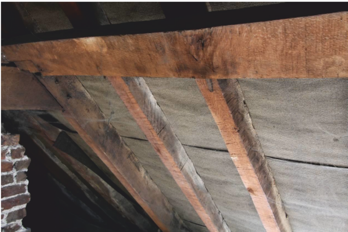
Plate 40 Oak rafters showing carpenters marks
