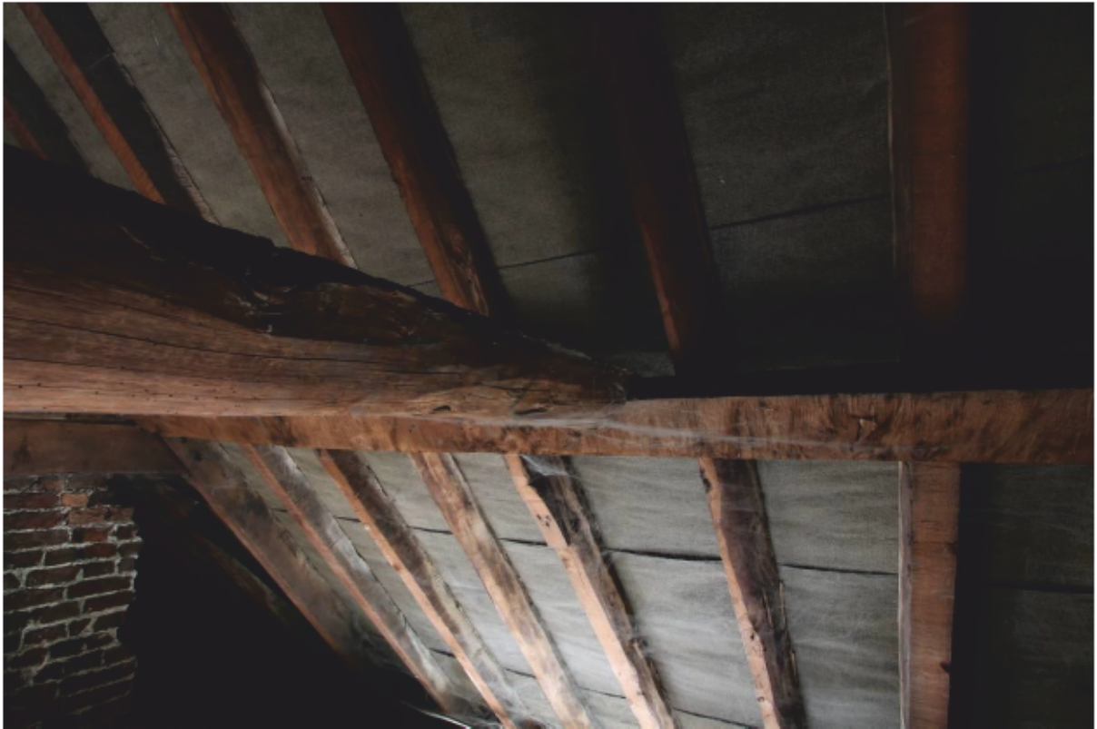
Plate 39 Intermediate collar and nailed-on cleat below purlin
