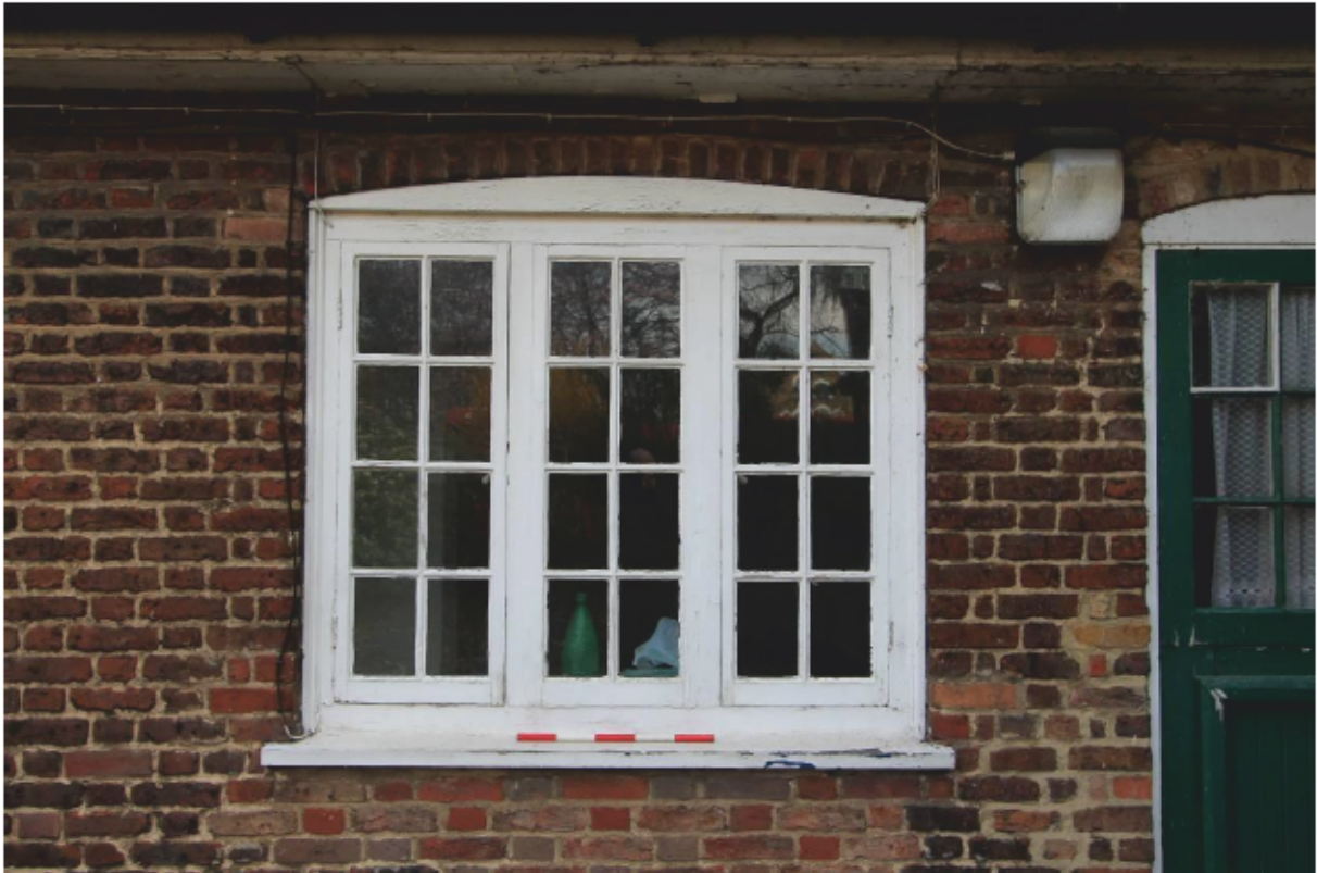
Plate 15 Typical mullioned casement window
