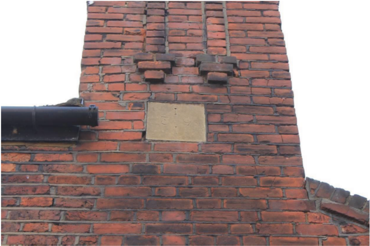
Plate 9 Date plaque of 1918 set into rebuilt stack
