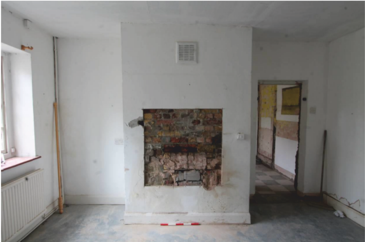
Plate 29 Central boxed in fireplace, looking north
