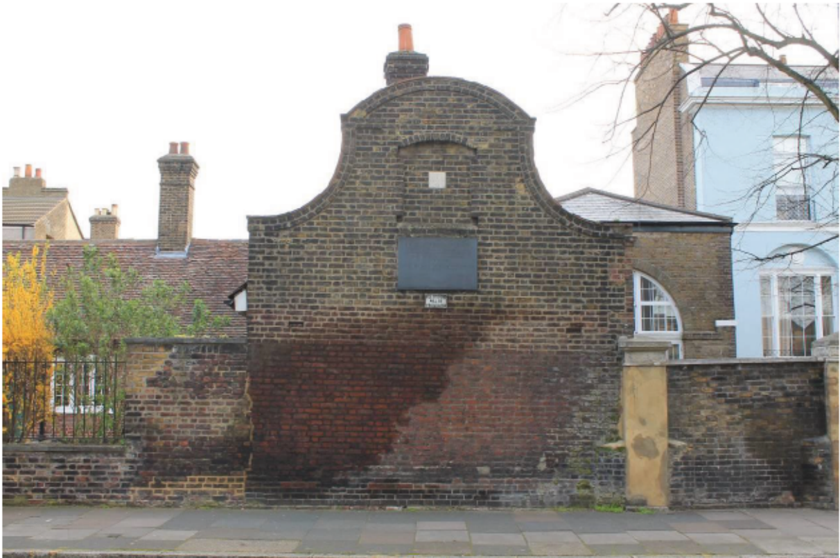
Plate 11 Rebuilt shaped gable elevation to south range, looking east
