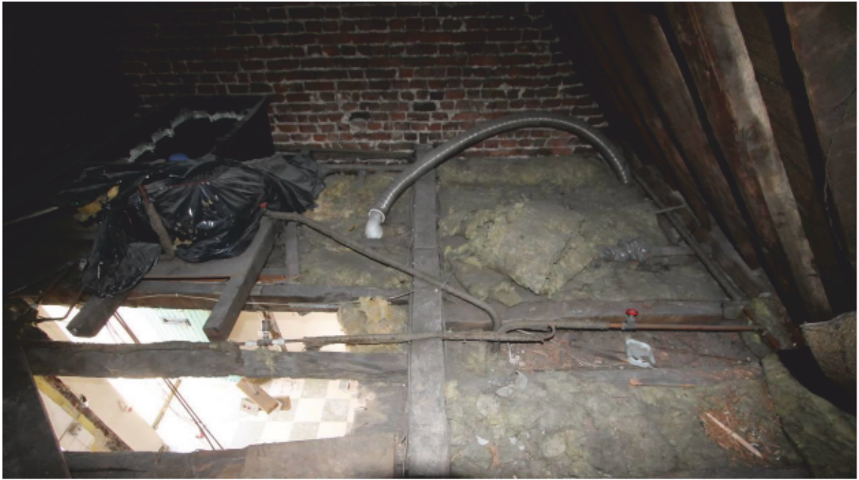
Plate 35 Axial bridging beam and common joists (unit 2)
