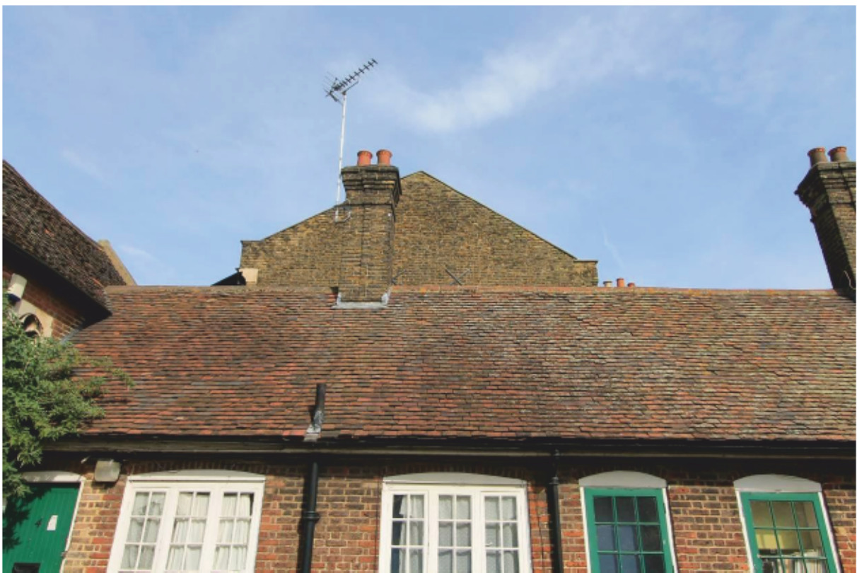
Plate 14 Plain tile roof over Unit 4, looking east
