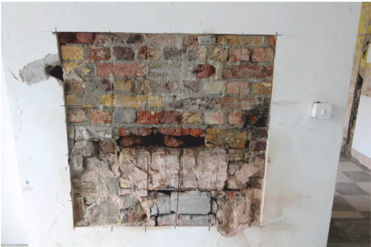
Plate 30 Detail of rebuilt fireplace and later blocked in opening
