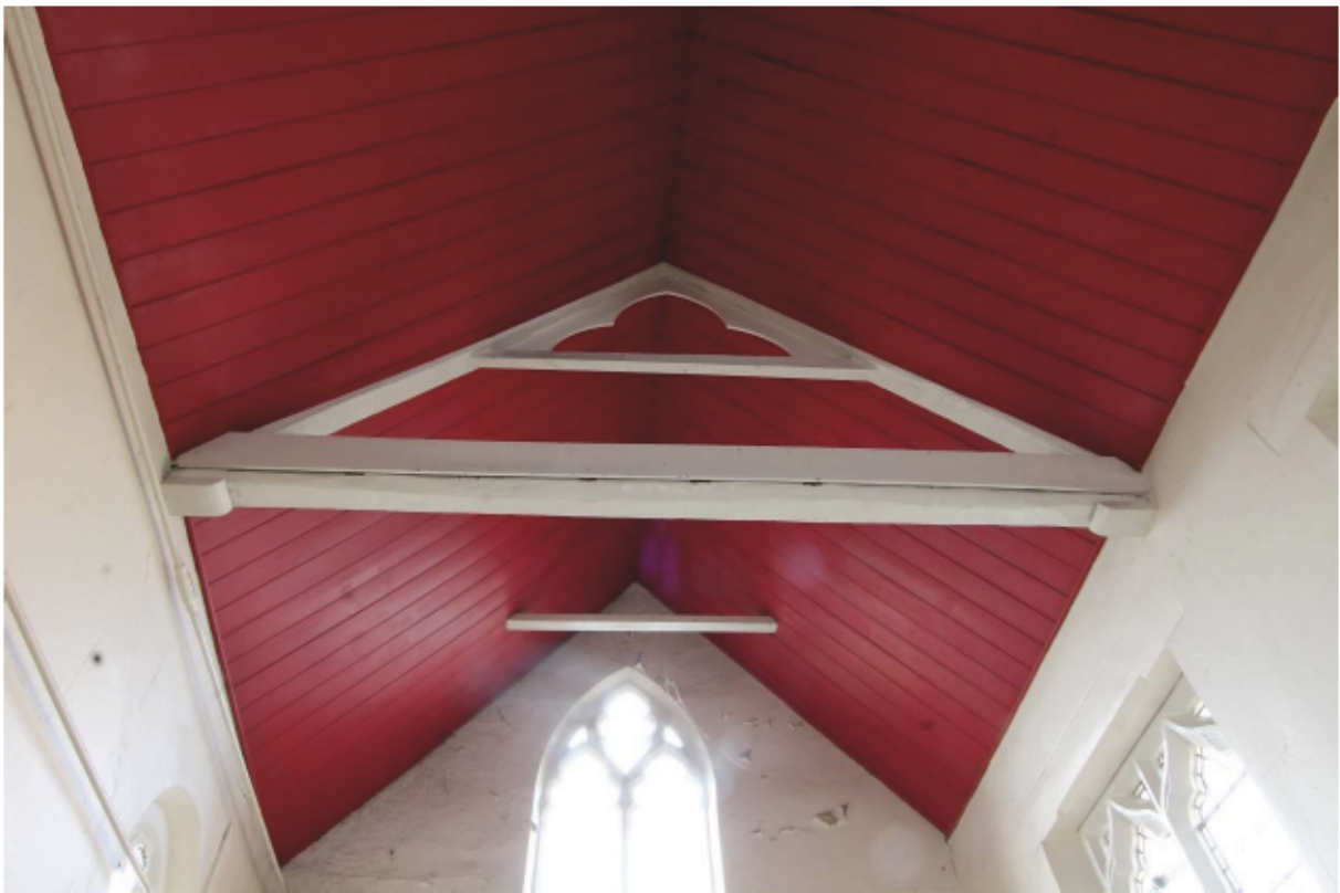
Plate 20 Chapel; Central roof truss, looking west
