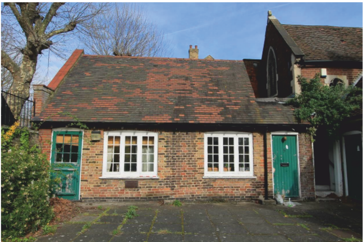
Plate 4 View to re-roofed northern range, looking north
