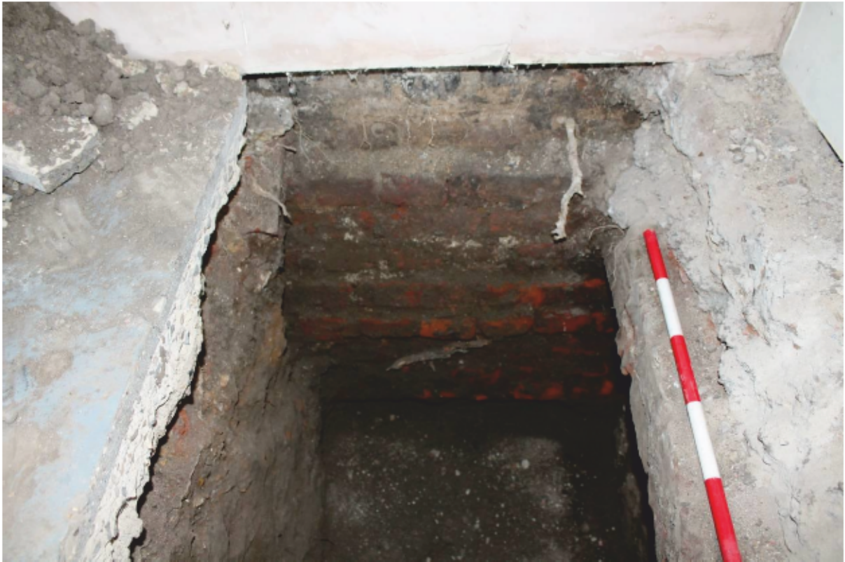
Plate 31 Brick Foundation to rear eastern wall
