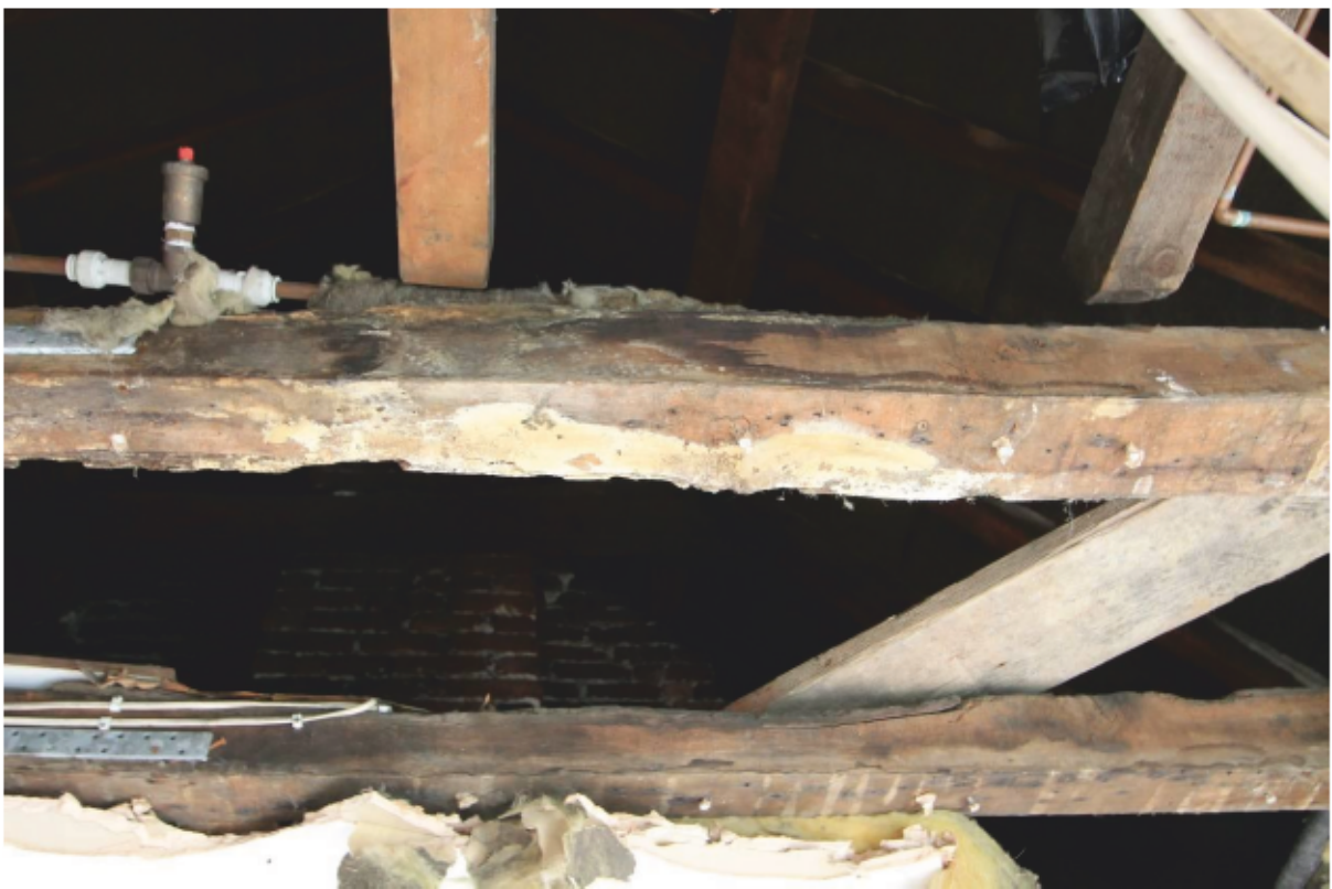
Plate 34 Detail of 17 th century rough sawn common ceiling joists looking south
