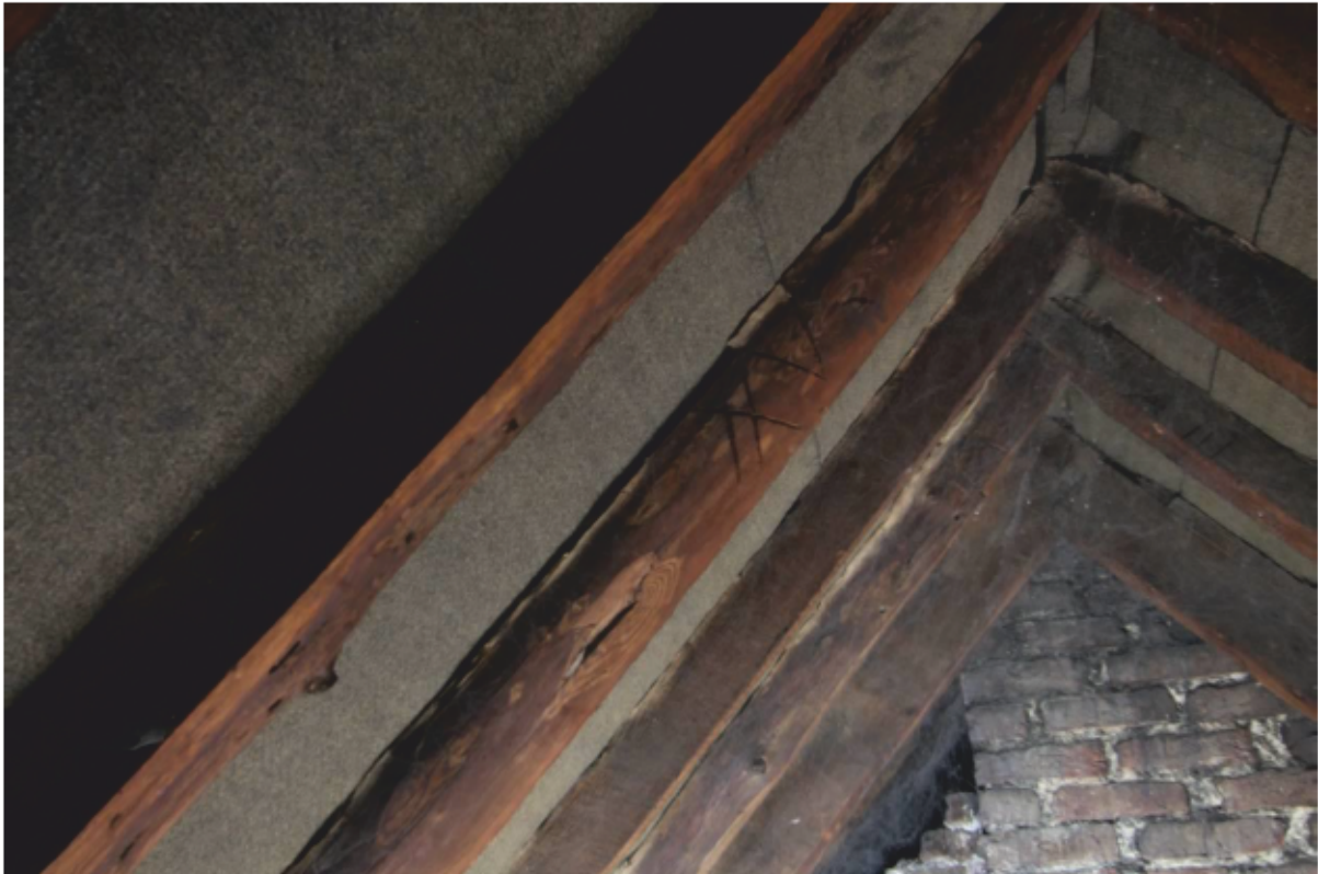
Plate 41 Mixture of hard and softwood rafters, pegged at ridge
