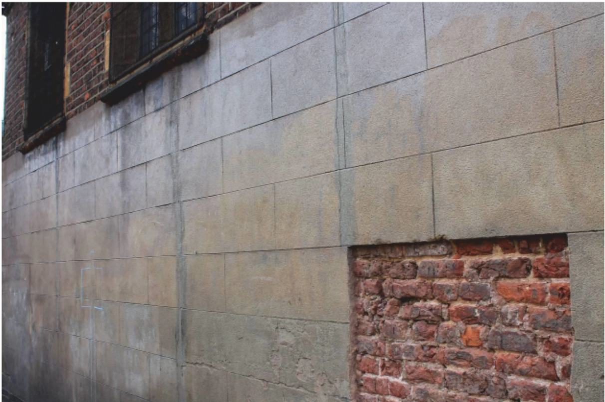
Plate 10 Hard cement 'Ashlar' render to lower wall.
