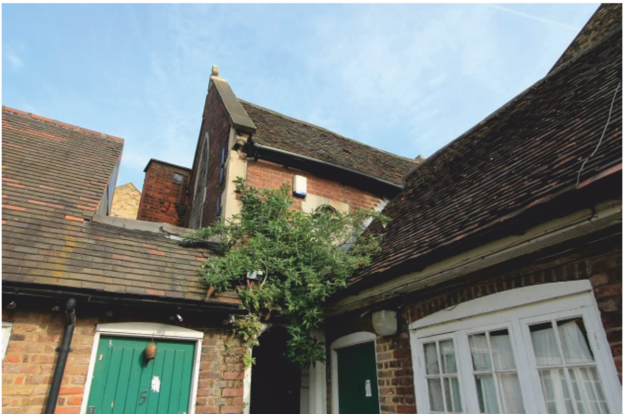
Plate 18 Arched entrance to Chapel, looking north
