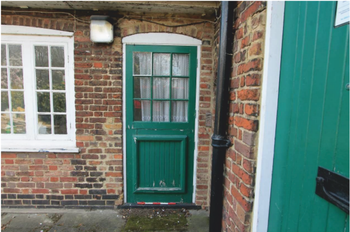
Plate 17 Typical 'heck-type' door to bedrooms (Unit 2) looking east
