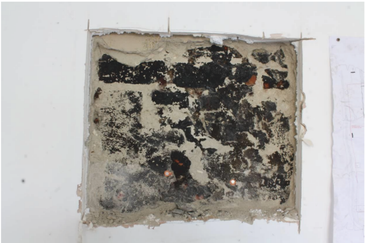
Plate 32 Bituminous paint covering to interior walls
