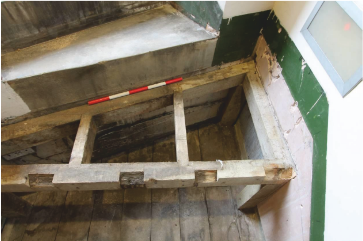
Plate 9 Detail of sub-structure
