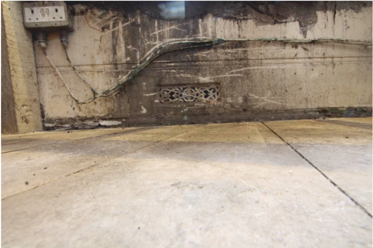
Plate 11 Plaster skirting and cast-iron ventilator
