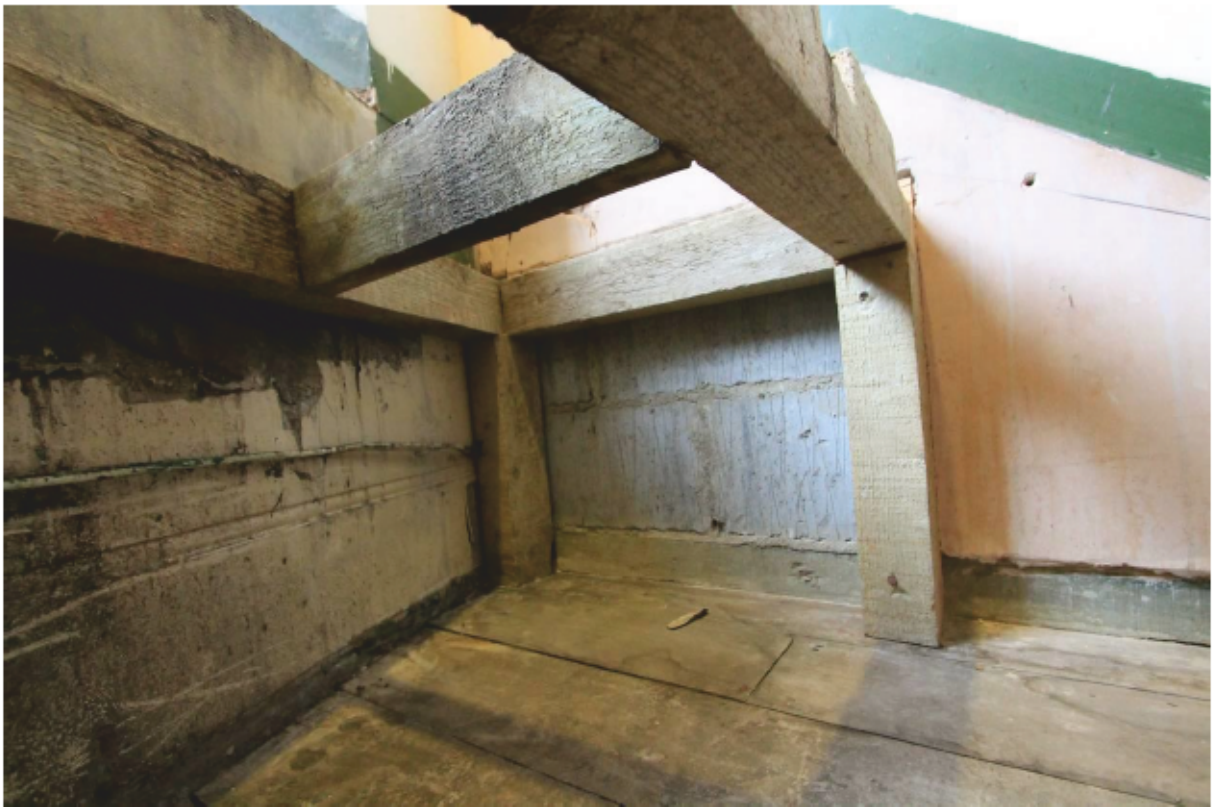
Plate 10 Detail of posts and modern blockwork in adjacent wall
