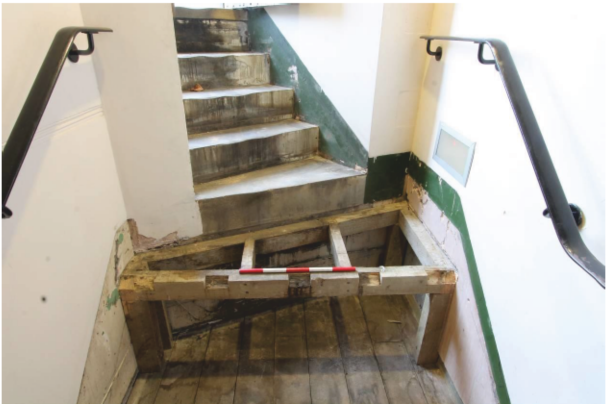
Plate 8 Sub-structure to modern stair
