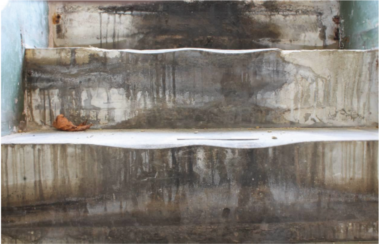
Plate 7 Wear to treads
