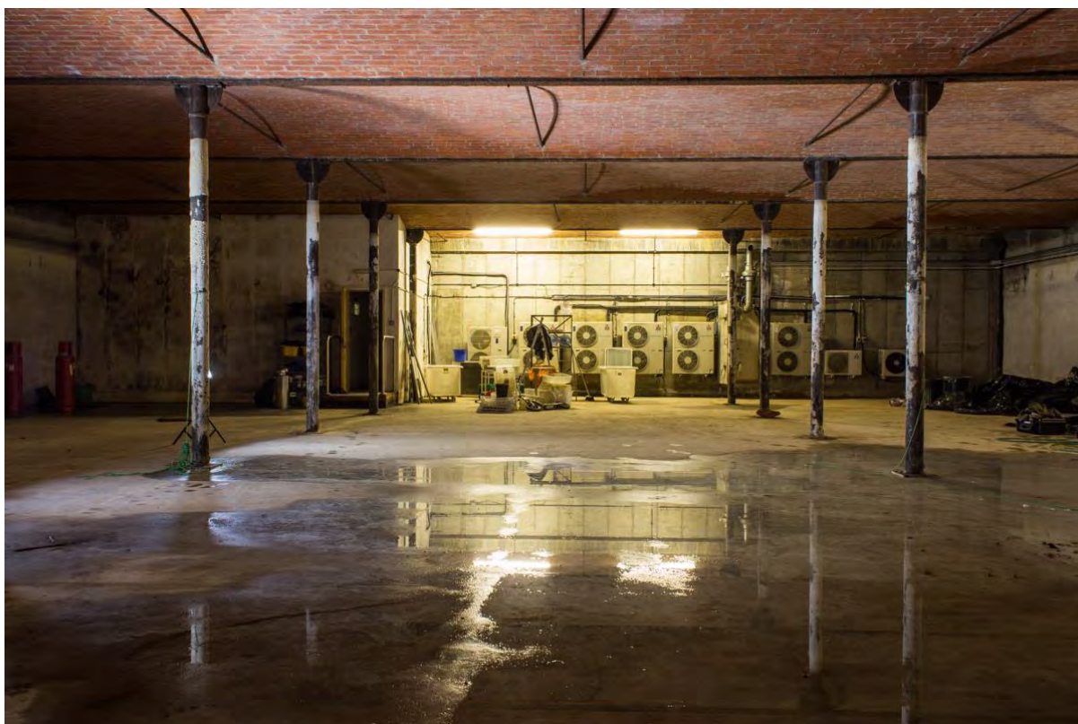
Plate 10 South-west facing internal elevation
