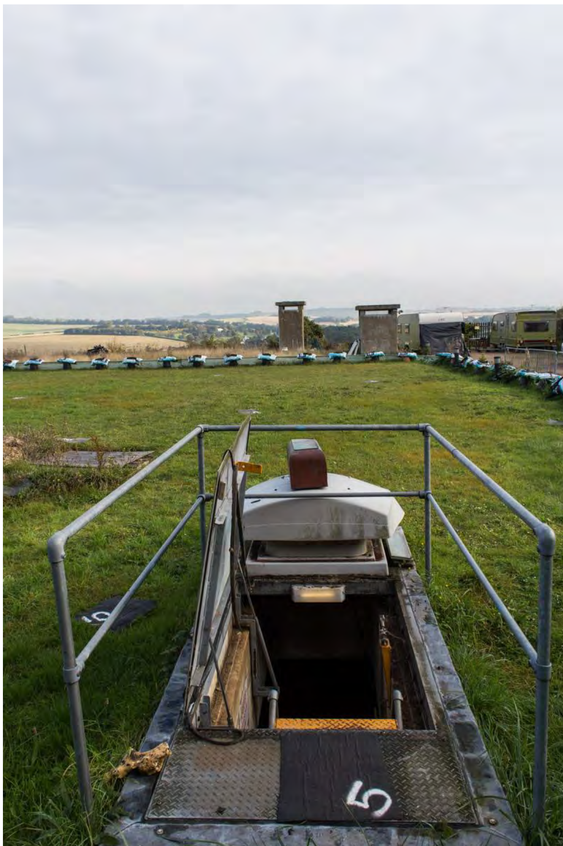
Plate 3 View to the north-east of escape hatch (foreground) and bunker ventilation shafts (background)
