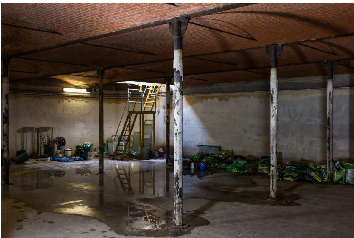
Plate 13 View to the south of reservoir interior - showing supporting steel columns
