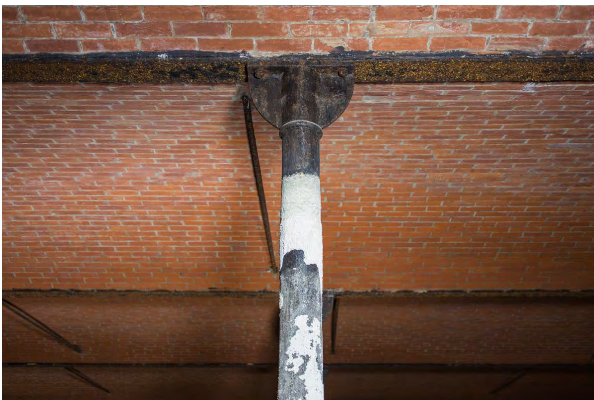
Plate 16 Example of supporting column and beam
