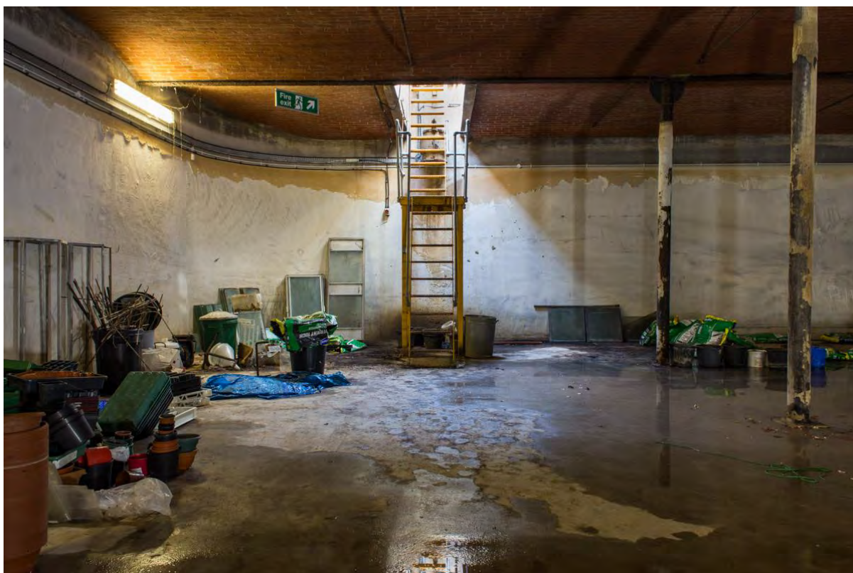
Plate 12 View to the south-west of escape hatch steps
