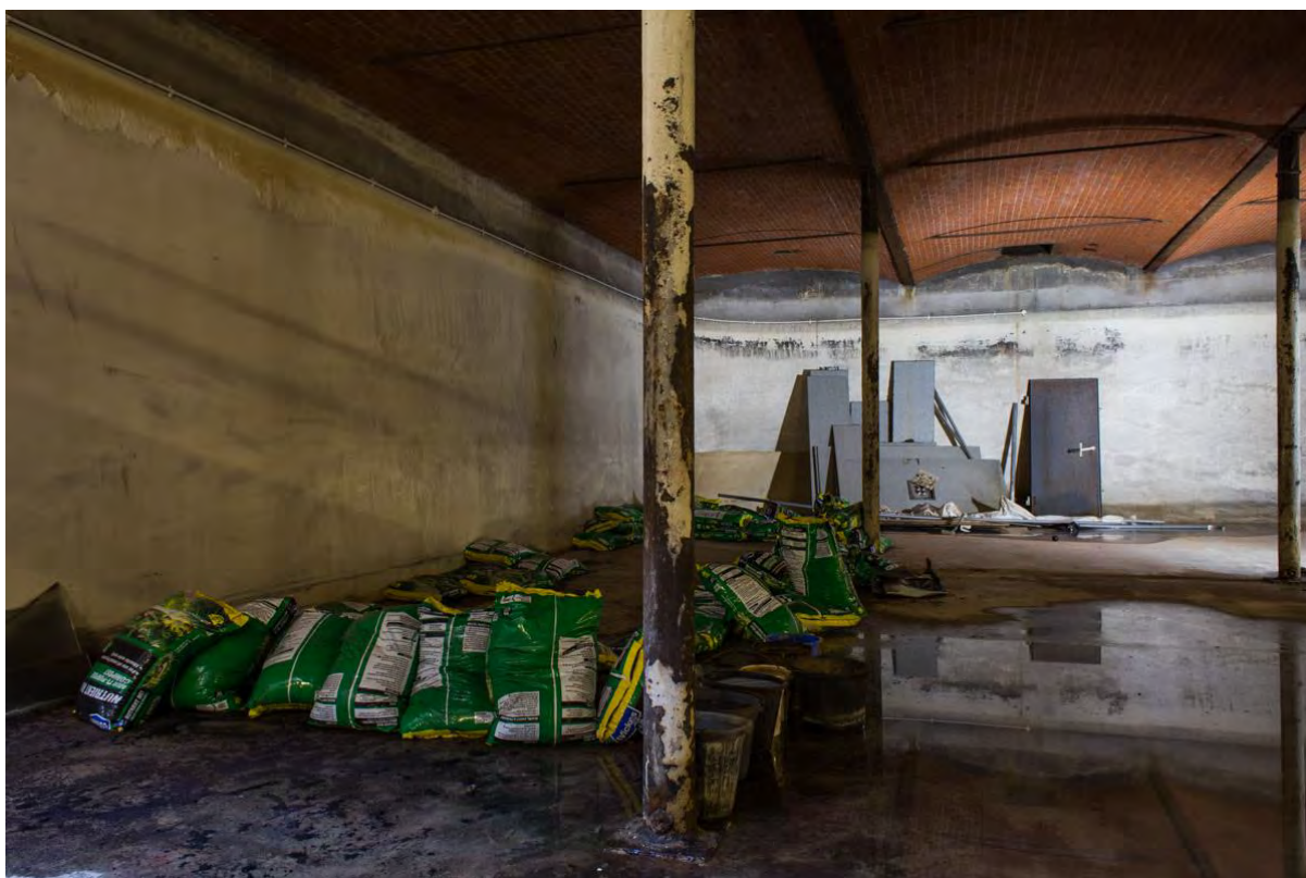
Plate 5 View to north-west from reservoir entrance
