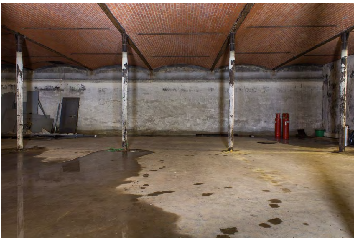
Plate 11 South-east facing internal elevation
