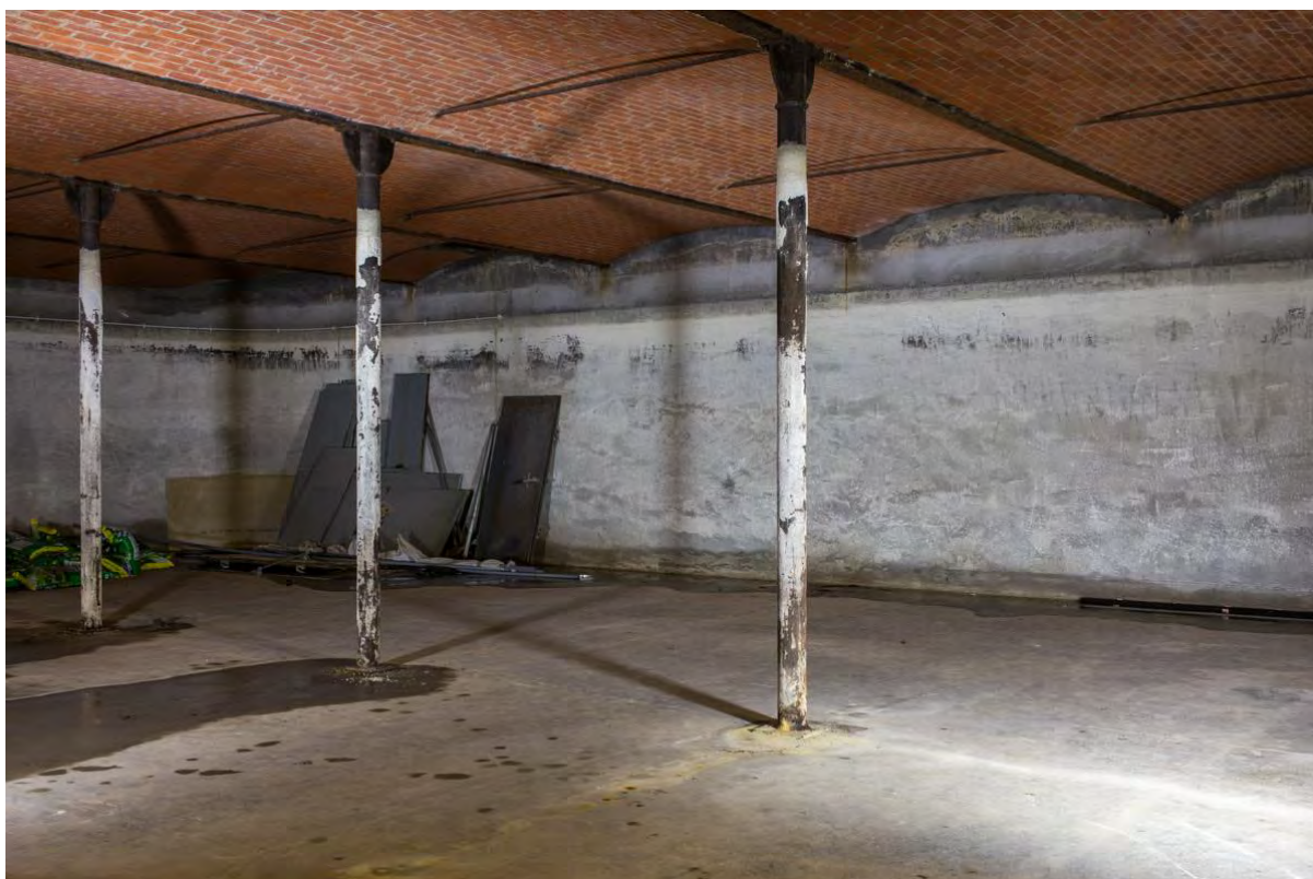
Plate 14 View to the west of reservoir interior - showing supporting steel columns and barrel vaulting
